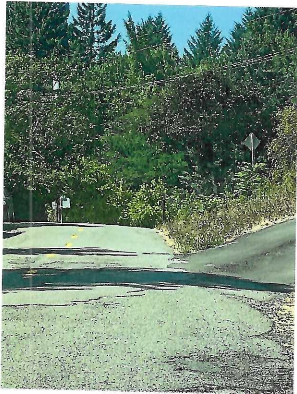
PHOTO 2 – Mile 0.0 Church Street intersection with Alderpoint
