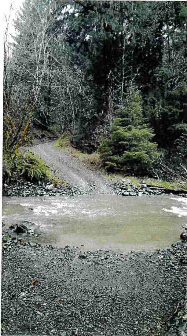
Picture 6: This is a photograph of the existing rock ford crossing downstream of the project area. Turbidity can be seen in the photo from recent vehicle traffic. The completion of the bridge installation will negate the use of this crossing. Photo date: 04/07/2017
