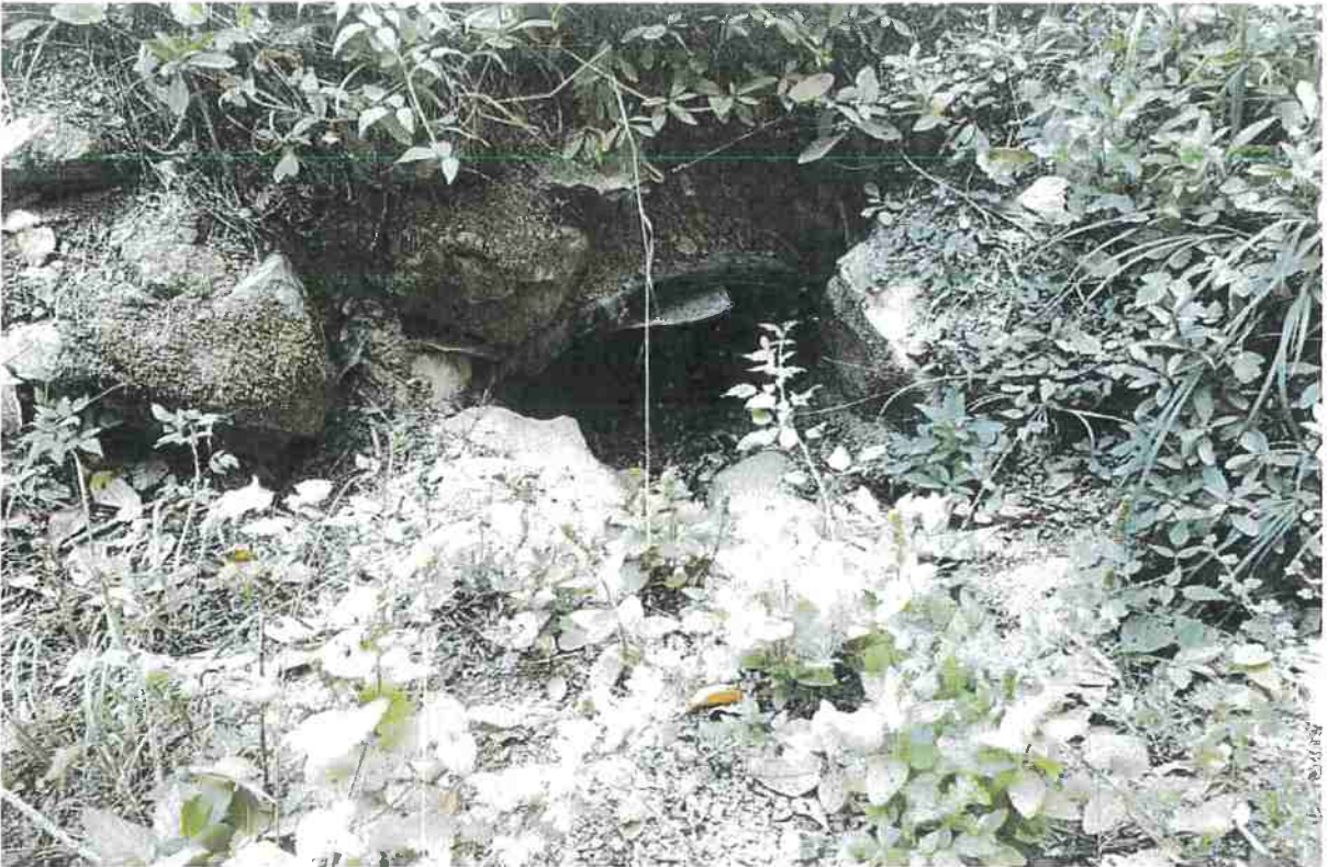
Photo looking at the inlet of the culvert at Site 07.
