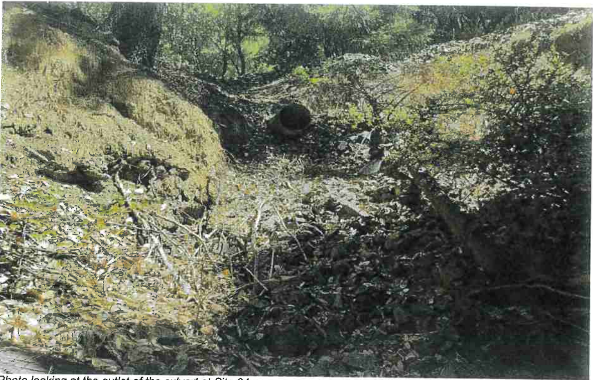
Photo looking at the outlet of the culvert at Site 04.
