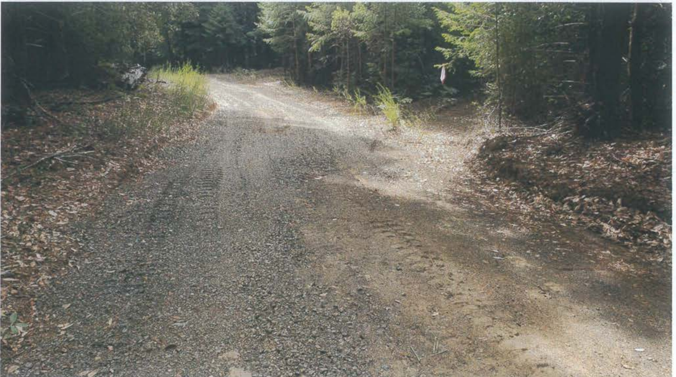
Photo looking down grade at rocked rolling dip installed at Site 12.
