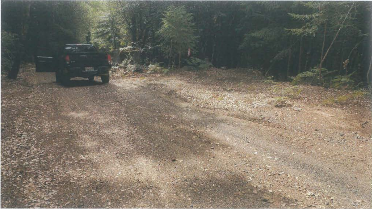
Photo looking down grade at a rocked rolling dip installed at Site 13.
