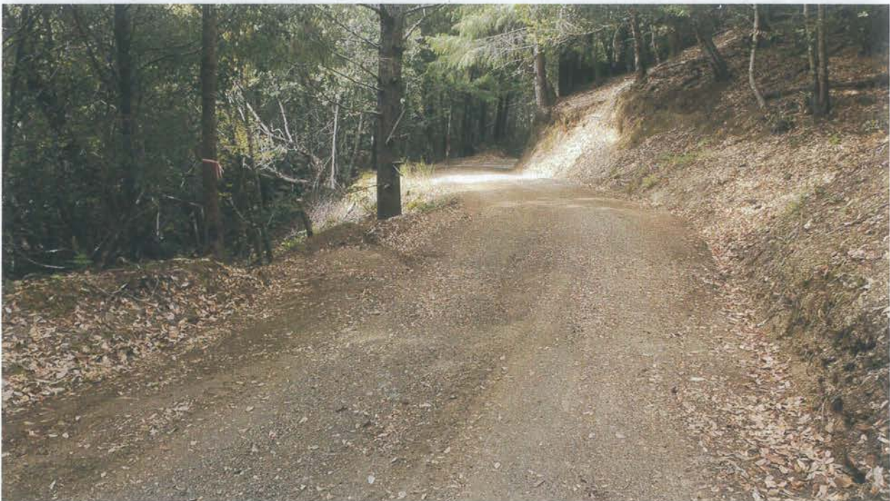
Photo looking down grade at a rocked rolling dip installed at Site 03.
