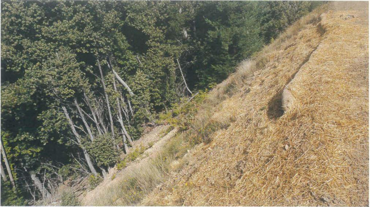
Photo looking at another fillslope that was treated at Site 08.
