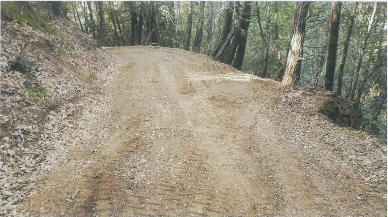
Photo looking down grade at a waterbar installed at Site 15.
