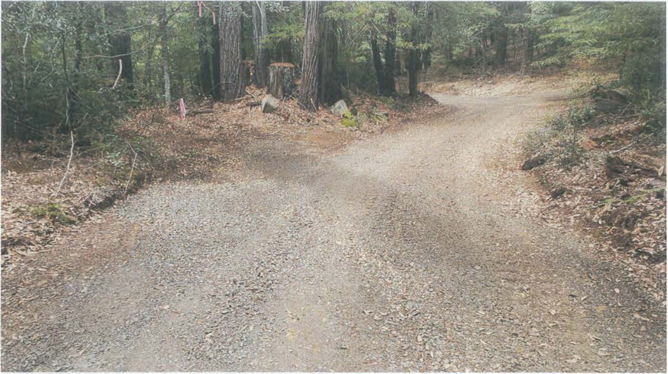
Photo looking down grade at a rocked rolling dip installed at Site 09.
