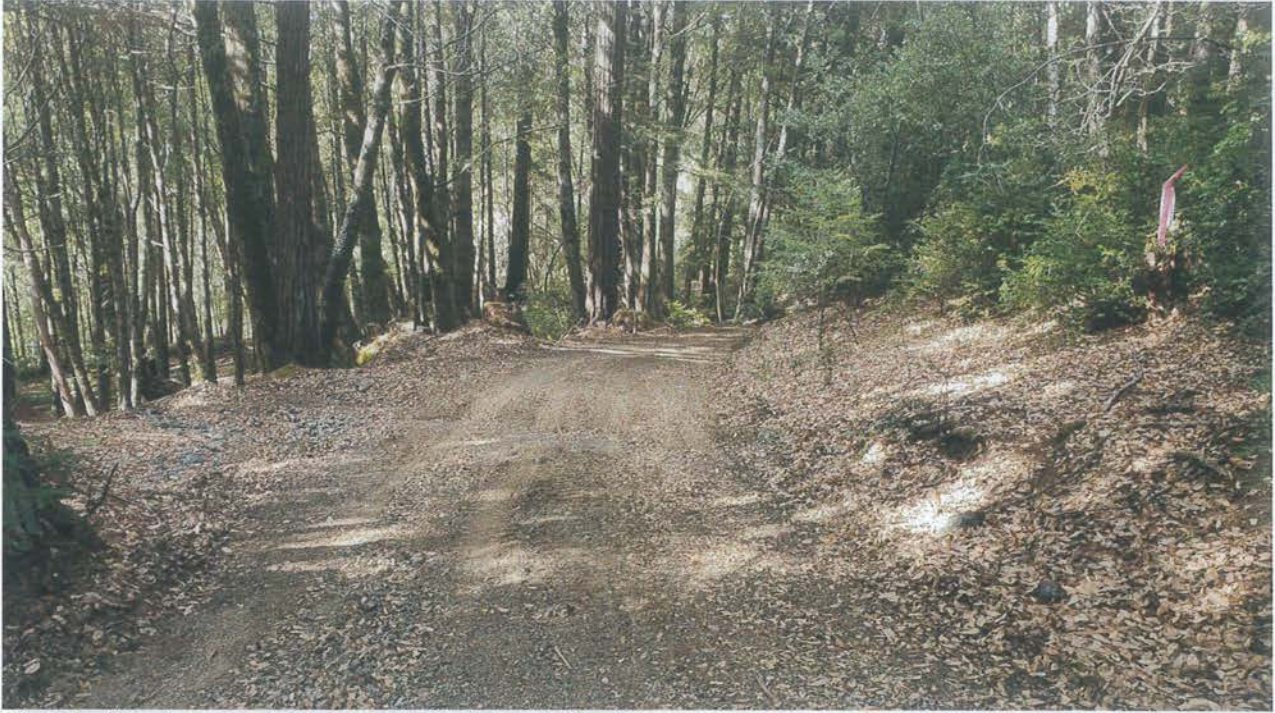
Photo looking down grade at a waterbar installed at Site 07.
