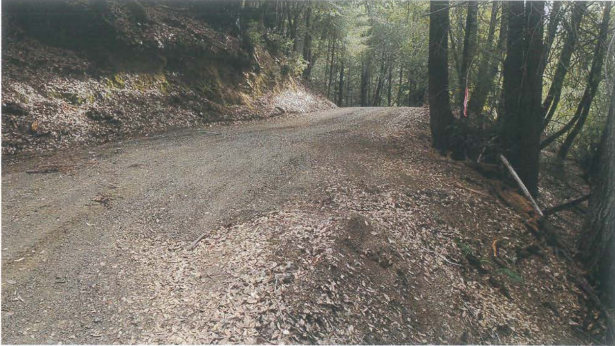
Photo of another rolling dip/kickout that was installed a short distance up grade of Site 03.
