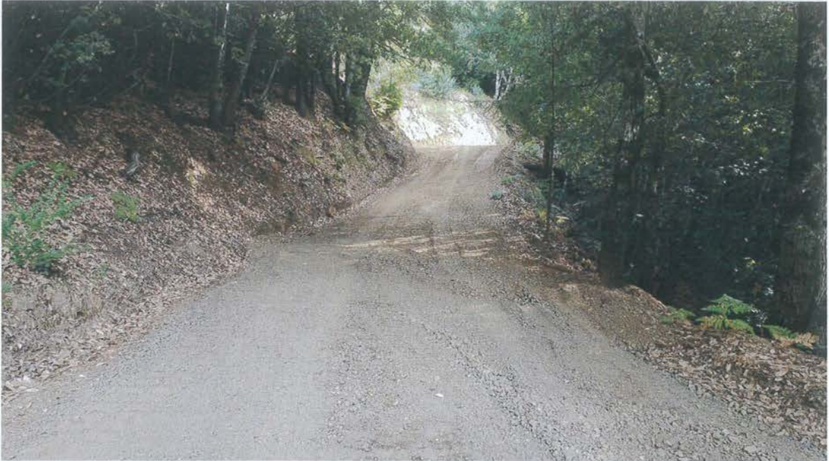
Photo looking up grade at Site 01. A rocked rolling dip was in the process of being installed here and additional road rock surfacing was being brought in to finish the prescribed treatment at this location.
