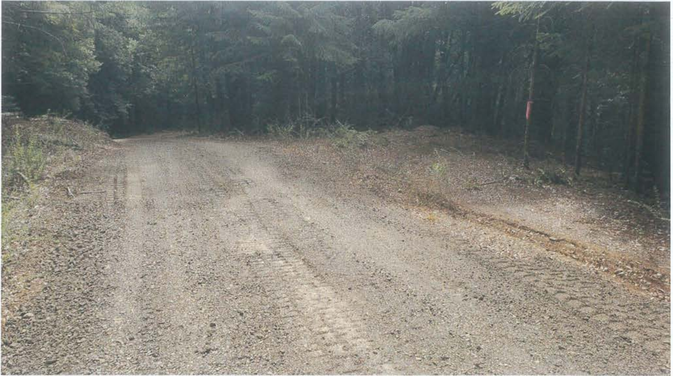
Photo looking down grade at a rocked rolling dip installed at Site 11.
