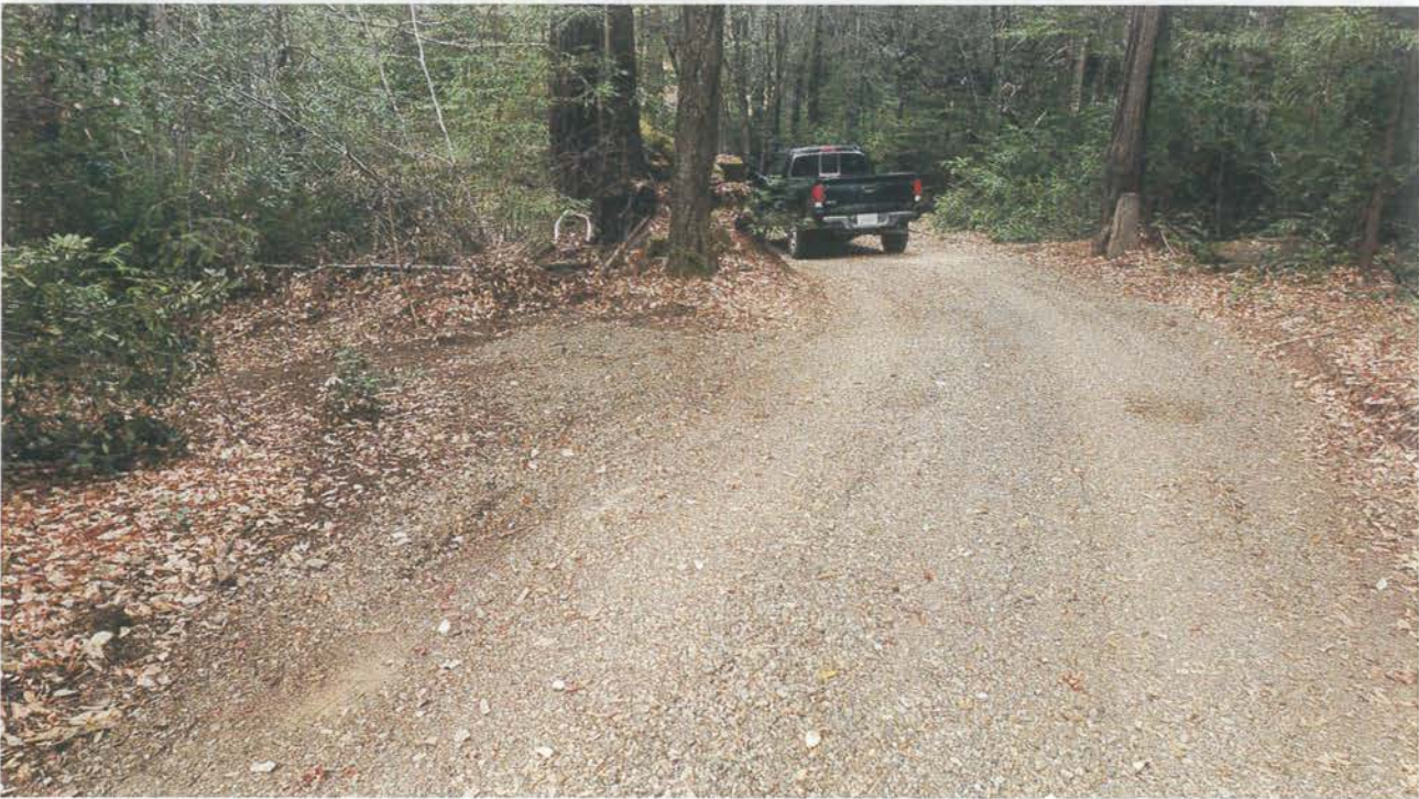
Photo looking down grade at a kick out/outsloping drainage feature up grade of Site 09.
