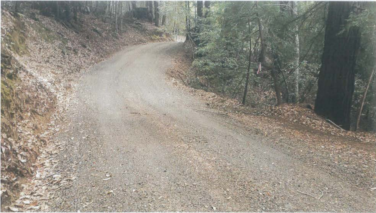
Photo looking up grade at Site 05.
