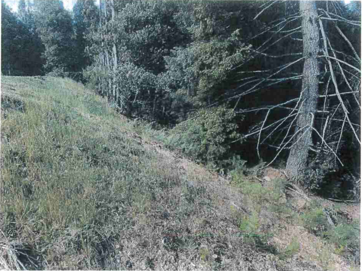
Picture 7. Site 3's fill-slope where no erosion occurred from poor drainage. Photo date 5-20-2021.
