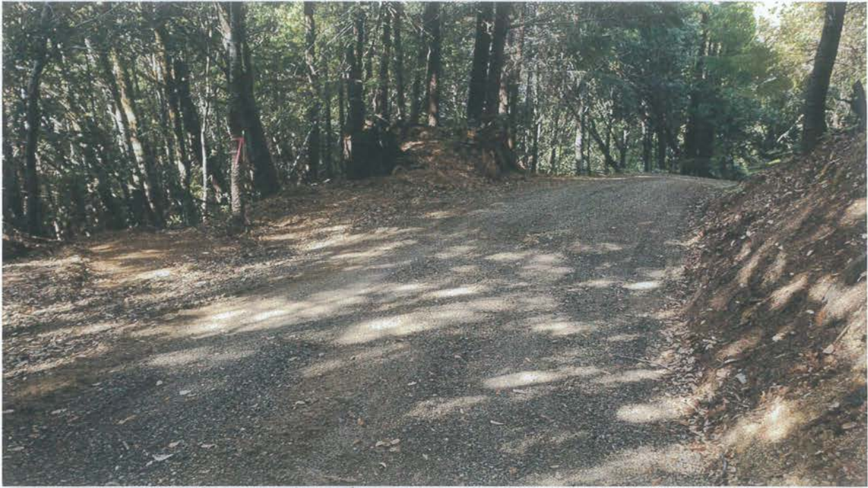
Photo looking down grade at a rocked rolling dip at Site 02.
