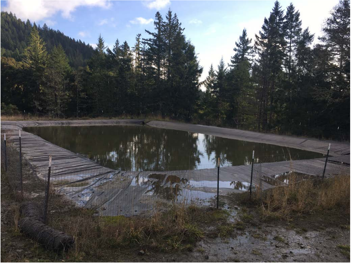
Rainwater catchment pond point of collection.
