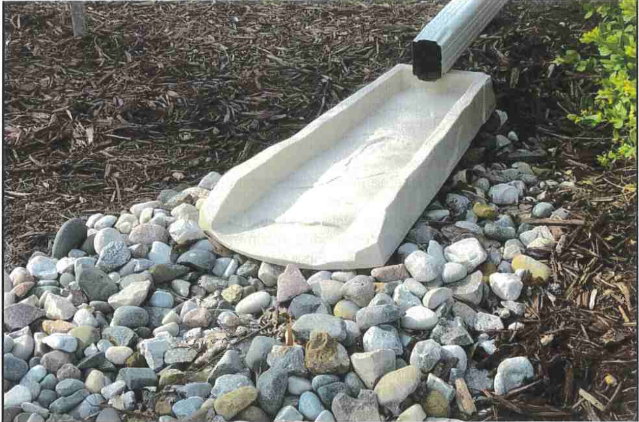
Figure 2: Rain gutter Splash Way/Energy Dissipator
