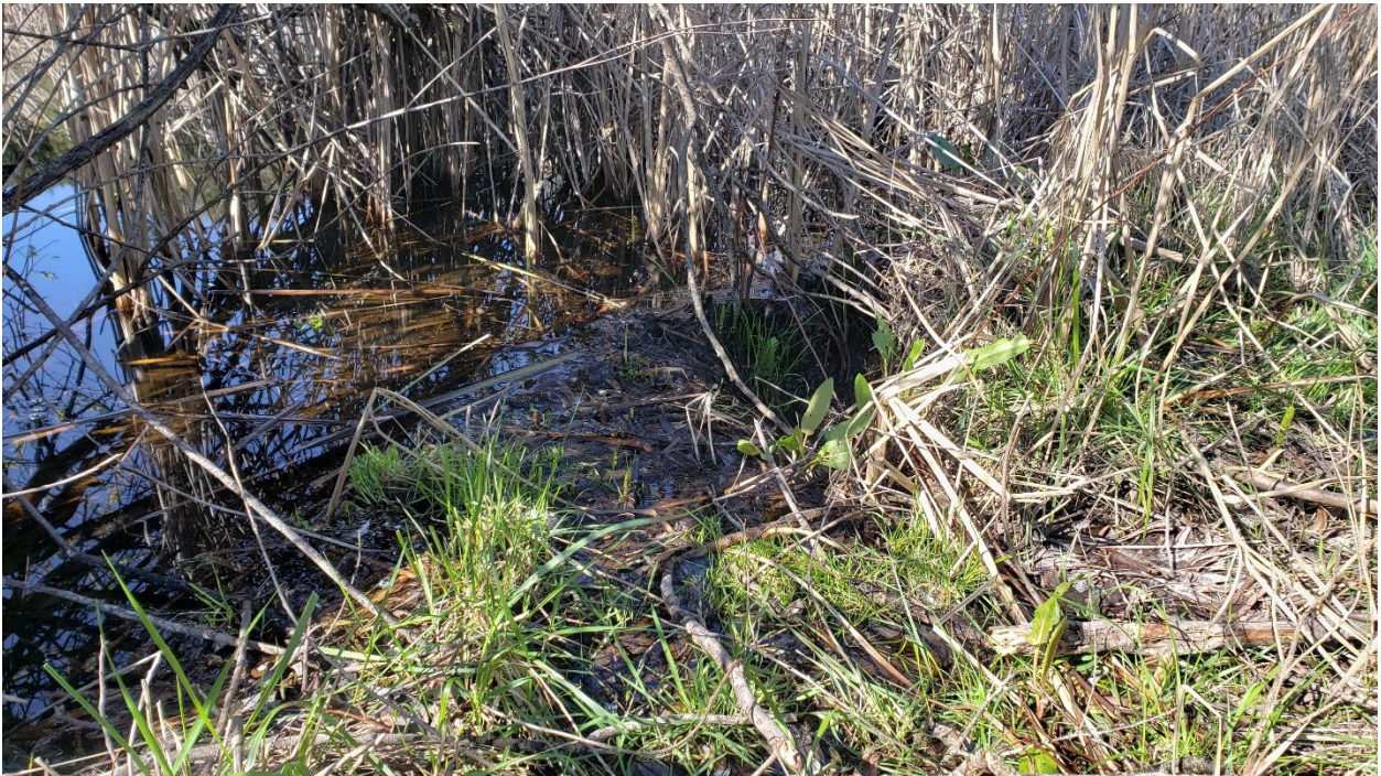
Photo looking northwest at the inlet of the impoundment overflow structure inlet at WQ-9. March 2 nd , 2021
