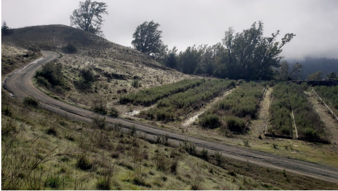
Photo looking southeast at the easternmost edge of WQ-1 grading area from PM 1. March 2 nd , 2021
