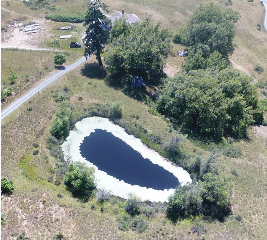
Aerial photo looking down at WQ-8. June 4 th , 2020
