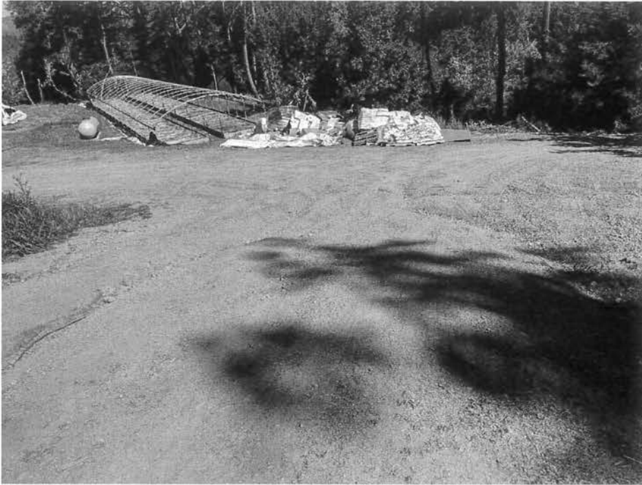
Site 19: Moderate riling occurring from concentrated surface runoff.
