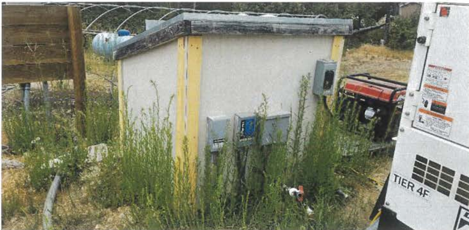
Groundwater well located on the south portion of the property.
