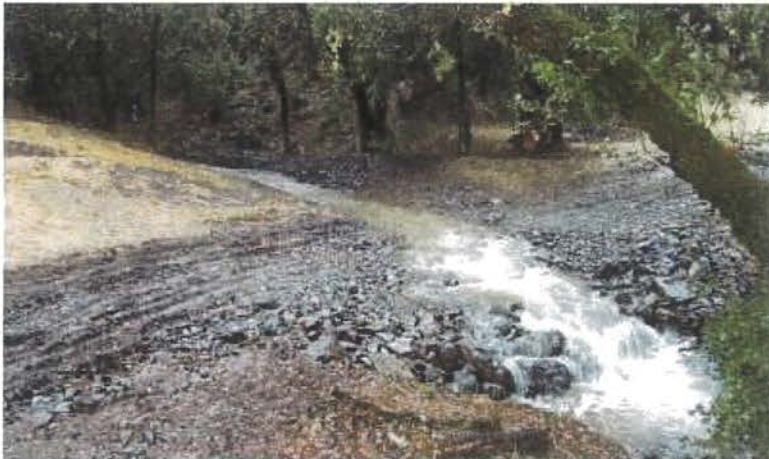
FIGURE 121E. Two weeks after this armored fill was constructed, a storm flow event occurred and the structure maintained its function and integrity. The road approaches had not yet been compacted or surfaced with road rock.
