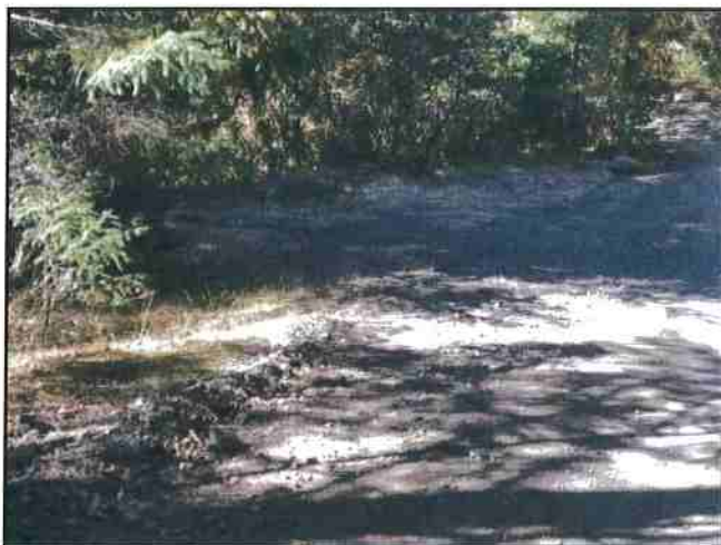
Photo #149 River Rd Looking NW @ Curve w/ Turnout
