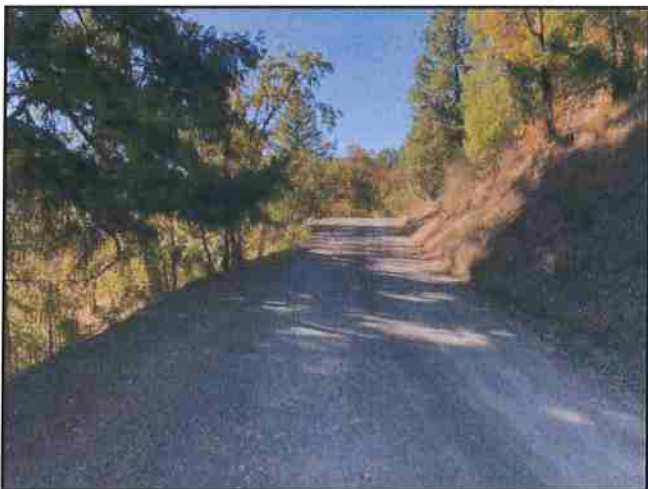
Photo #59 River Rd Looking NW @ Curve w/ Turnout
