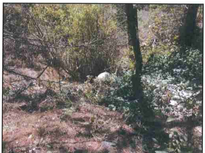
Photo #138 River Rd Looking @ 36" Culvert Out
