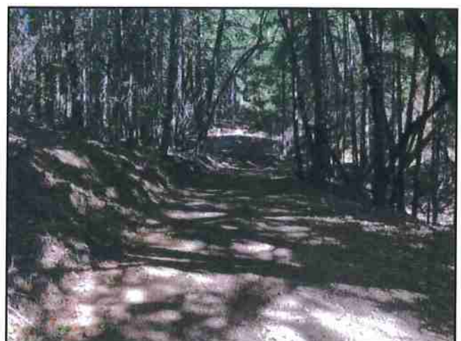
Photo #611 Mad River Trail @ Turnout Location Looking NE @ Curve
