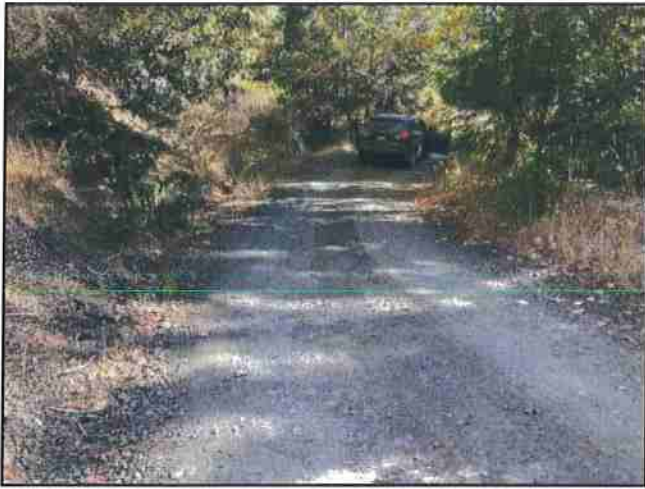
Photo #373 River Rd @ Turnout Location Looking NE @ Curve
