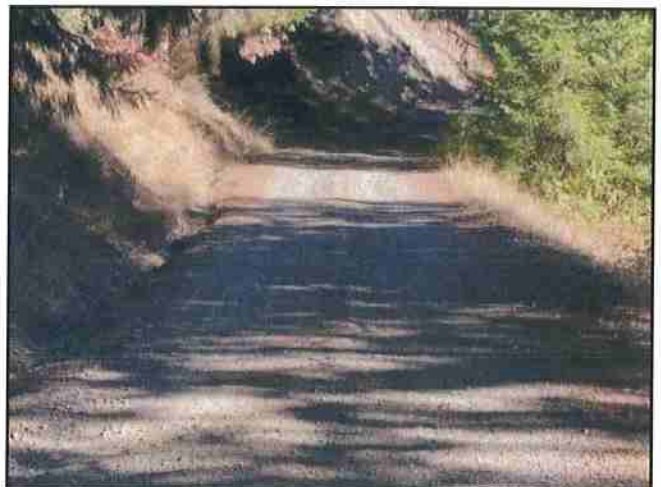
Photo #340 River Rd @ Turnout Location Looking SE @ Curve
