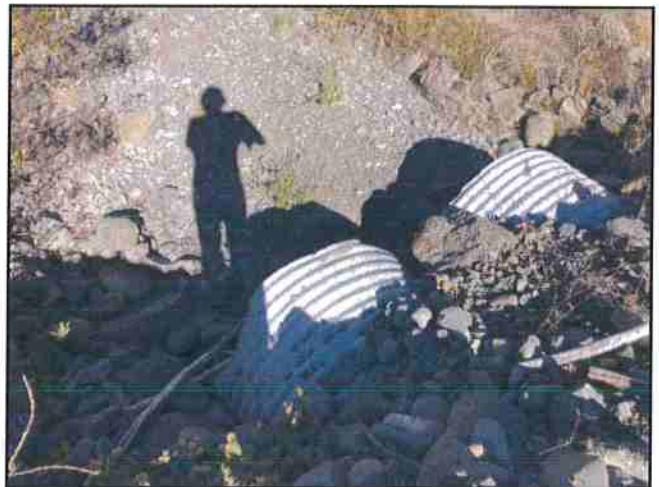
Photo #16 River Rd Looking @ Dual 36" Culverts Out
