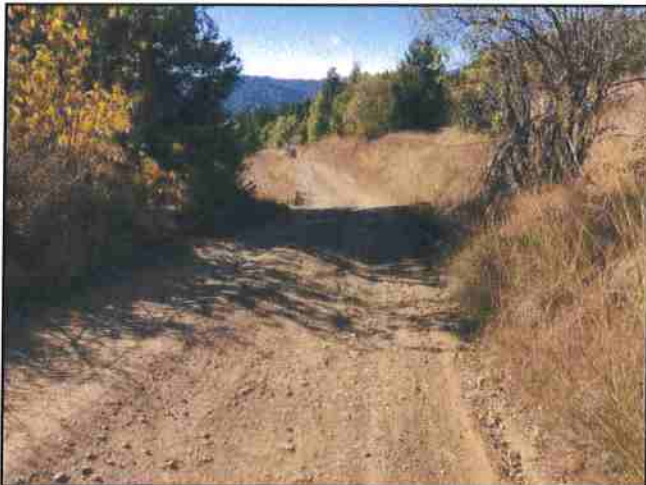
Photo #417 River Rd @ Curve w/o Turnout Looking West
