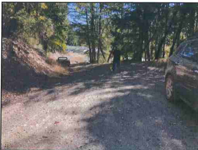
Photo #110 Private Access Rd APN 208-221-014 @ Cultivation / Turnout Area Looking SE
