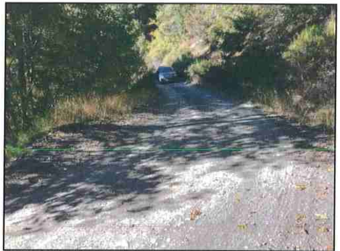
Photo #356 River Rd @ Turnout Location Looking NE @ Curve
