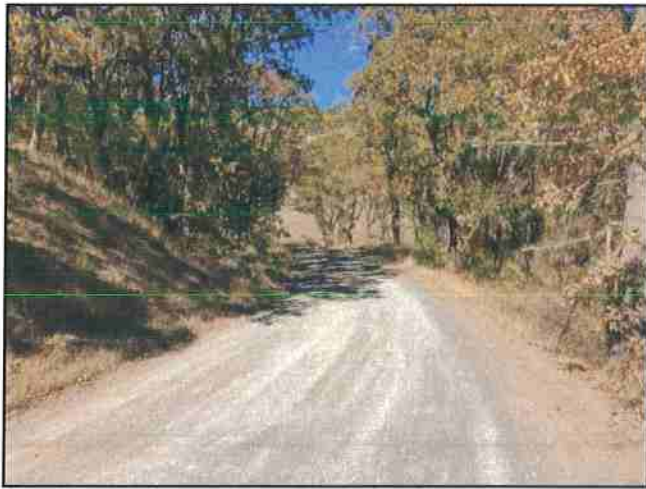
Photo #73 River Rd @ Turnout Looking North @ Curve
