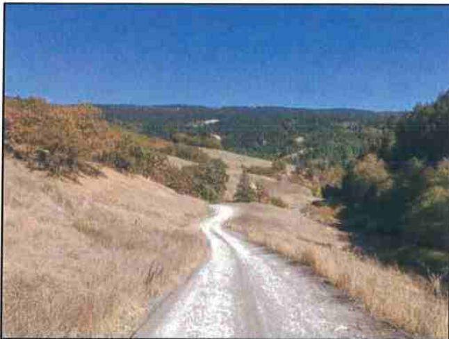
Photo #45 River Rd Looking East @ Curve w/ Pullout
