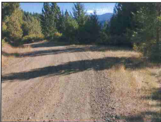
Photo #371 River Rd @ Turnout Location Looking SE @ Curve
