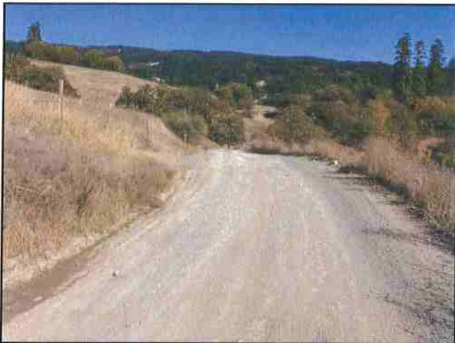
Photo #39 River Rd Looking East @ Curve w/ Pullout
