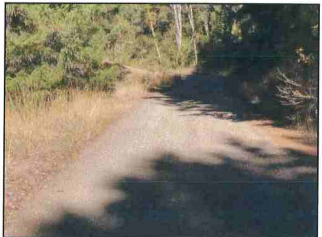
Photo #292 River Rd Looking South @ Curve w/ Turnout
