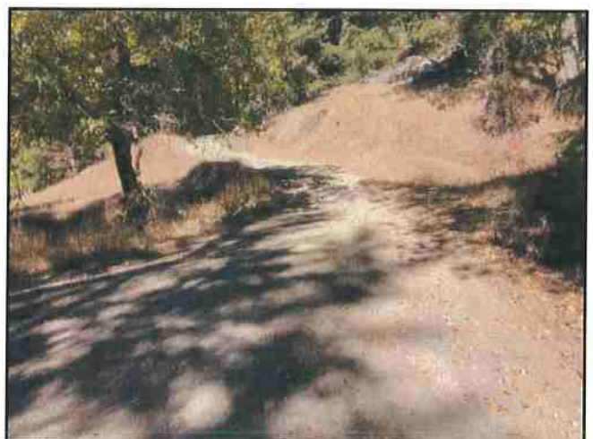
Photo #111 Private Access Rd APN 208-221-014 @ Cultivation / Turnout Area Looking NW
