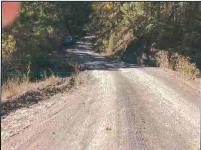
Photo #123 River Rd Looking West @ Curve w/ Turnout
