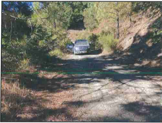
Photo #367 River Rd @ Turnout Location Looking NW
