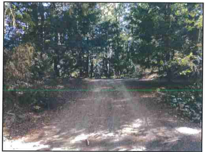
Photo #440 River Rd @ Turnout Location Looking SE @ Curve w/ Turnout
