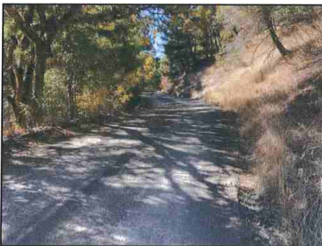
Photo #107 River Rd Looking West @ Curve w/ Turnout
