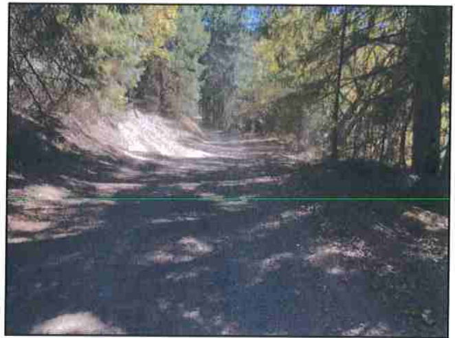
Photo #631 Mad River Trail @ Curve w/ Turnout Looking SE
