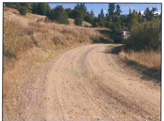
Photo #396 River Rd @ Turnout Location Looking NE @ Curve
