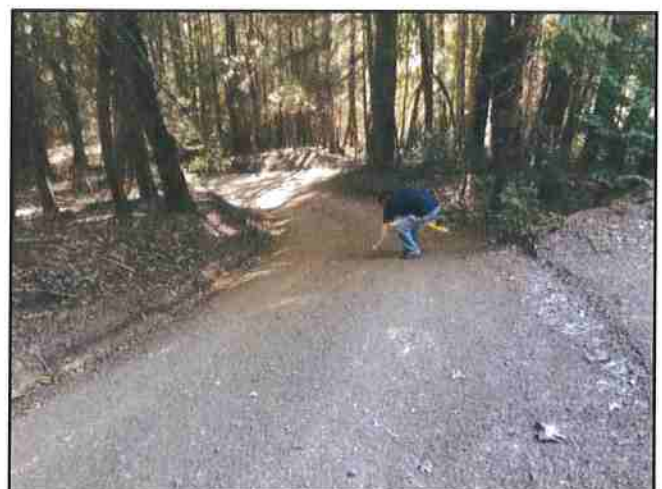
Photo #462 River Rd @ Turnout Location Looking SE @ Curve
