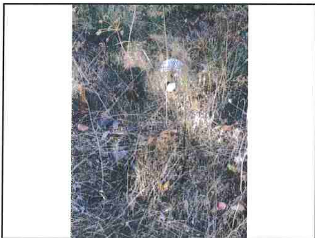
Photo #323 River Rd 24" Culvert In
