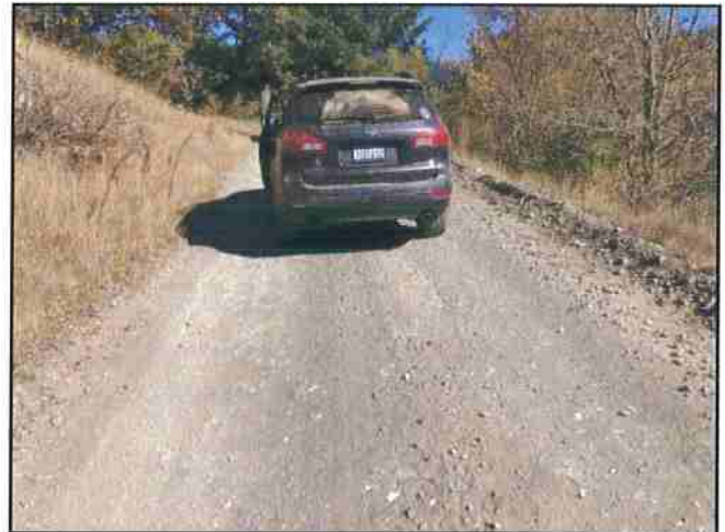
Photo #82 River Rd Looking East
