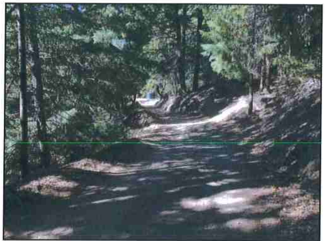
Photo #649 Mad River Trail @ Curve w/ Turnout Looking NW
