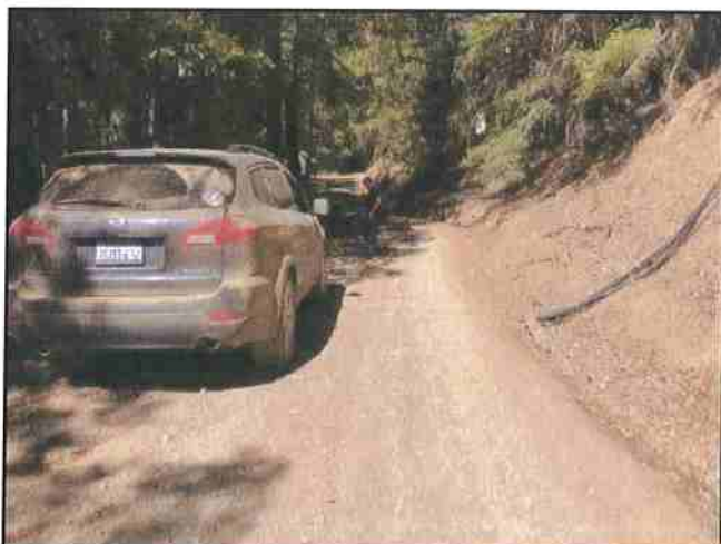
Photo #116 Private Access Rd APN 208-221-014 @ Cultivation / Turnout Area Looking NW
