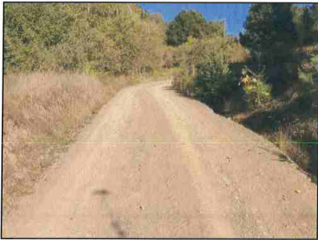
Photo #427 River Rd @ Curve w/ Turnout Looking NE
