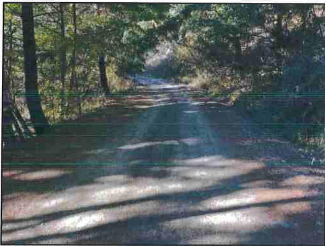
Photo #213 River Rd @ Turnout Looking NW @ Curve
