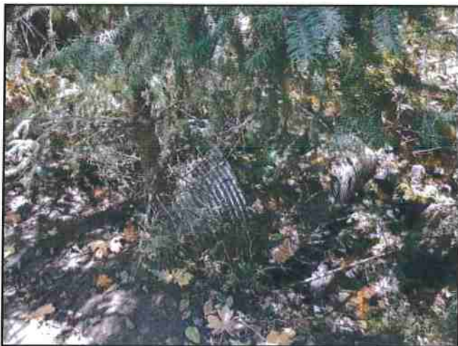
Photo #153 River Rd Looking @ 36" Culvert Out
