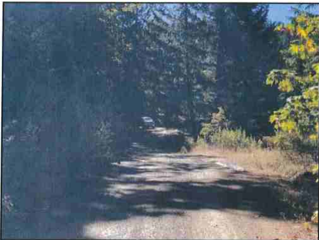
Photo #267 River Rd Looking North @ Curve w/ Turnout
