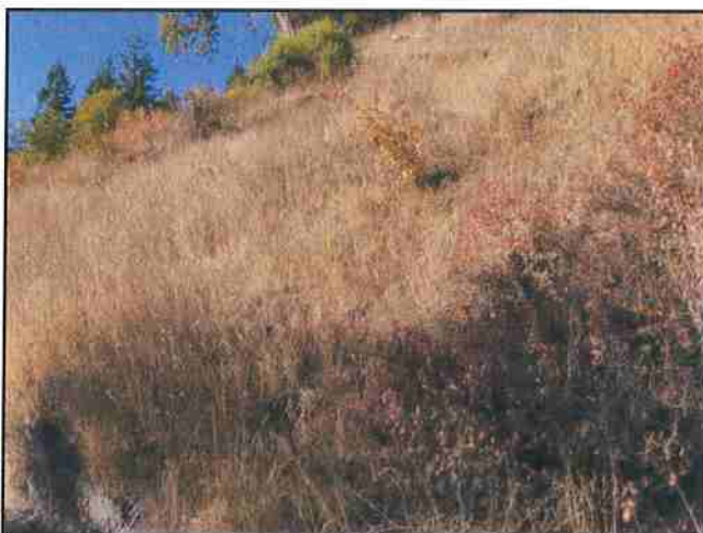
Photo #221 River Rd Looking North @ Hillside Slip
