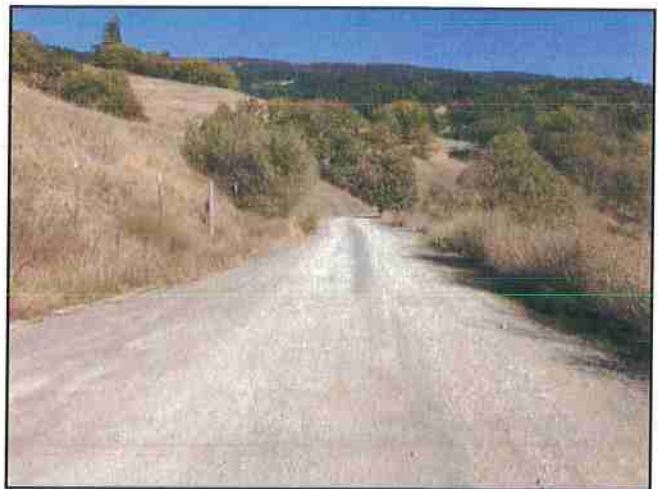
Photo #38 River Rd Looking East
