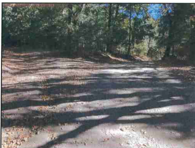
Photo #23 River Rd Looking @ Curve w/ Turnout
