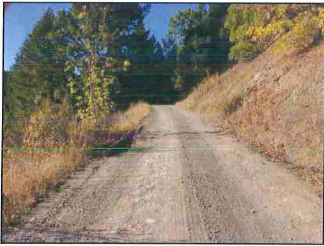
Photo #211 River Rd Looking NW @ Drainage Issue
