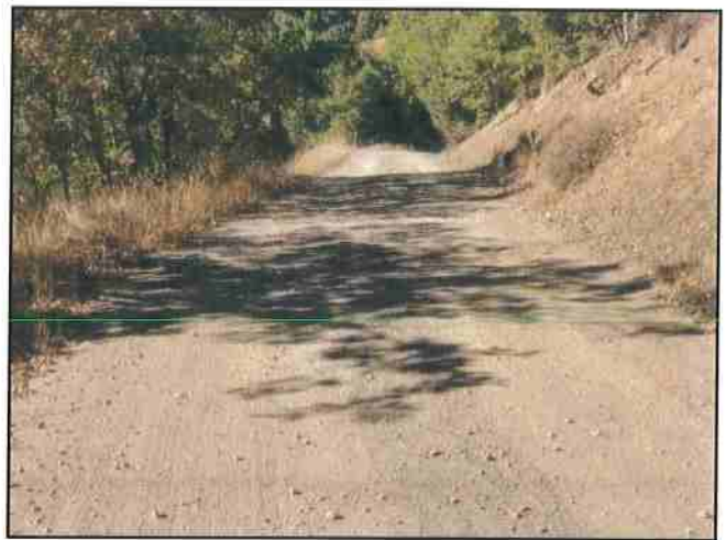
Photo #404 River Rd @ Turnout Location Looking North
