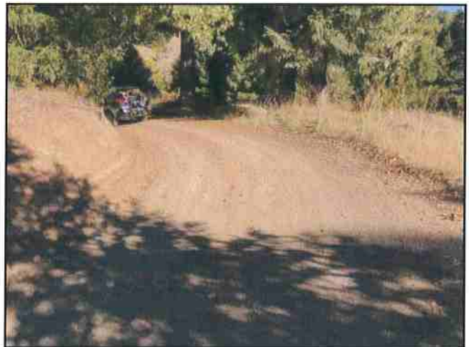
Photo #400 River Rd @ Turnout Location Looking NE @ Curve
