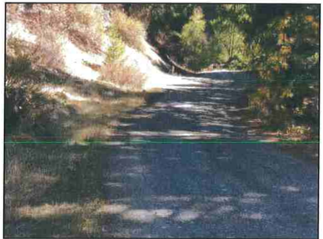
Photo #284 River Rd Looking East @ Curve w/ Turnout & Old Culverts to be removed
