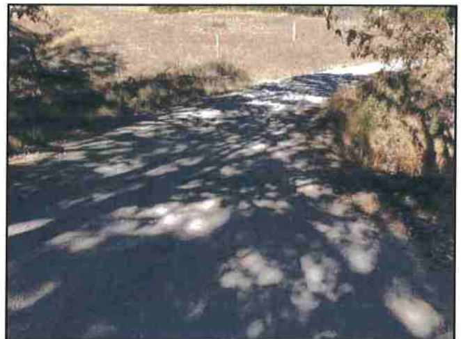
Photo #70 River Rd @ Turnout Looking @ Curve
