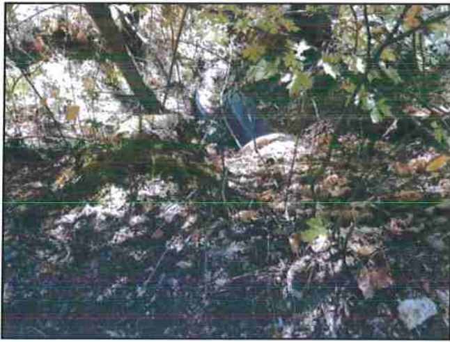
Photo #103 River Rd Looking @ 36" Culvert Out
