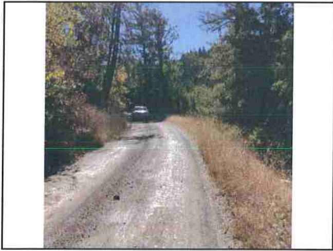
Photo #247 River Rd Looking North @ Curve w/ Pullout.
