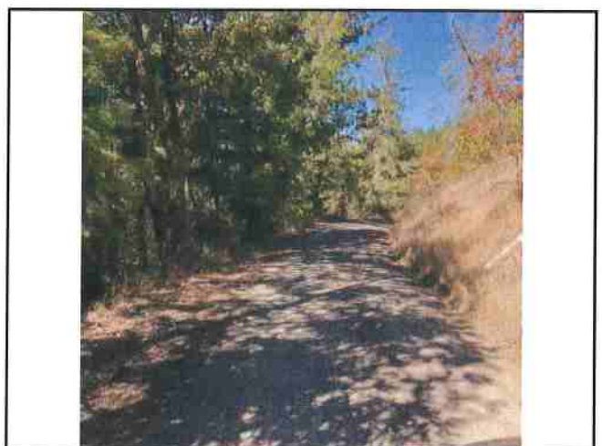
Photo #246 River Rd Looking NW @ Curve w/ Turnout
