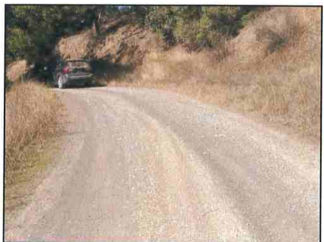
Photo #258 River Rd @ Turnout Lookng NW @ Curve
