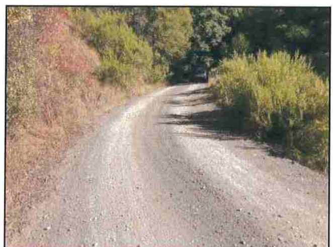
Photo #360 River Rd @ Turnout Location Looking NE @ Curve
