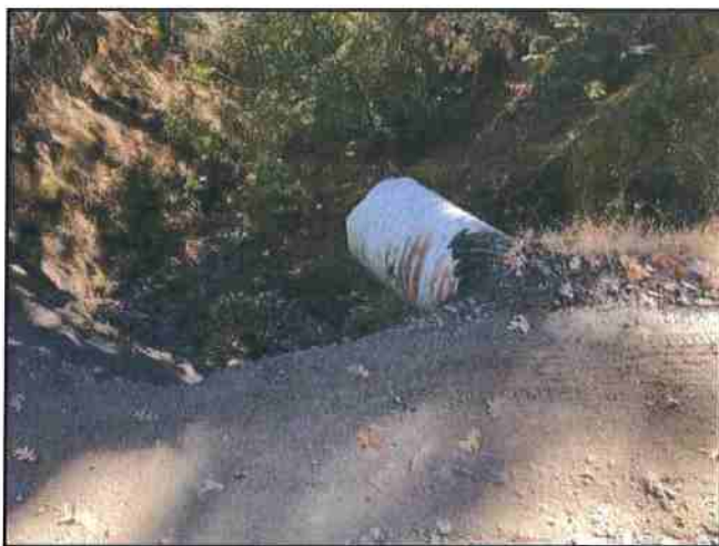
Photo #89 River Rd Looking @ 24" Culvert Out
