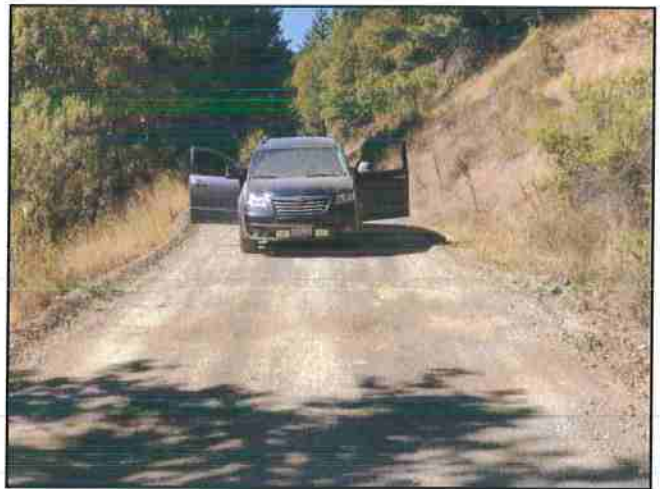
Photo #140 River Rd Looking West @ Drainage Issue
