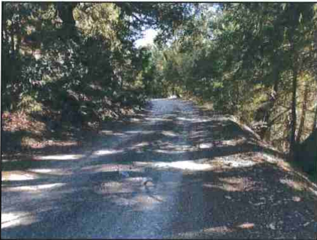
Photo #381 River Rd @ Turnout Location Looking SE @ Curve
