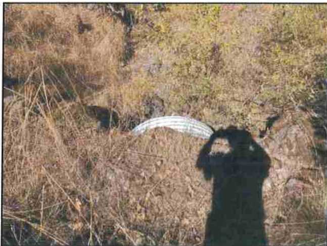
Photo #63 River Rd Looking @ 36" Culvert Out (Dual?)
