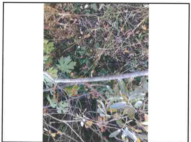
Photo #204 River Rd Looking @ 12" Culvert Out
