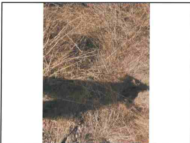
Photo #29 River Rd Looking @ Clogged 12" Culvert In
