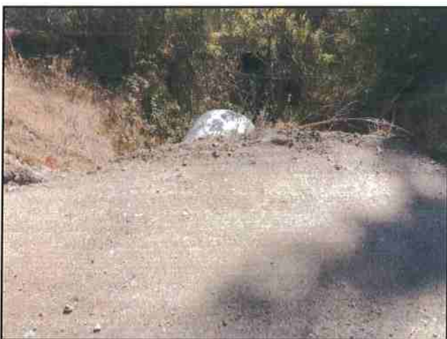
Photo #125 River Rd Looking @ 36" Culvert Out
