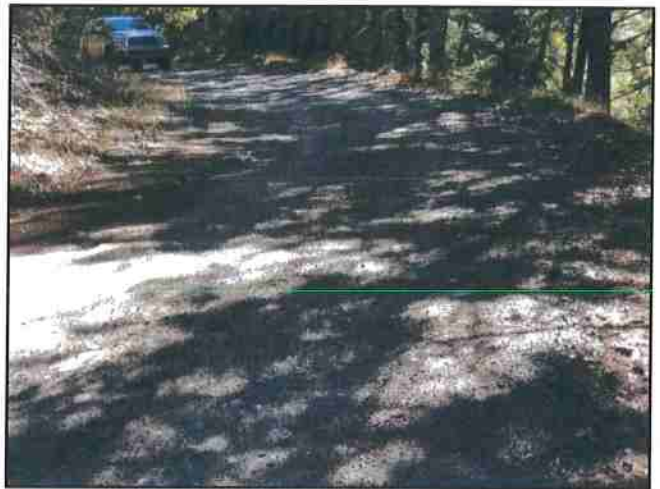
Photo #290 River Road Looking North @ Curve w/ Turnout
