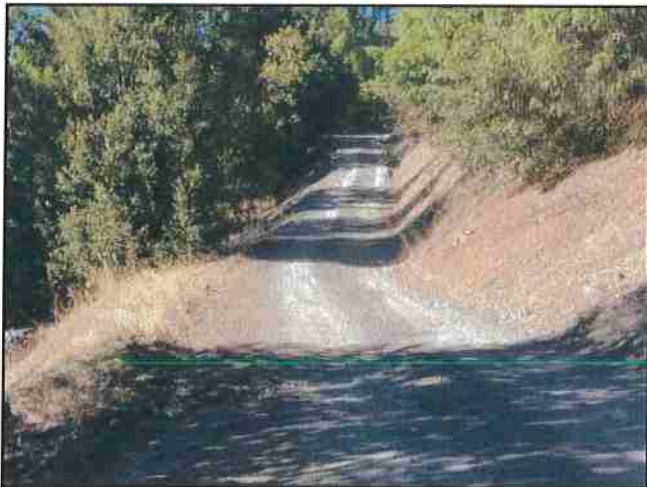
Photo #345 River Rd @ Turnout Location Looking NW
