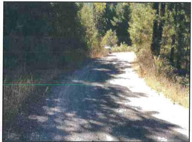
Photo #272 River Rd Looking North @ Curve w/ Turnout
