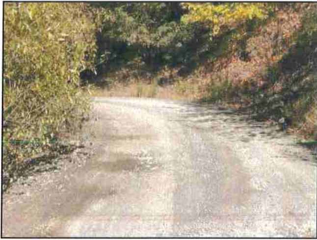
Photo #277 River Rd Looking North @ Curve w/ Turnout
