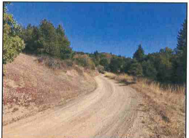
Photo #418 River Rd @ Curve w/ Turnout Looking SE
