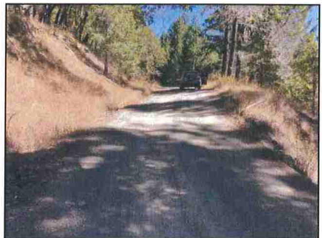
Photo #174 River Rd Looking NE @ Curve w/ Pullout
