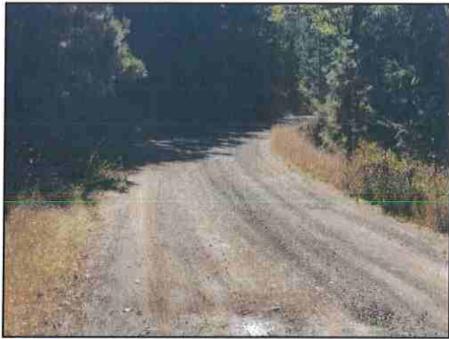
Photo #271 River Rd Looking South @ Curve w/ Turnout
