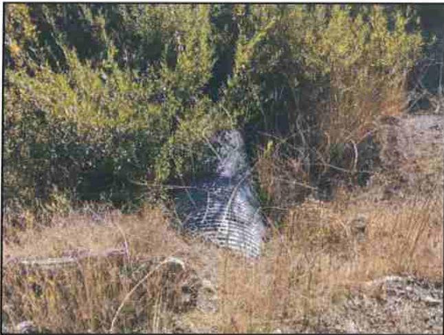
Photo #15 River Rd Looking @ 36" Culvert In
