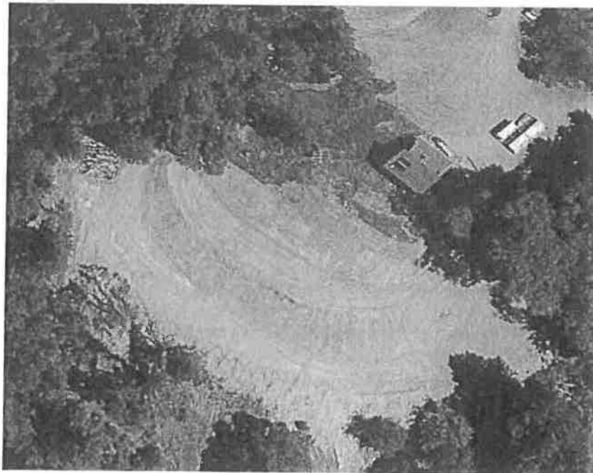
Picture 4: CS #3 consists of a hillside developed into two terraces that contain greenhouses. Photo date: 05/26/2016
