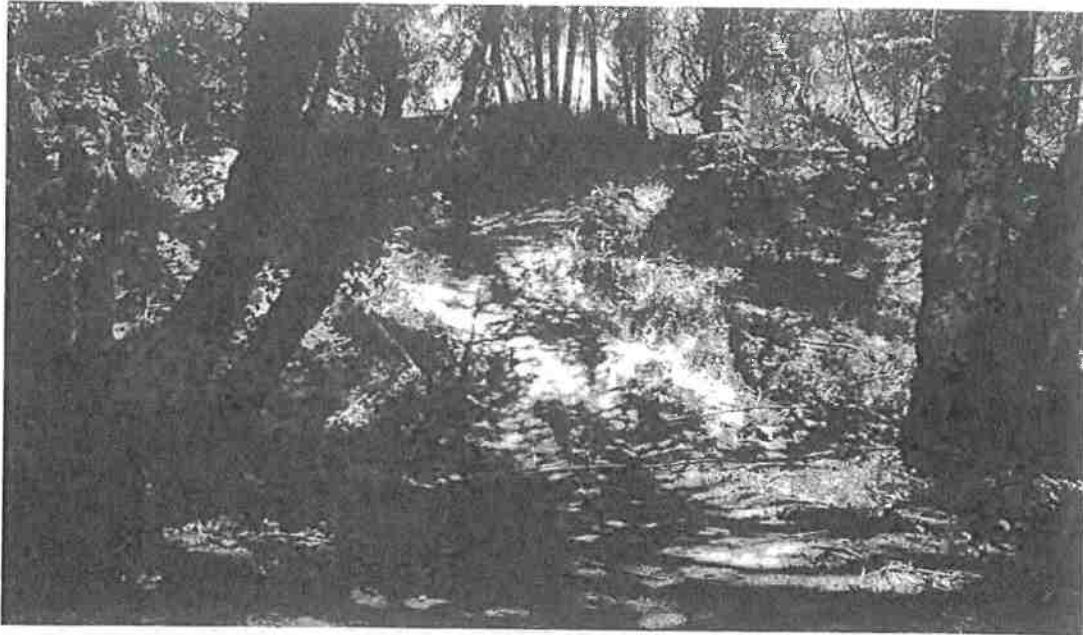
Picture 18: SC #2 consists of a dirt ford located on a Class III watercourse. The Discharger shall decommission and abandon this location by seeding and mulching the site with a native riparian seed mix. Also seen in this picture is the road segment located at MP #4. This road shall be decommissioned by the Discharger per attached BMP specifications. Photo date: 07/14/2016
