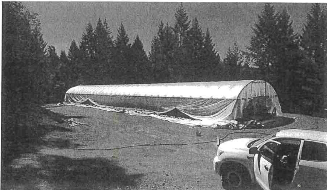
Picture 2: Fifth greenhouse located at CS #1. Photo date: 07/14/2016
