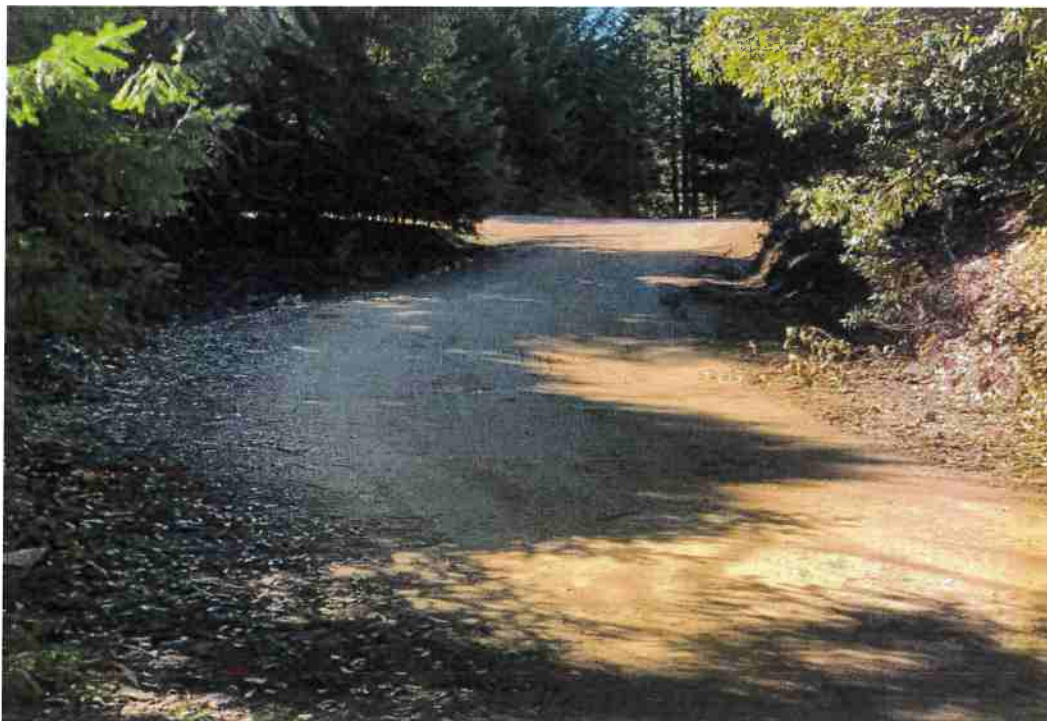
Figure 32: RP 23 on Old 3 Creeks Rd.
