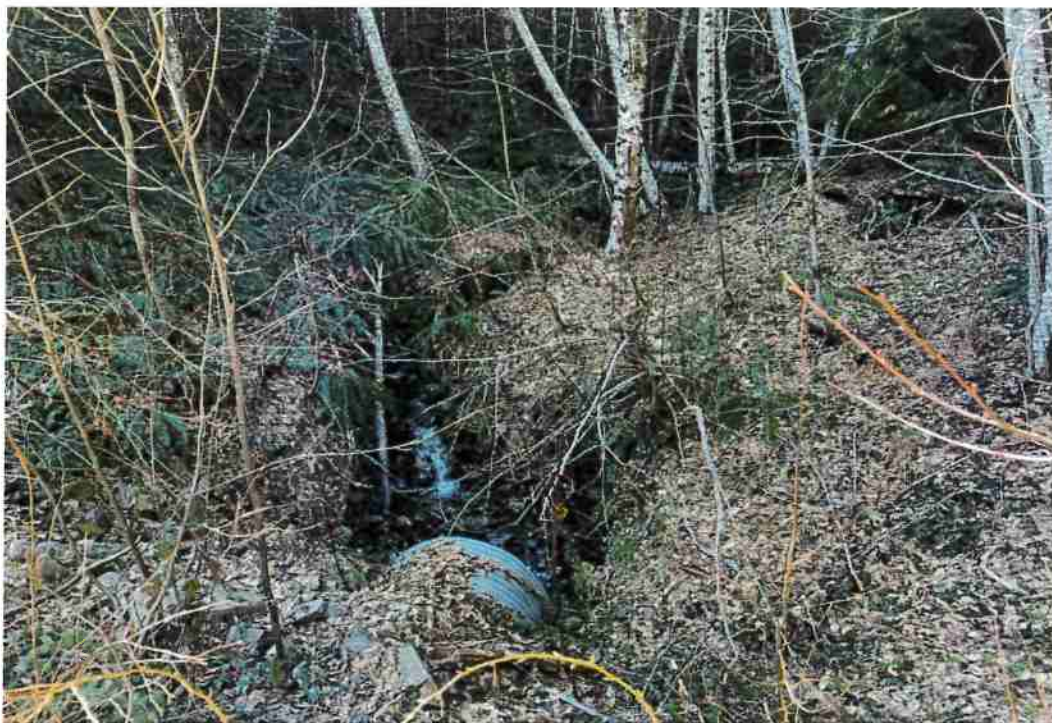
Figure 9: RP 6 on Supply Creek Rd.
