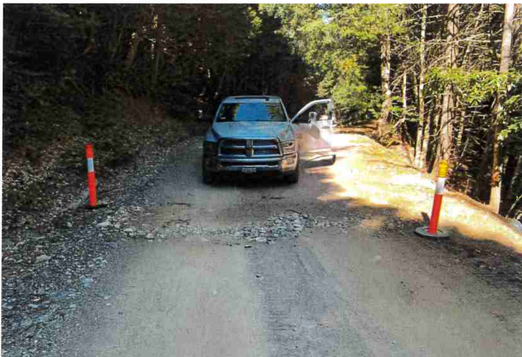
Figure 25: RP 22 on Old 3 Creeks Rd.
