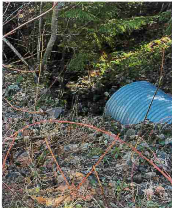
Figure 4: RP 4 on Supply Creek Rd.
