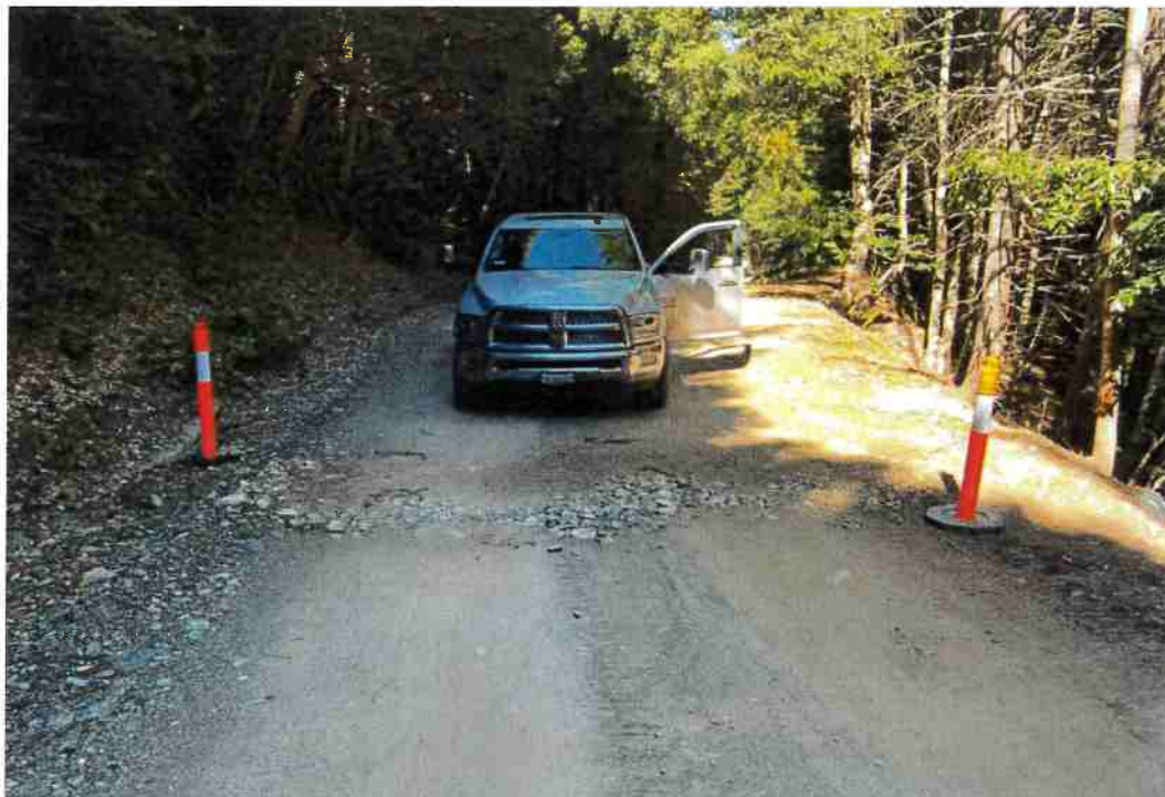
Figure 25: RP 22 on Old 3 Creeks Rd.
