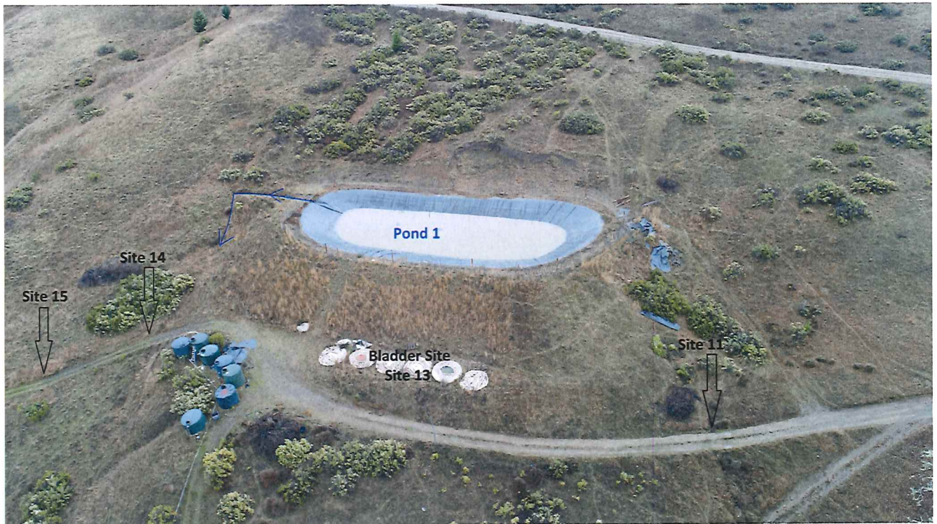
Photo shows the area around Pond 1. Water from the outflow appears to disperse or go subsurface before reaching a stream. See the Mitigation Report for details and prescribed actions needed at Site 11, 13, 14, and 15. Photo date 12/15/2020.
