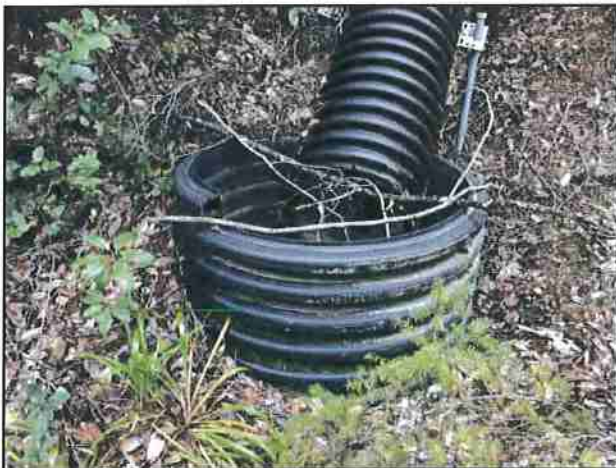
Photo #209 Kings Peak Rd Looking @ 18" Culvert Down Slope In
