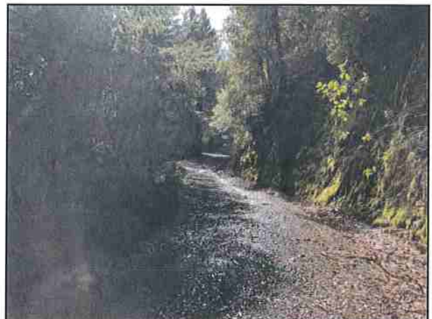
Photo #148 Kings Peak Rd @ Curve w/ Pullout Looking NE
