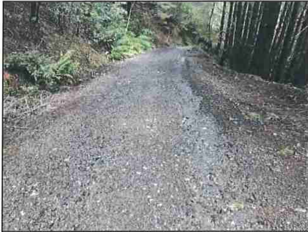
Photo #153 Kings Peak Rd @ Curve w/ Pullout Looking NE
