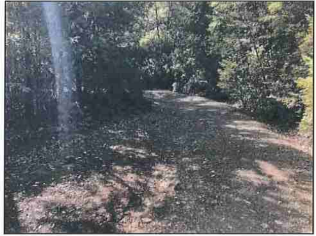
Photo #68 Kings Peak Rd @ Curve w/ Pullout Looking NE @ Rutting
