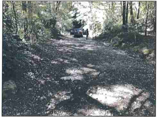
Photo #92 Kings Peak Rd @ Curve w/ Pullout Looking SW
