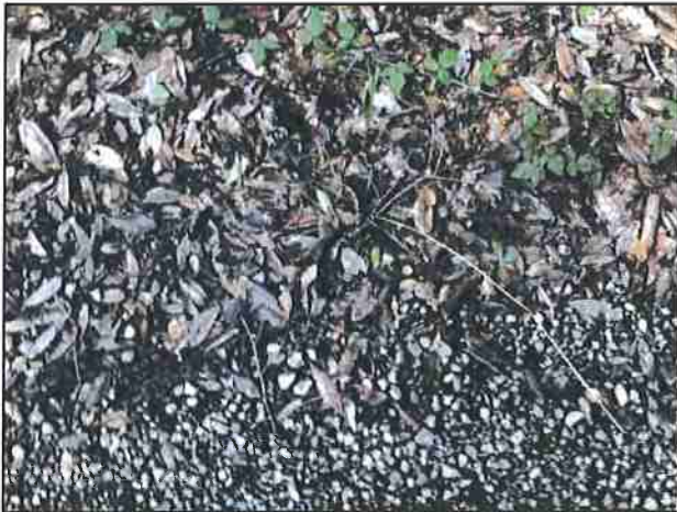
Photo #129 Kings Peak Rd Looking @ 18" Culvert In
