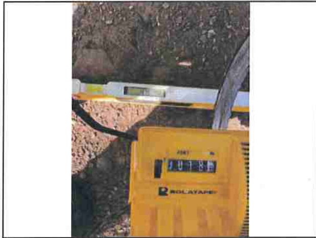
Photo #69 Kings Peak Rd Slope 4.8% Width 18'10"
