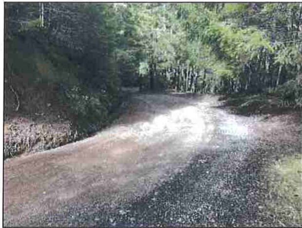
Photo #145 Kings Peak Rd @ Curve w/ Pullout Looking NE
