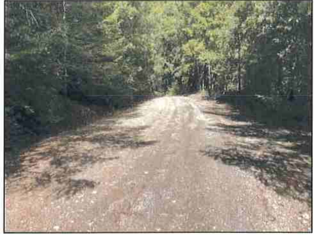
Photo #110 Kings Peak Rd @ Curve w/ Pullout Looking NE
