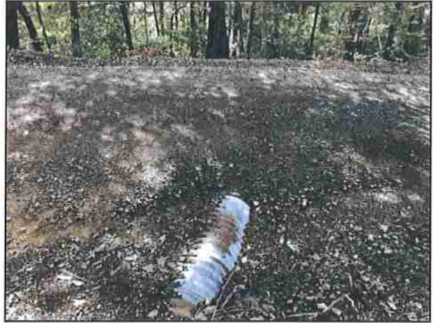
Photo #188 Kings Peak Rd Looking @ Exposed 18" Culvert
