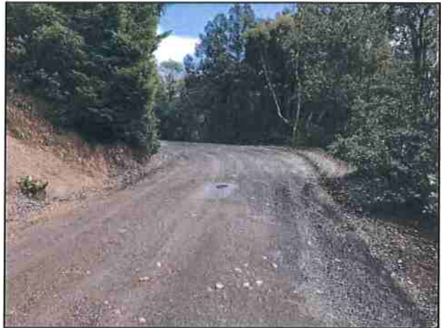
Photo #214 Kings Peak Rd @ Curve w/ Pullout Looking NE
