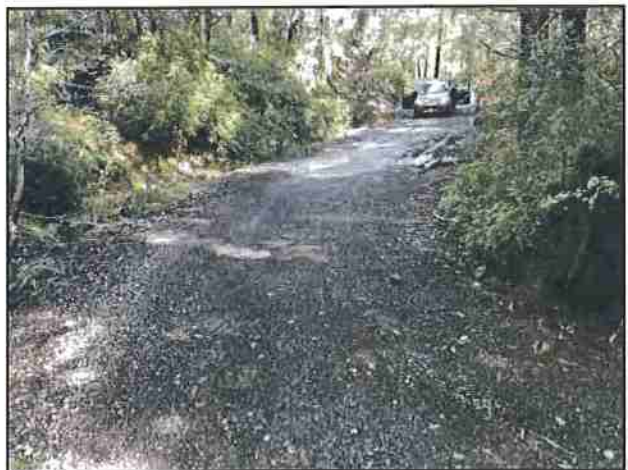
Photo #90 Kings Peak Rd @ Curve w/ Pullout Looking NE
