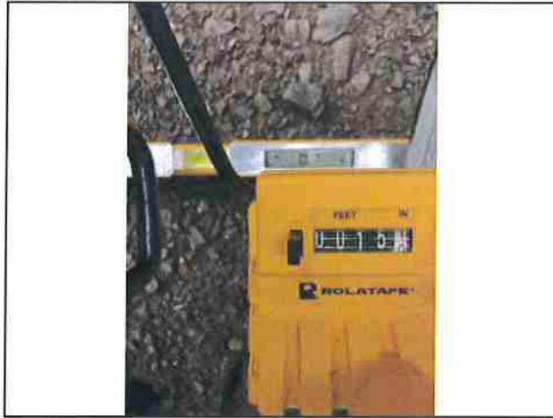
Photo #199 Kings Peak Rd Slope 0.7% Width 15'1"
