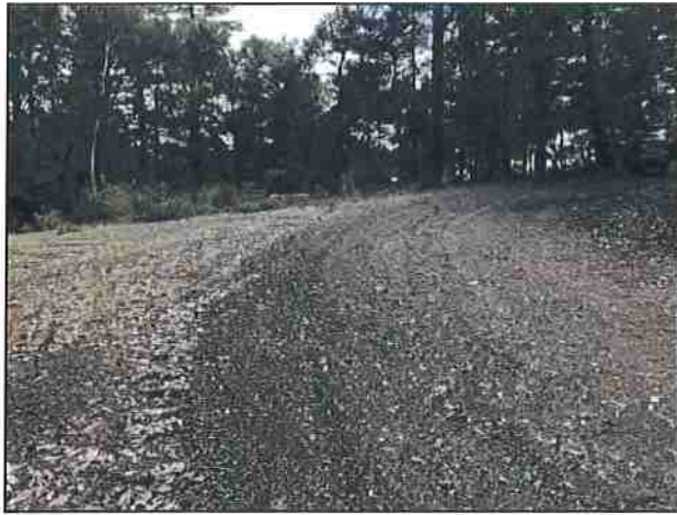
Photo #157 Kings Peak Rd @ Curve w/ Pullout Looking SW
