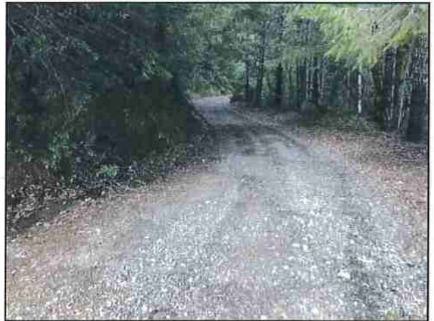
Photo #156 Kings Peak Rd @ Curve w/ Pullout Looking NE
