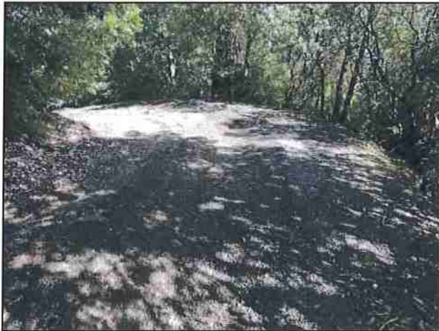
Photo #39 Private Access Rd @ Curve w/ Pullout Looking NE
