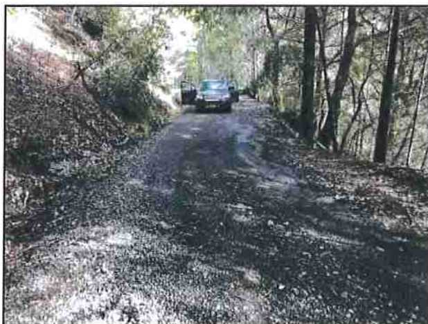
Photo #149 Kings Peak Rd @ Curve w/ Pullout Looking SW
