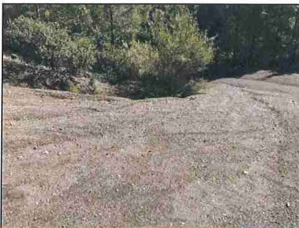
Photo #179 Kings Peak Rd @ Curve w/ Pullout Looking SW
