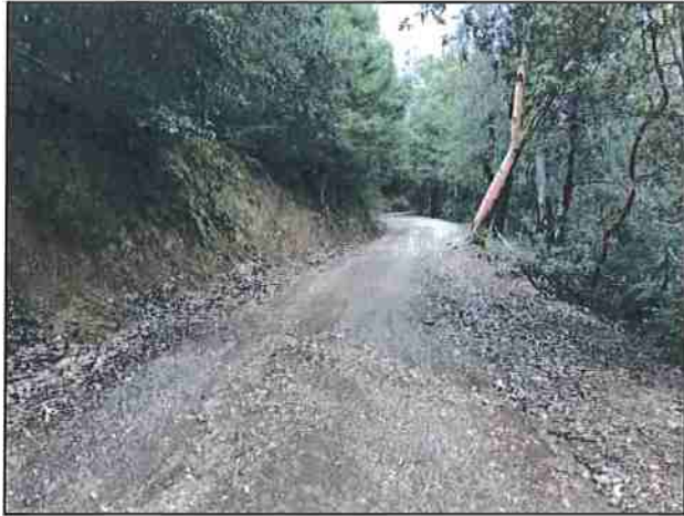
Photo #211 Kings Peak Rd @ Curve w/ Pullout Looking NE
