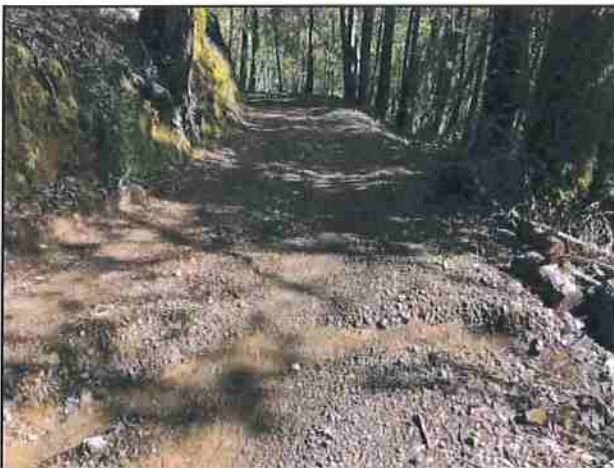
Photo #29 Private Access Rd @ Curve w/ Pullout Looking NE
