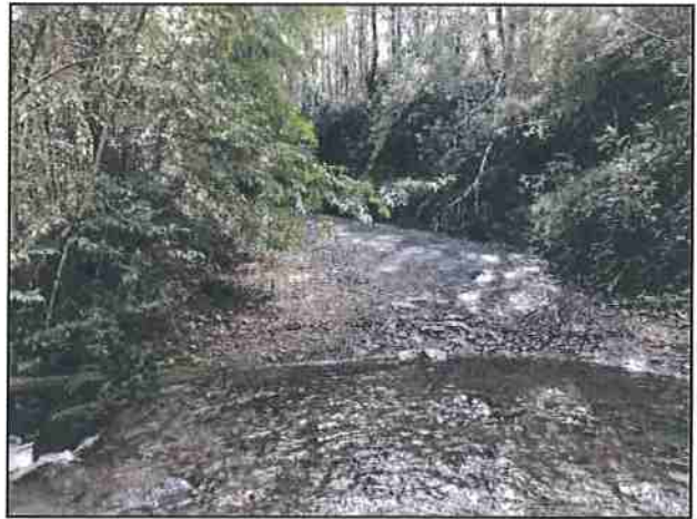
Photo 94 Kings Peak Rd Looking @ Stream Crossing on Road (Culvert Needed)
