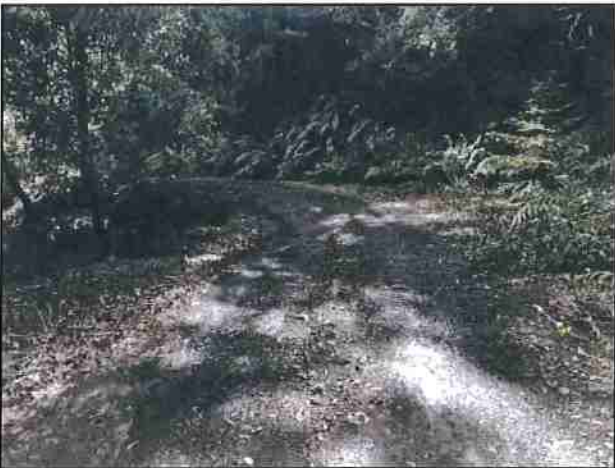
Photo #191 Kings Peak Rd @ Curve w/ Pullout Looking SW
