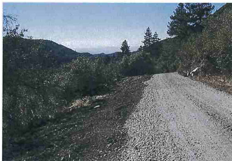
Figure 1. Low-volume road that has been newly gravelled and out-sloped, San Bernardino County. Photo: Richard Harris.
