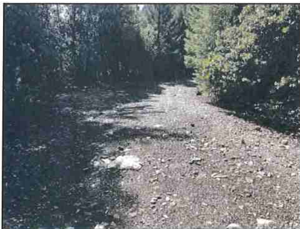
Photo #101 Kings Peak Rd @ Curve w/ Pullout Looking SW
