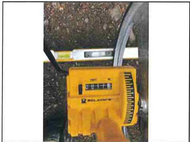
Photo #216 Kings Peak Rd Slope 1.0% Width 17'3"
