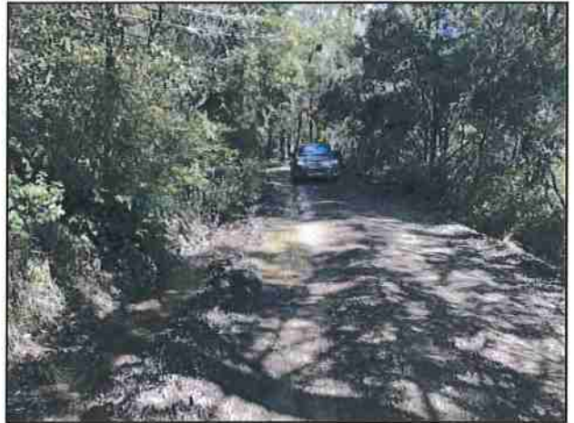
Photo #76 Kings Peak Rd @ Pullout Looking NE @ Drainage Issue
