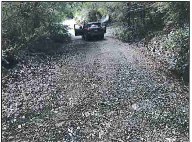
Photo #138 Kings Peak Rd @ Curve w/ Pullout Looking SW
