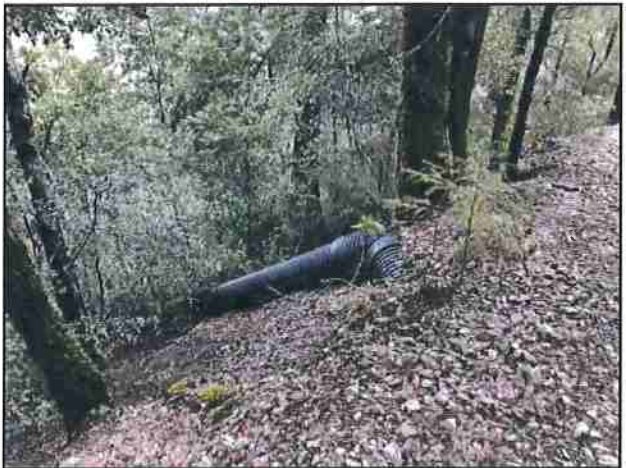
Photo #210 Kings Peak Rd Looking @ 18" Culvert Down Slope Out
