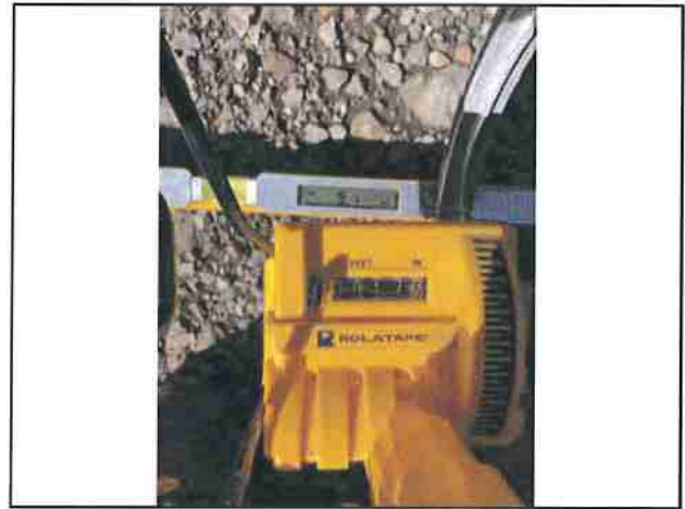
Photo #100 Kings Peak Rd Slope 9.1% Width 17'5"
