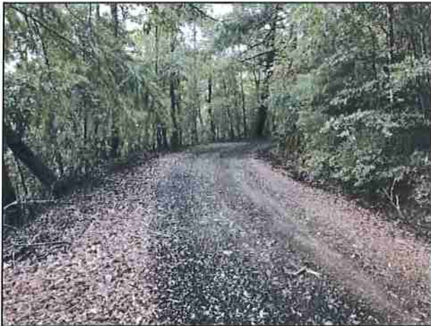
Photo #159 Kings Peak Rd @ Curve w/ Pullout Looking SW
