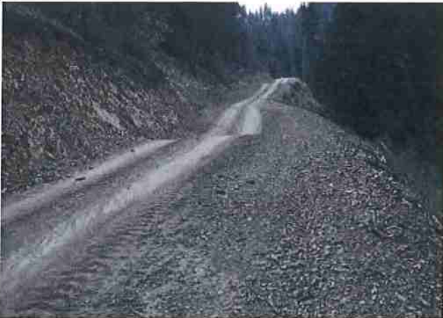
Figure 8. Rolling dips installed to drain an out-sloped road. Source: Bill Weaver, Pacific Watershed Associates.
