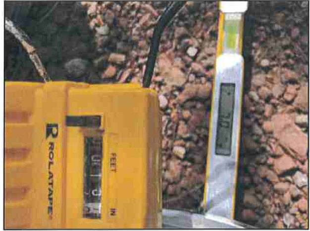
Photo #56 Kings Peak Rd Slope 7.0% Width 15'7"
