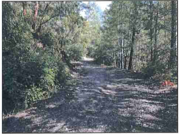
Photo #86 Kings Peak Rd @ Curve w/ Pullout Looking NE
