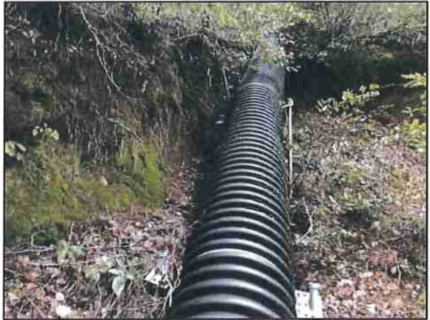
Photo #208 Kings Peak Rd Looking @ 18" Culvert Down Slope
