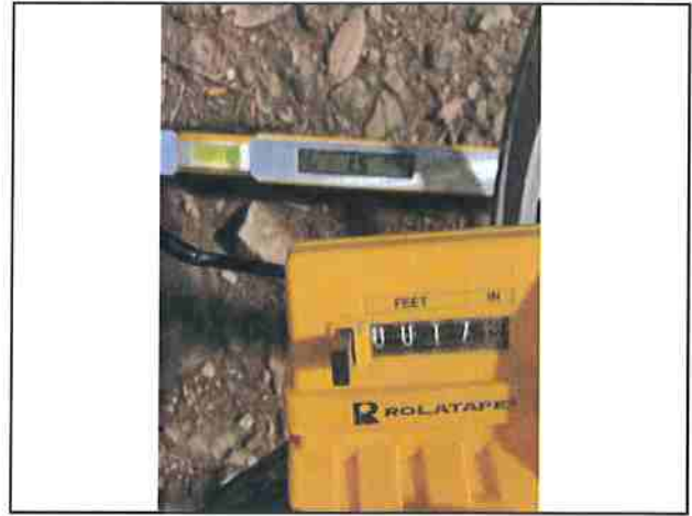
Photo #98 Kings Peak Rd Slope 1.5% Width 17'5"
