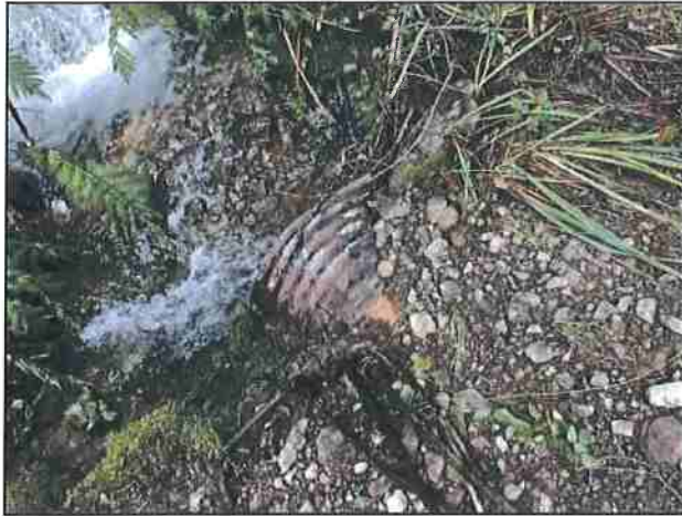
Photo #127 Kings Peak Rd Looking @ 18" Culvert In
