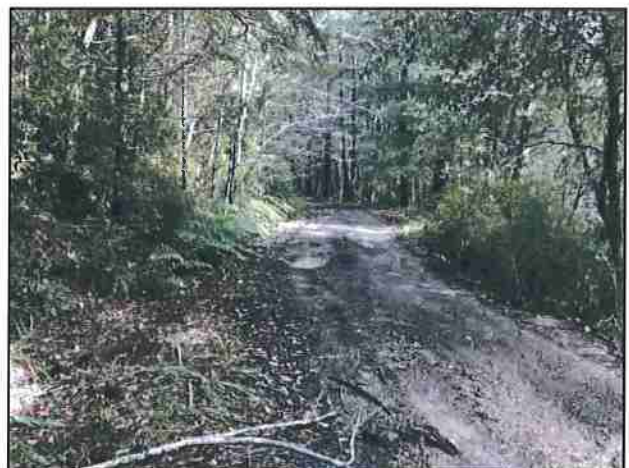
Photo #126 Kings Peak Rd @ Curve w/ Pullout Looking NE
