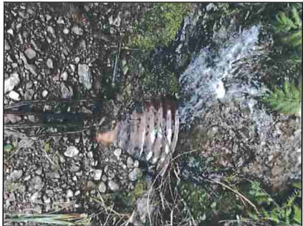
Photo #124 Kings Peak Rd Looking @ 18" Culvert In
