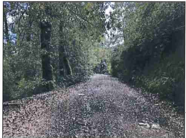
Photo #132 Kings Peak Rd @ Curve w/ Pullout Looking NE
