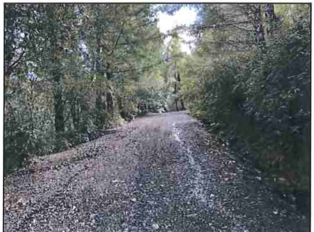
Photo #144 Kings Peak Rd @ Pullout Looking SE
