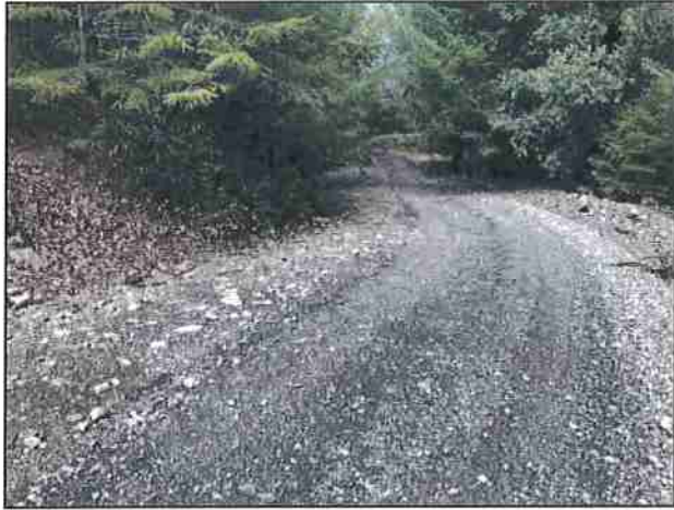
Photo #133 Kings Peak Rd @ Curve w/ Pullout Looking NE
