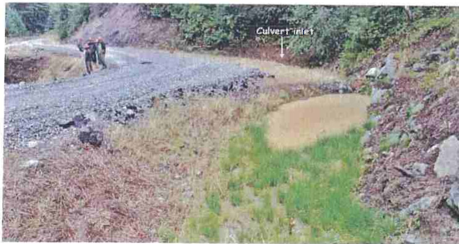
FIGURE 238. Traffic and surface runoff from gravelled roads often produces surface erosion, turbid runoff and fine sediment transport that can be delivered to streams. Where ditches can't be eliminated, sediment traps and roadside settling basins can be installed to capture and remove most of the eroded sediment. This settling basin has been constructed along the inside ditch just before a stream crossing culvert inlet (see arrow). Eroded sediment from the road and ditch are deposited in the basin before flow is released to the stream. Fine sediments have filled about 1/3 of this basin and vegetation is now growing. Sediment basins require periodic maintenance to maintain their storage capacity.
