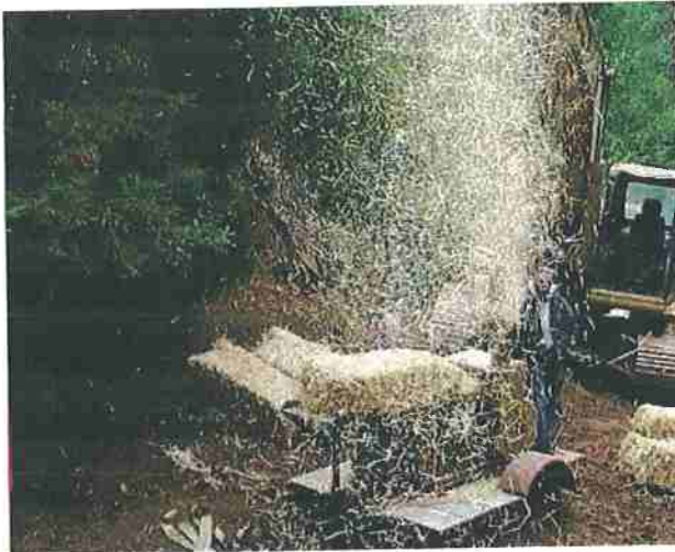
Figure 40. Using a portable blower to spread straw mulch on a disturbed road site. Photo: Julie Bawcom, California Geological Survey.
