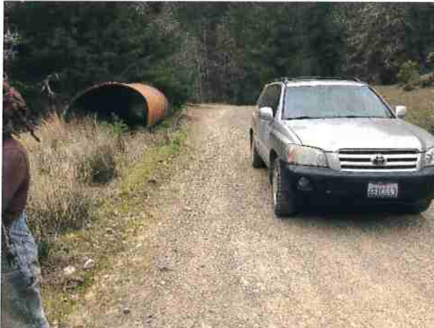
Photo #185 Unnamed Rd Looking West @ Tank
