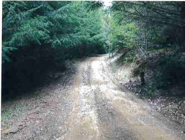
Photo #5 @ Access Rd Looking Northwest
