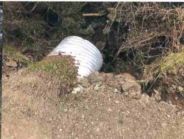
Photo #208 Unnamed Rd Looking @ 36" Culvert Out
