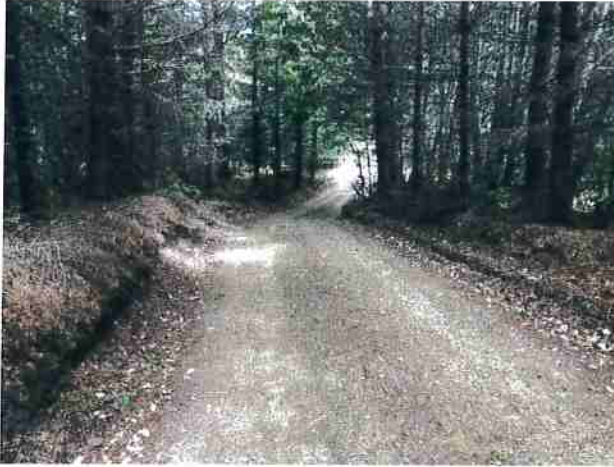
Photo #37 Access Rd Looking Northeast
