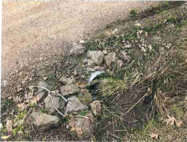
Photo #153 @ Unnamed Rd Looking @ 12" Culvert In
