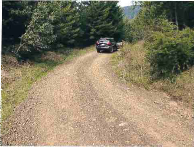
Photo #39 Access Rd Looking North @ Curve w/Pullout
