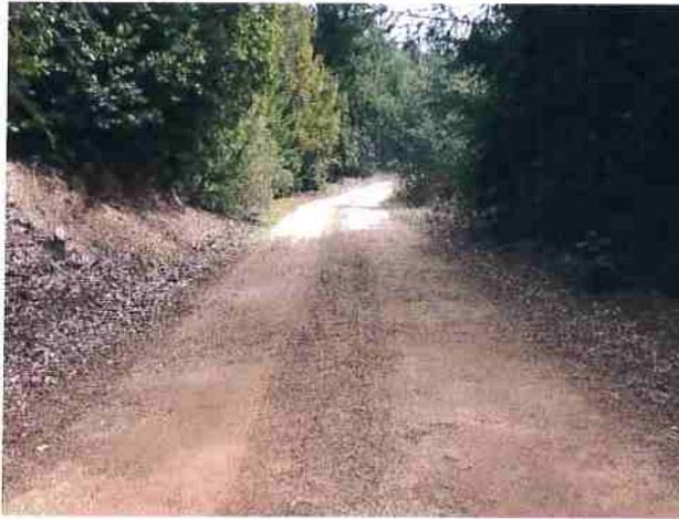
Photo #25 Access Rd Looking Southwest @ Curve w/Pullout
