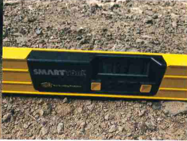
Photo #44 Access Rd @ Grade Steeper than 16%
