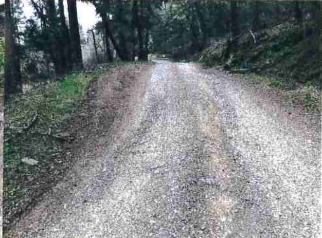
Photo #219 Unnamed Rd Looking @ Erosion From Clogged Culvert
