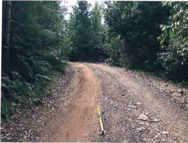
Photo #45 Access Rd Looking Southwest @ Curve w/Pullout
