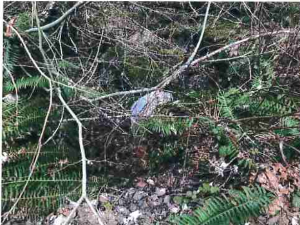
Photo #173 Unnamed Rd Looking @ 18" Culvert Out
