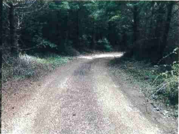
Photo #20 Access Rd Location with Grade Greater Than 16%
