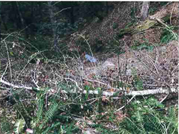
Photo #106 @ Unnamed Rd Looking @ 12" Culvert
