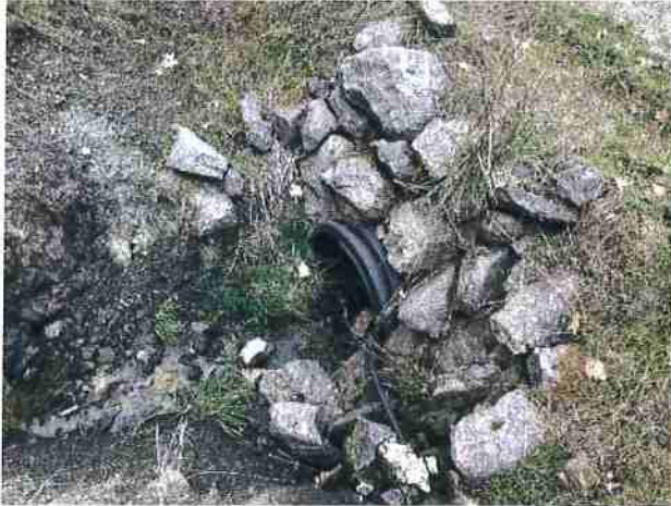
Photo #133 @ Unnamed Rd Looking @ 12" Culvert In
