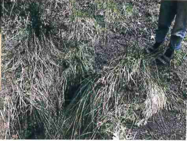
Photo #152 @ Unnamed Rd Looking @ 12" Culvert Out
