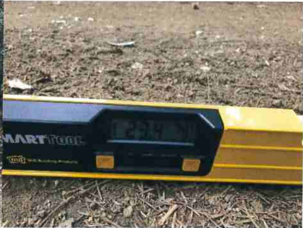
Photo #32 Access Rd Looking @ Grade Steeper Than 16%
