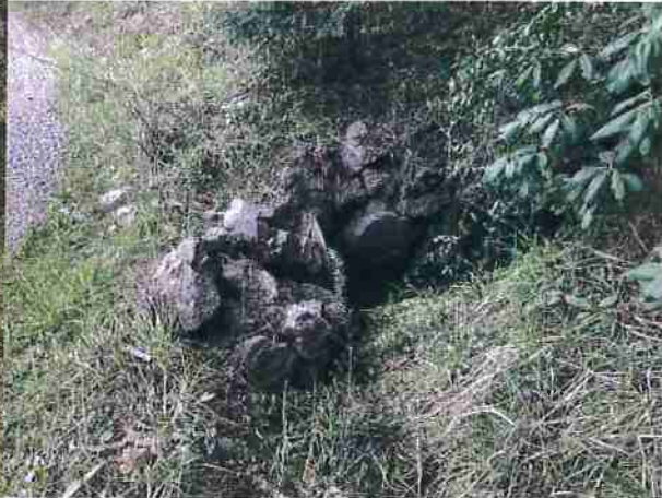
Photo #146 @ Unnamed Rd Looking @ 12" Culvert In
