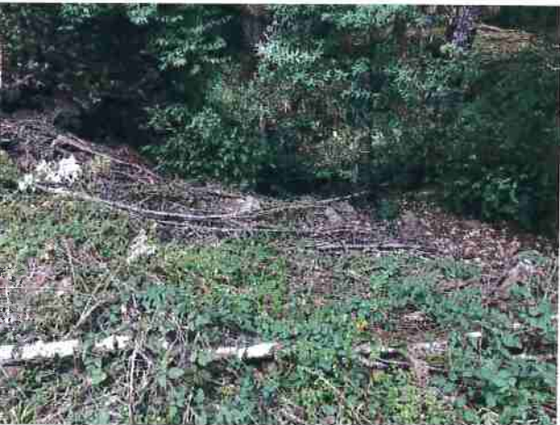
Photo #88 @ @ Unnamed Rd 12" Culvert Outlet
