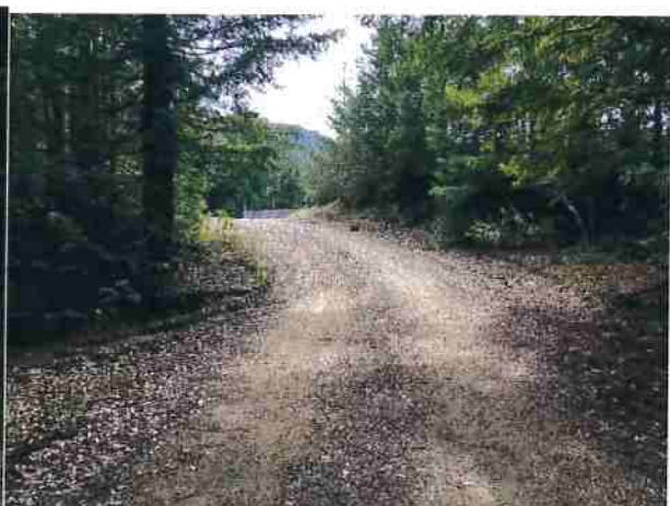
Photo #30 Access Rd Looking Southwest @ Curve w/Pullout
