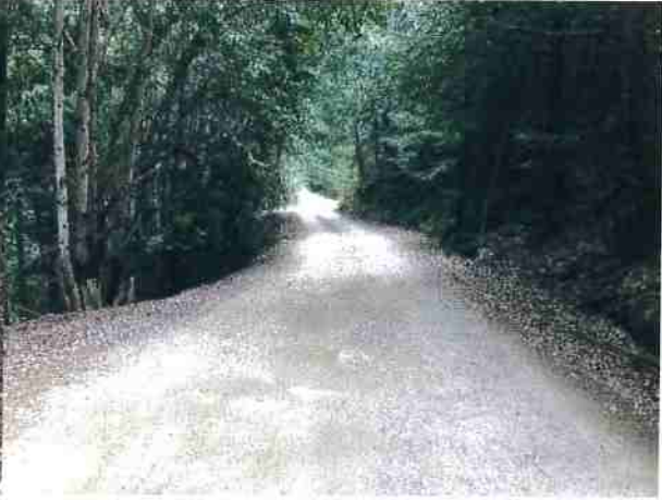
Photo #122 @ Unnamed Rd Curve Looking Southeast
