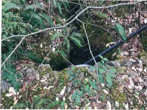
Photo #87 @ Unnamed Rd 12" Culvert Inlet
