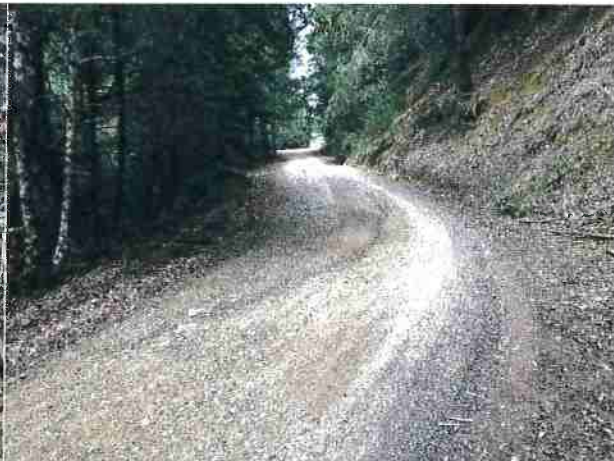
Photo #108 @ Unnamed Rd @ Curve Looking Southeast
