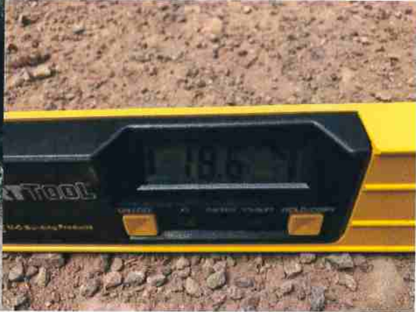
Photo #92 @ Unnamed Rd Steep Grade
