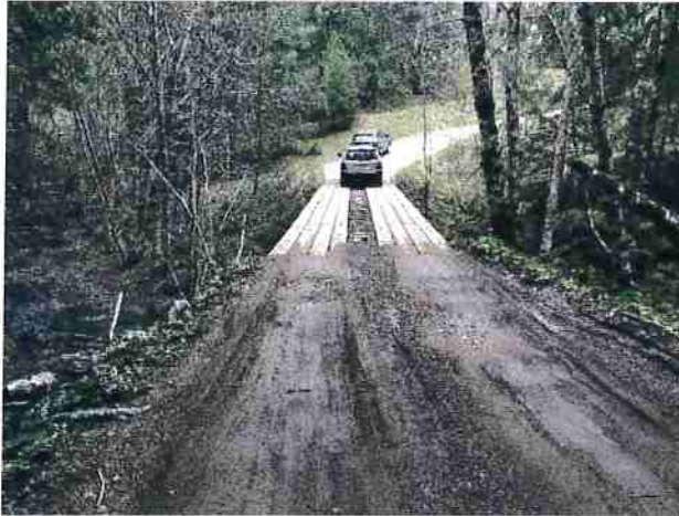
Photo #177 Railroad Car Bridge Looking North
