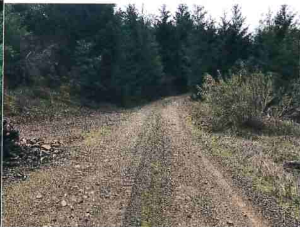
Photo #48 Access Rd Looking Southwest @ Curve w/Pullout
