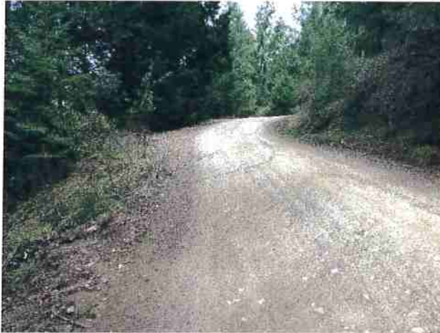
Photo #93 @ Unnamed Rd Looking NE @ Curve
