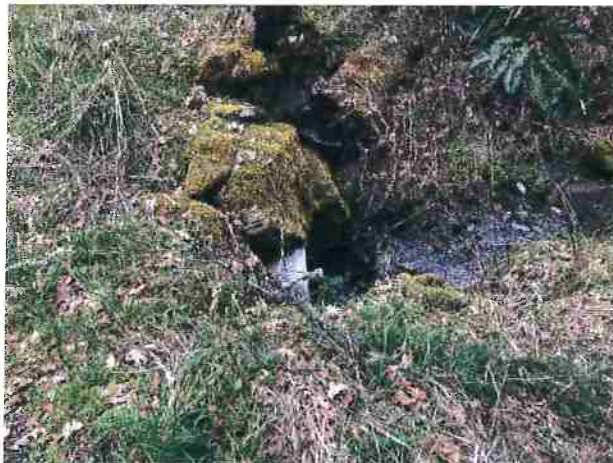
Photo #209 Unnamed Rd Looking 36" Culvert In
