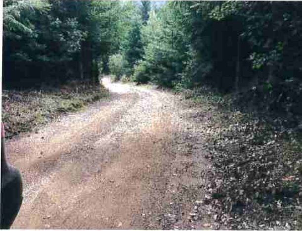
Photo #19 Access Rd Looking Southwest @ Curve w/Pullout
