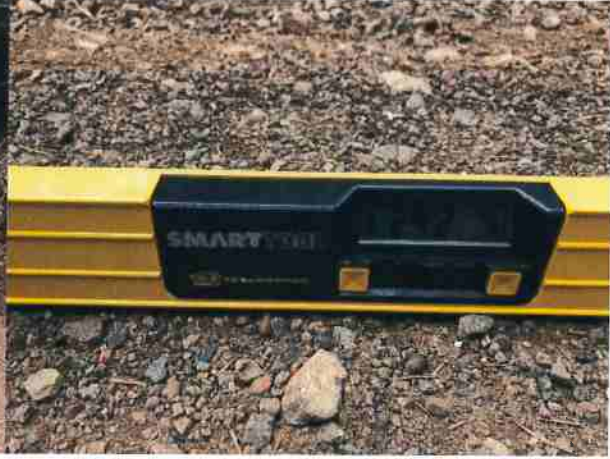
Photo #50 Access Rd @ Grade Steeper than 16%
