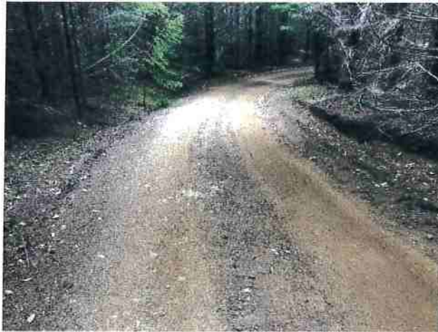
Photo #15 Access Rd Looking Northwest @ curve w/Pullout
