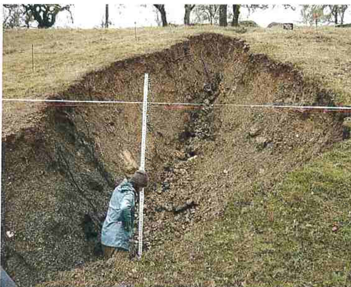
Figure 22. Gully caused by through-cut on road at base of steep road section. Photo: Jared Gerstein.
