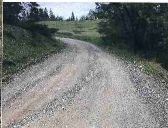
Photo #192 Unnamed Rd Looking East
