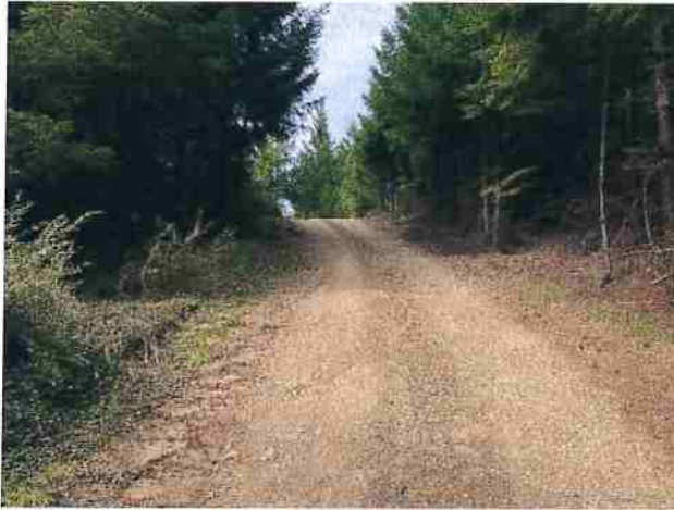
Photo #21 Access Rd Looking Northwest
