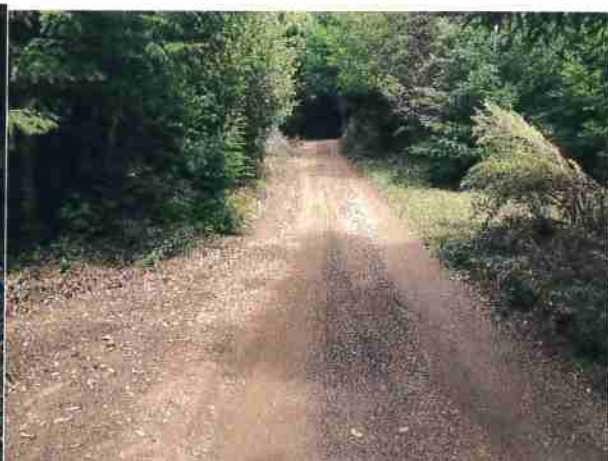
Photo #18 Access Rd Looking Northeast w/Pullout
