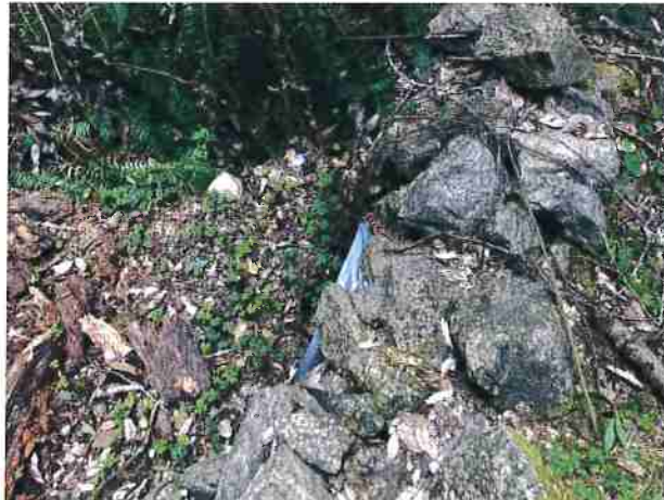
Photo #107 @ Unnamed Rd 12" Culvert
