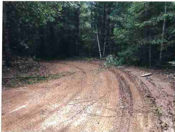
Photo #11 Access Rd Looking South @ Curve w/Pullout
