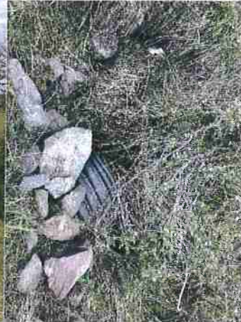
Photo #140 @ Unnamed Rd Looking @ 12" Culvert In
