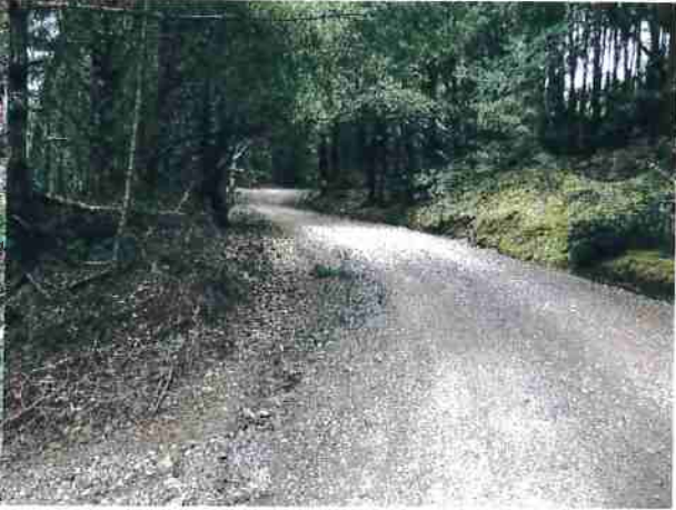
Photo #98 @ Unnamed Rd Looking Southwest
