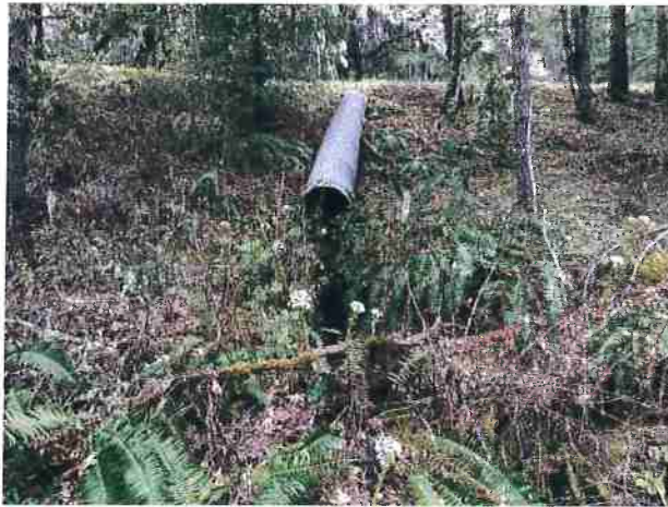
Photo #225 Unnamed Rd Looking @ 24" Culvert Out
