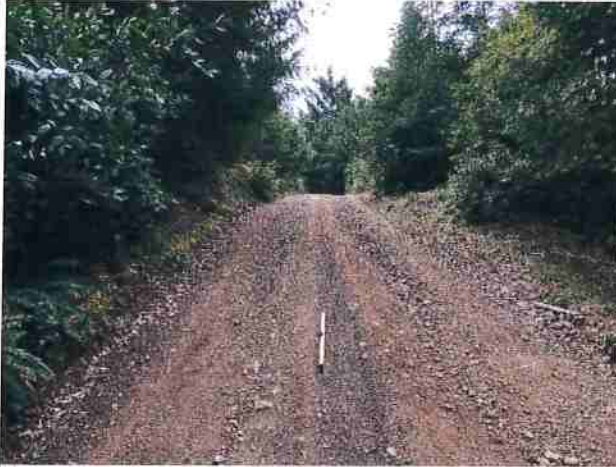
Photo #51 Access Rd Looking Southwest
