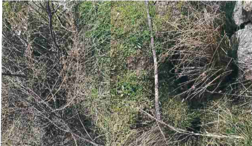
Photo #141 @ Unnamed Rd Looking @ 12" Culvert Out
