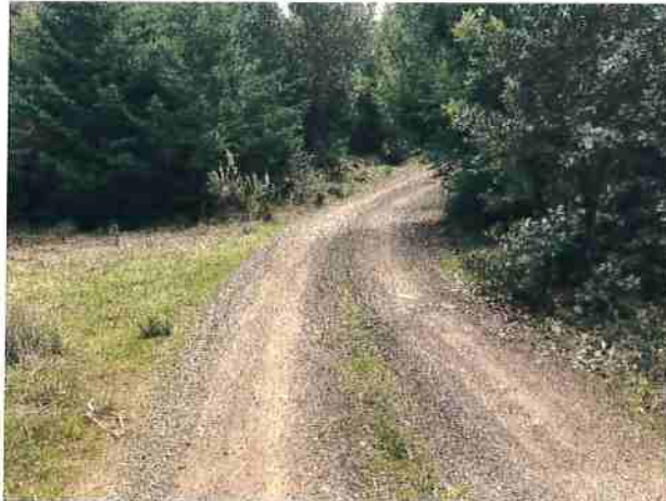
Photo #41 Access Rd Looking South @ Curve w/Pullout
