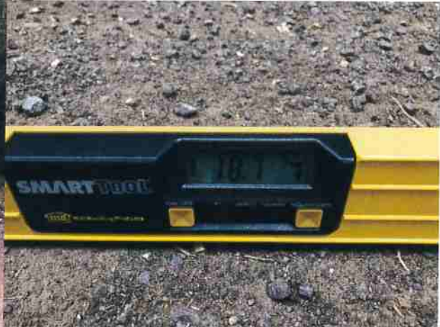
Photo #82 @ @ Unnamed Rd Steep Grade
