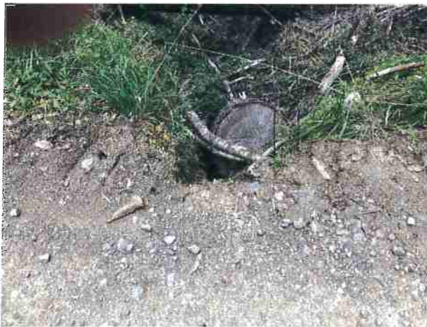
Photo #219 Unnamed Rd Looking @ Erosion From Clogged Culvert
