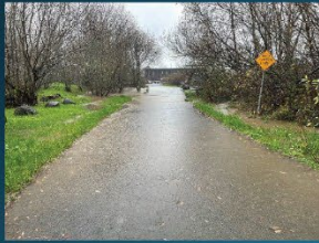
14 th Street looking west to Bob's Lumber
