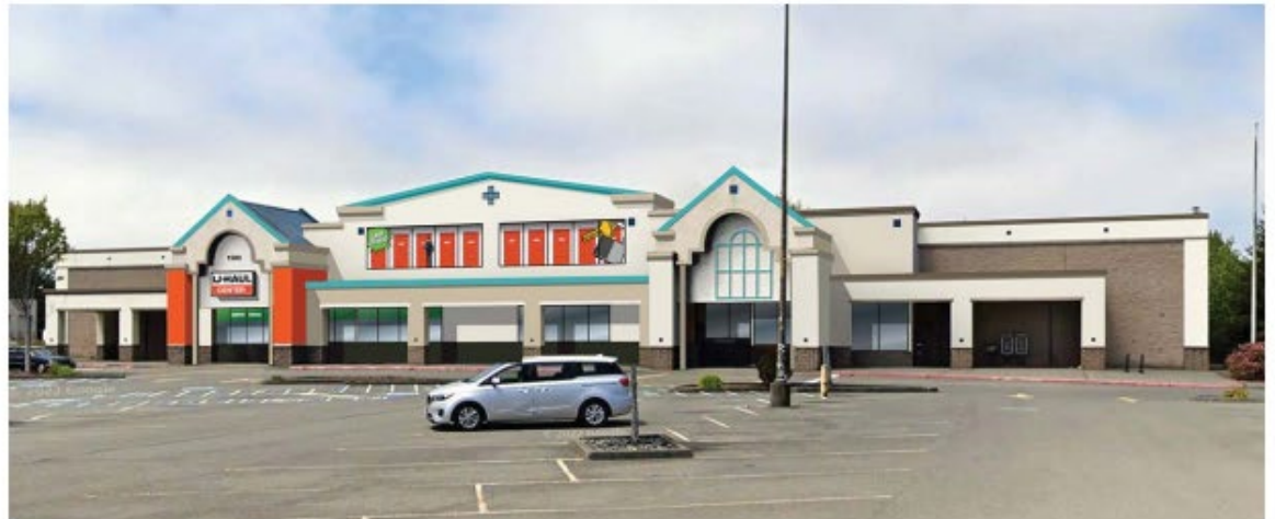
1 East Elevation East Elevation - After
