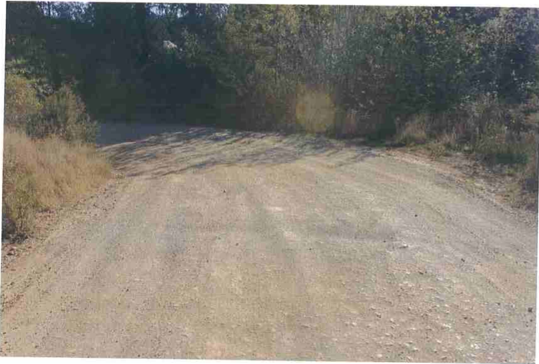
Photo 11. Mile 0.8: 22-ft road width with 1-ft shoulder.
