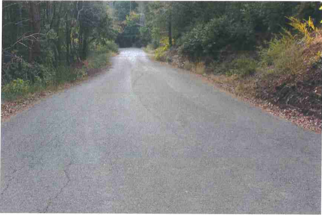
Photo 15. Mile 1.4: 22-ft road width with 1-ft shoulders.
