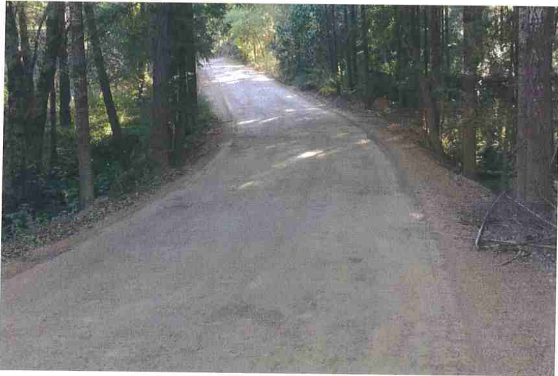
Photo 15. Mile 1.2: 18-ft road width with no shoulder at culvert crossing with decent visibility.
