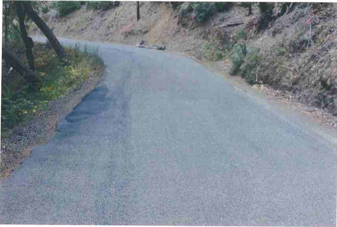
Photo 21. Mile 2.0: 15-ft road width with 1-ft shoulders.
