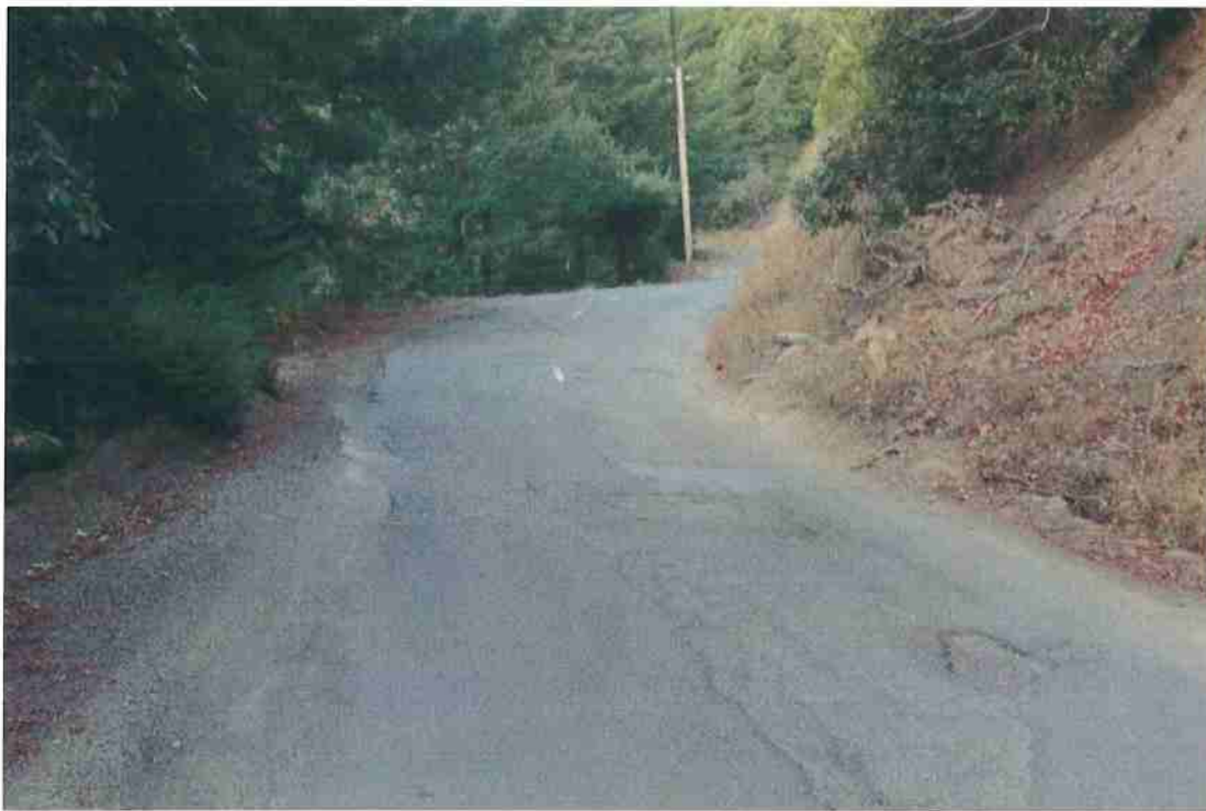
Photo 2. Mile 0.3: Pinch point at recent debris slide and tree; 14' width, no shoulder, blind corner, dangerous spot.
