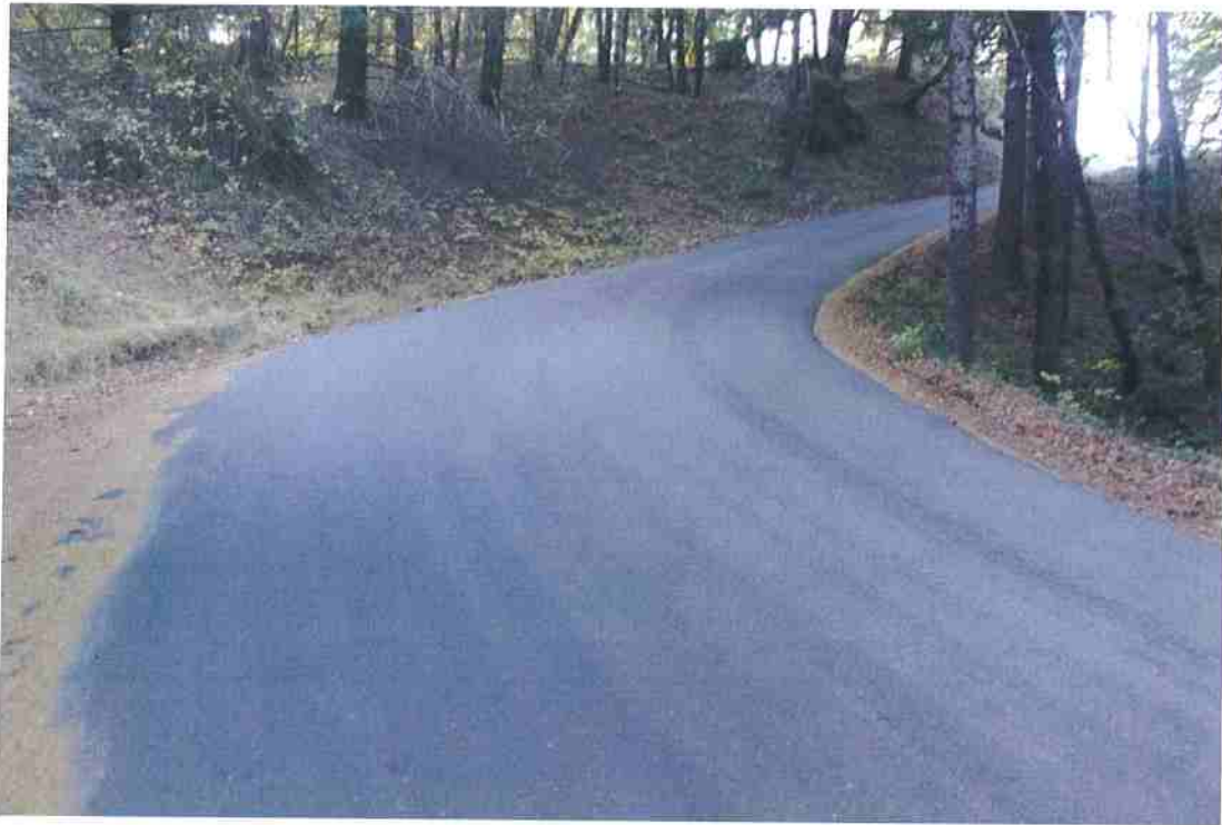
Photo 37. Mile 3.2: 20-ft road width with 2-ft shoulders.
