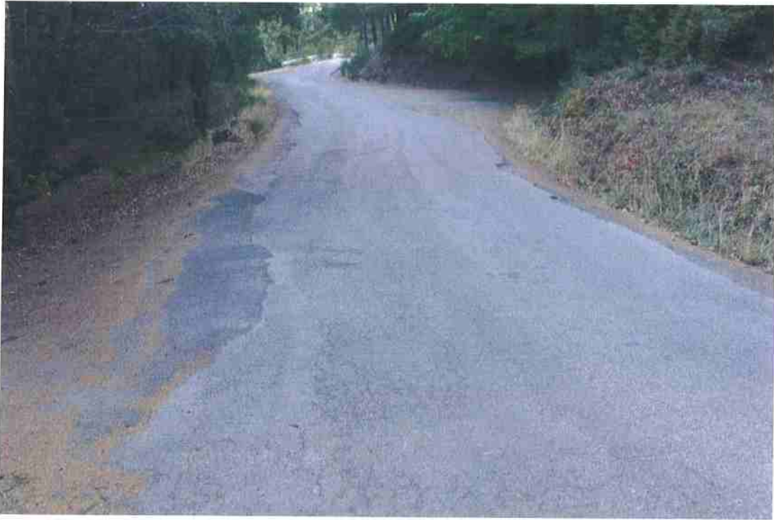
Photo 33. Mile 2.9: 18-ft road width with 1-ft shoulders.
