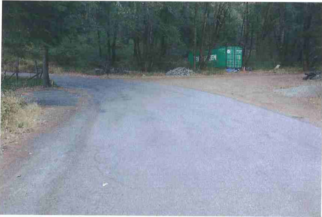
Photo 7. Mile 0.6: 24-ft road width with 2-ft shoulders.
