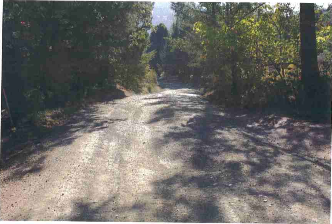
Photo 1. Mile 0.1: 18-ft road width with 1-ft shoulder (begin of segment).
