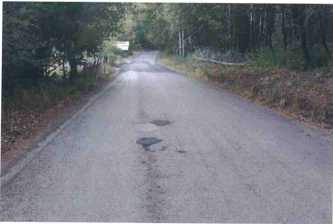
Photo 8. Mile 0.7: 20-ft road width with 2-ft shoulders.
