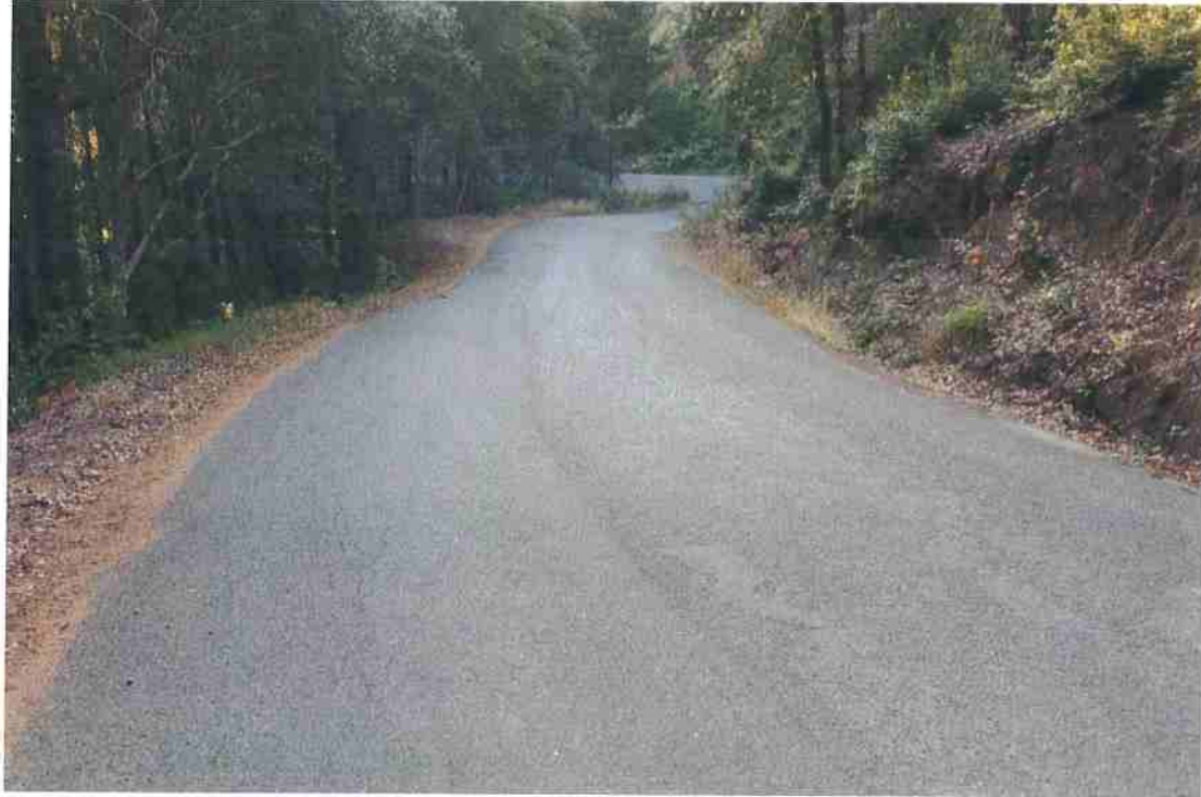
Photo 16. Mile 1.5: 20-ft road width with 1-ft shoulders.
