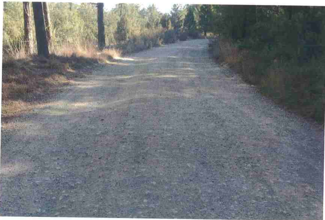
Photo 12. Mile 0.9: 18-ft road width with 1-ft shoulder.
