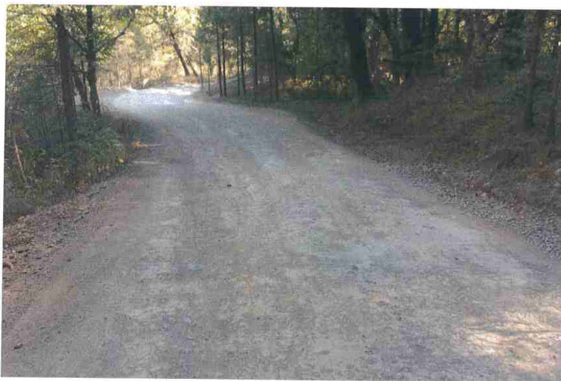
Photo 10. Mile 0.7: 18-ft road width with 1-ft shoulder.
