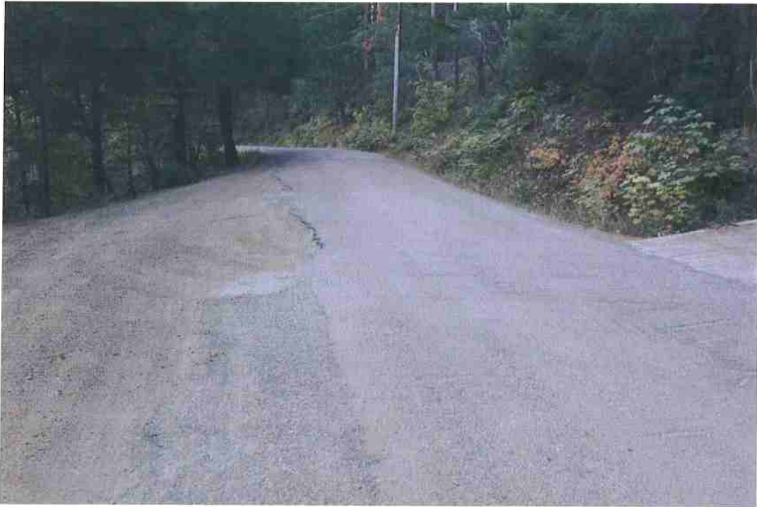
Photo 25. Mile 2.3: 20-ft road width with 2-ft shoulders.
