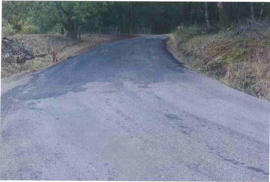
Photo 9. Mile 0.8: 30-ft road width with 1-ft shoulders.
