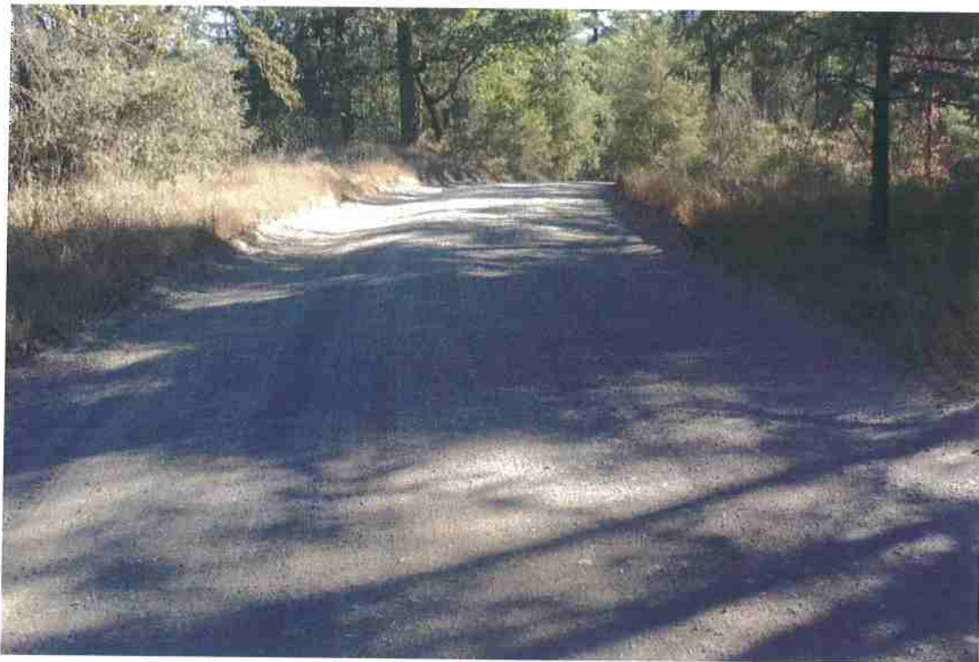
Photo 9. Mile 0.6: 18-ft road width with 1-ft shoulder.
