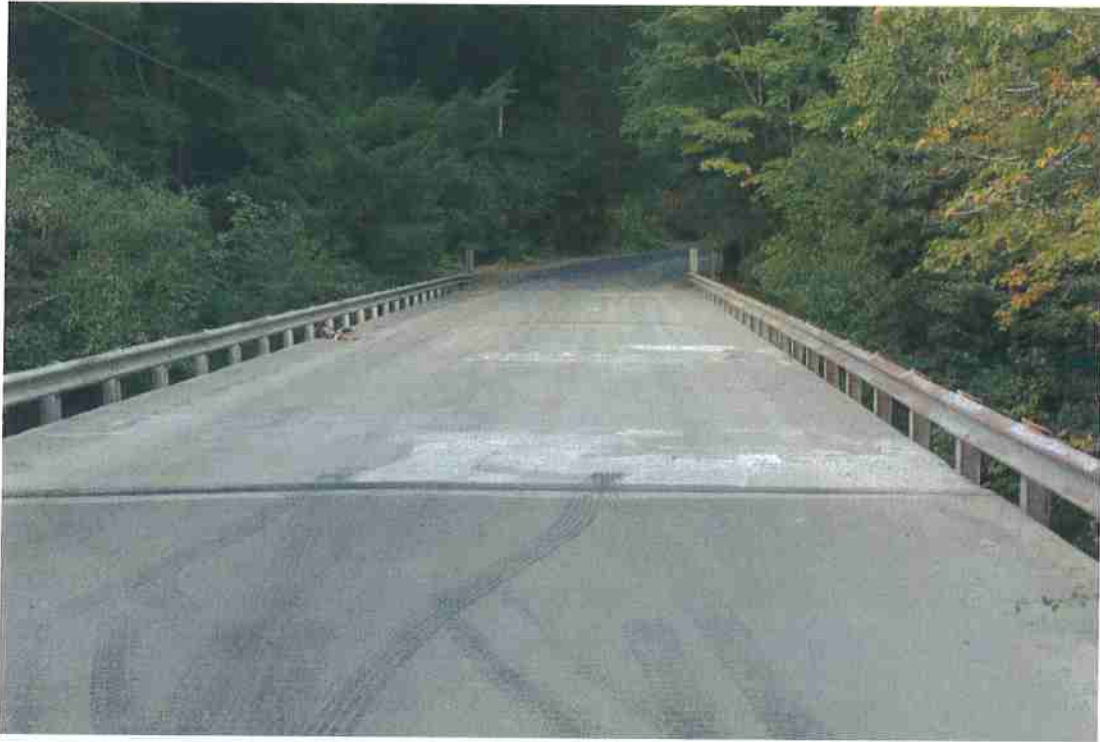
Photo 11. Mile 1.45: 28' width bridge, no shoulders.
