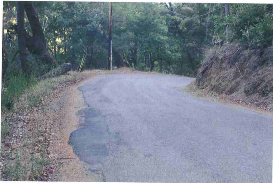
Photo 24. Mile 2.2: 20-ft road width with 1-ft shoulders.
