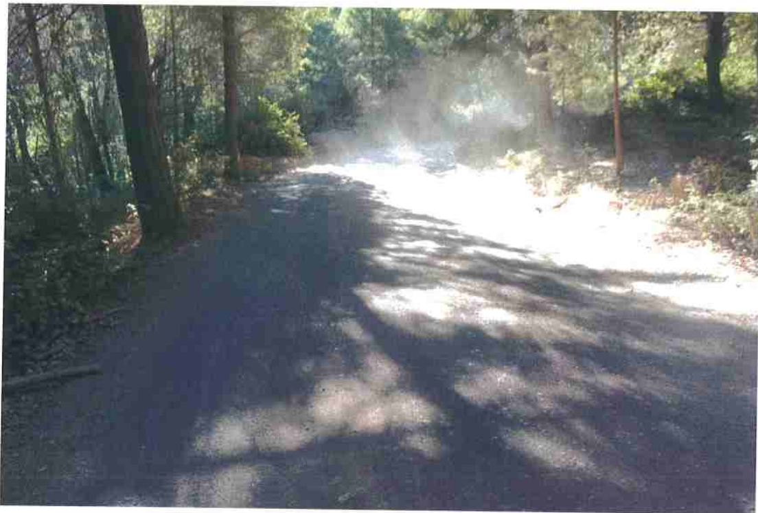
Photo 16. Mile 1.3: 18-ft road width with 2-ft shoulders.
