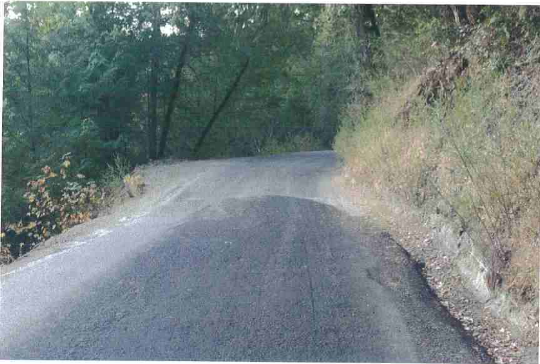
Photo 4. Mile 0.9: relatively narrow section, 15' width, 1' shoulders.
