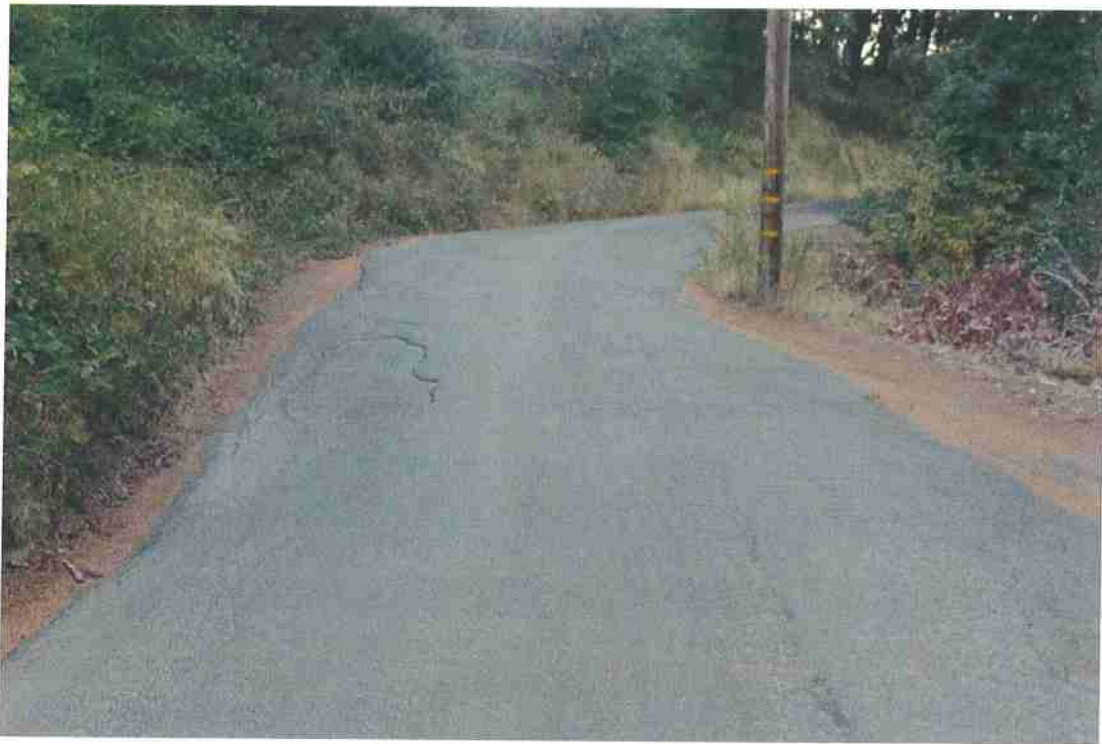
Photo 5. Mile 1.0: 18' width, 1' shoulder.
