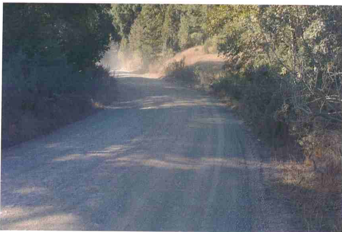
Photo 18. Mile 1.5: 18-ft road width with 1-ft shoulders.
