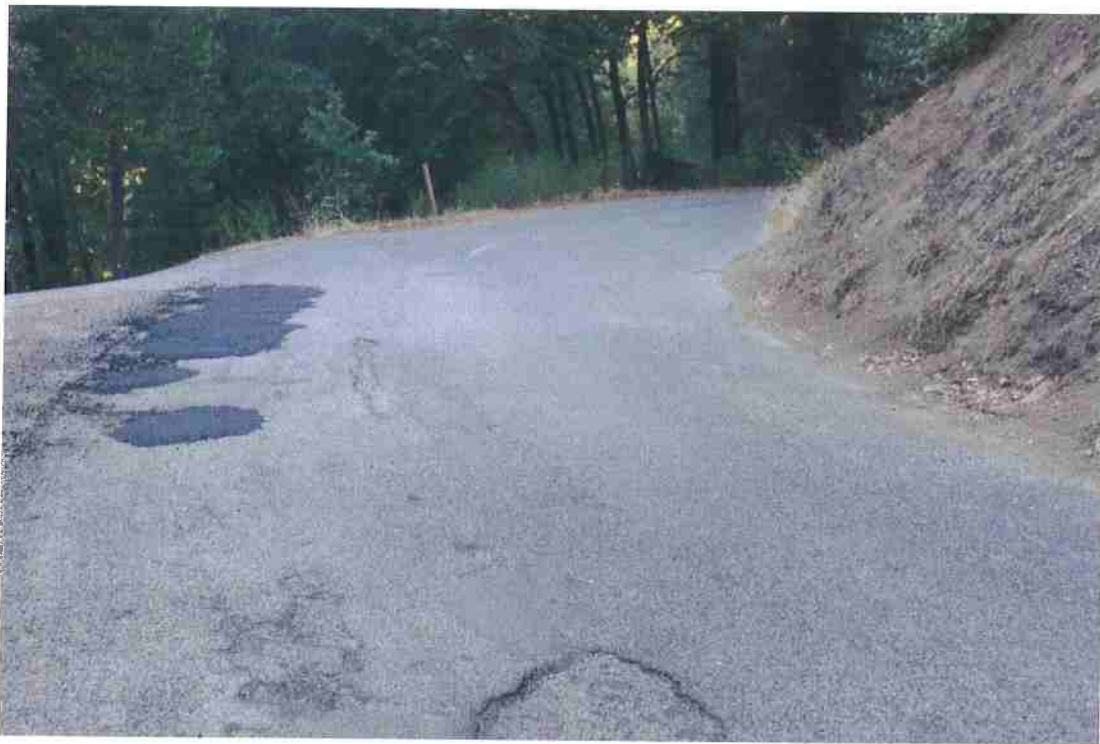
Photo 20. Mile 1.9: 18-ft road width with 2-ft shoulders.
