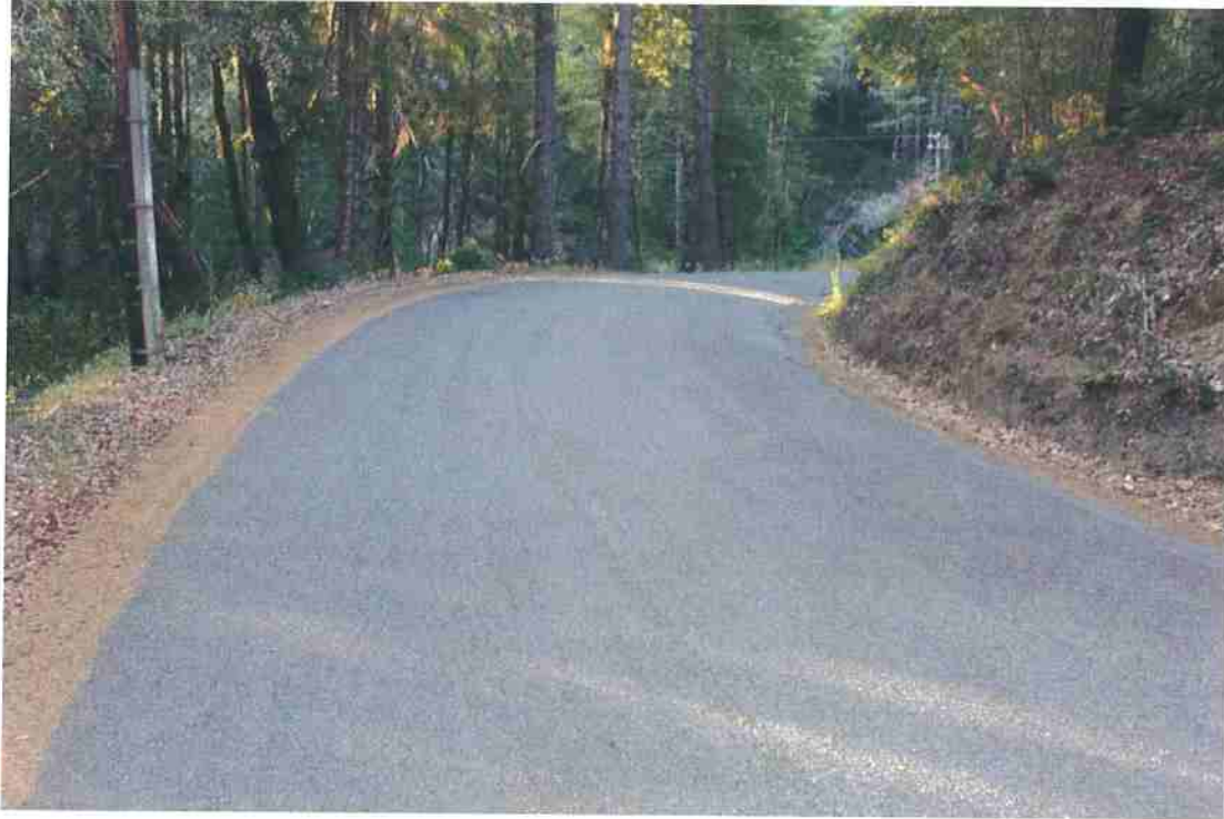
Photo 18. Mile 1.7: 20-ft road width with 1-ft shoulders.
