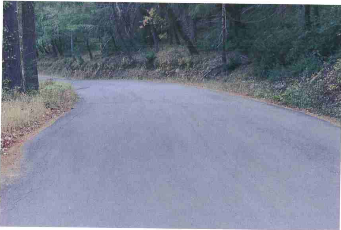
Photo 12. Mile 1.1: 20-ft road width with 2-ft shoulders.
