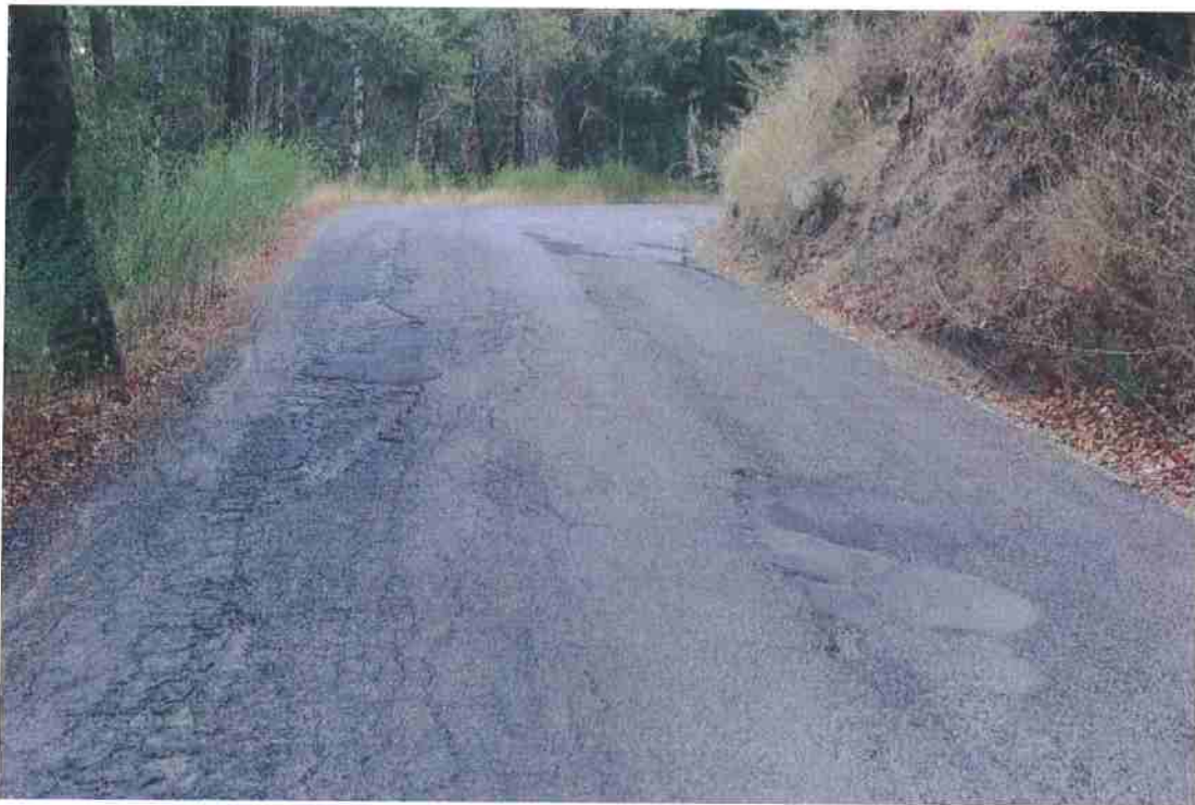
Photo 6. Mile 0.5: 18-ft road width with 1-ft shoulders.
