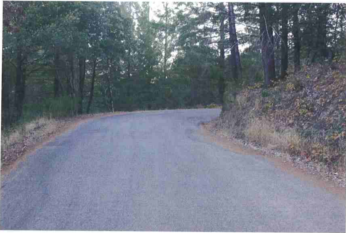
Photo 13. Mile 1.2: 20-ft road width with 1-ft shoulders.
