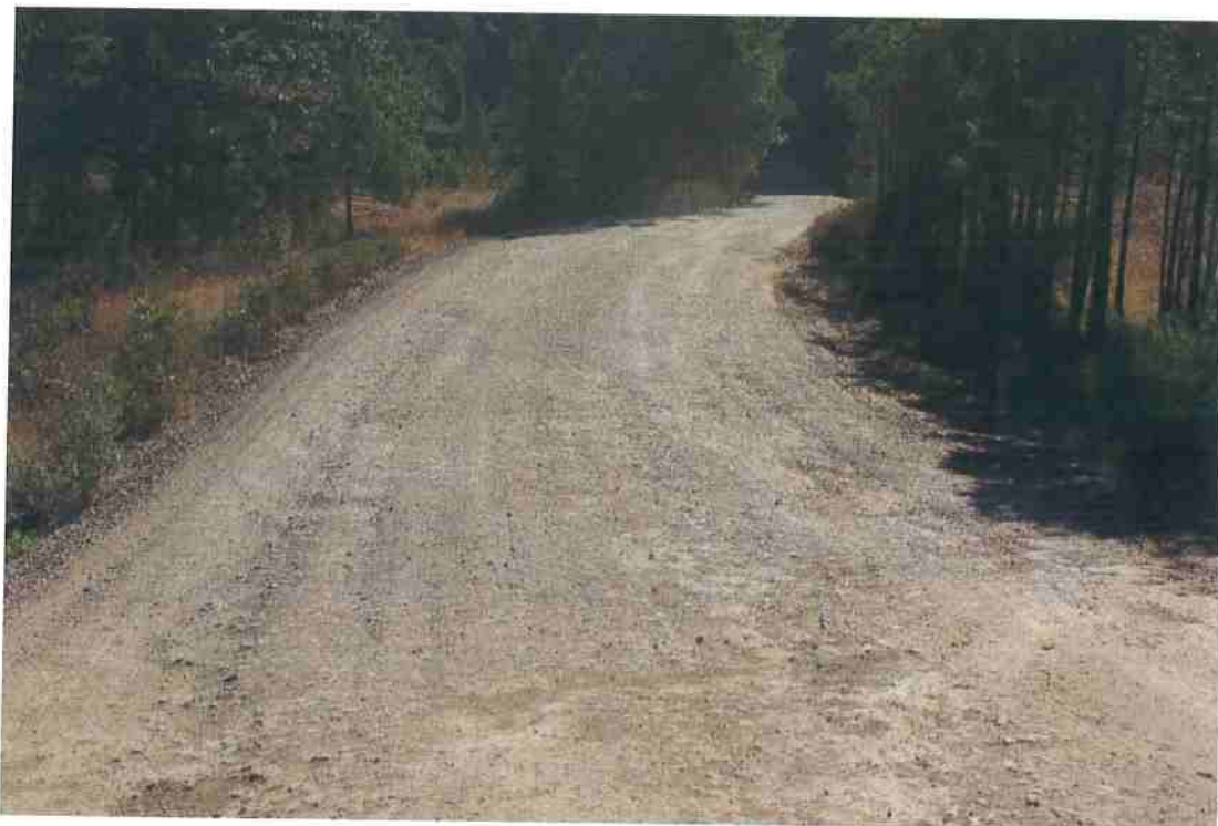
Photo 7. Mile 0.5: 18-ft road width with 1-ft shoulder.
