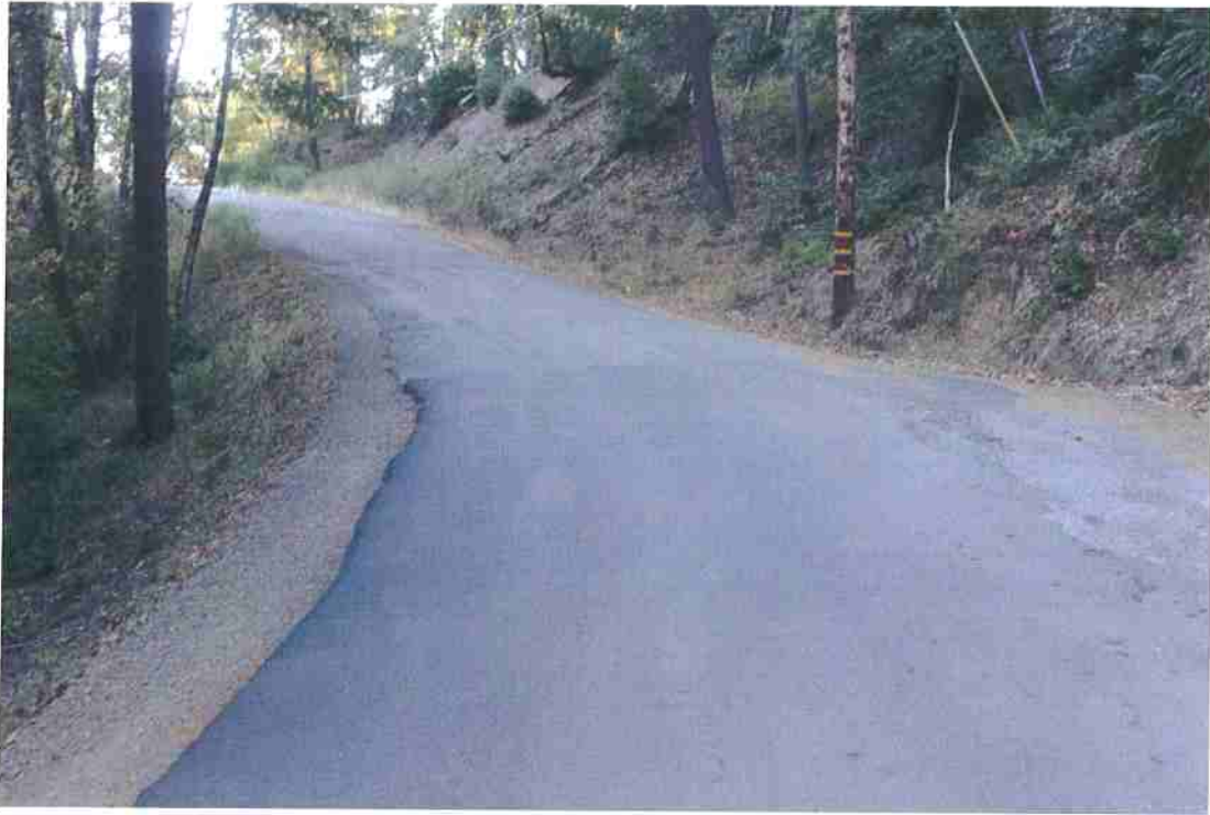
Photo 29. Mile 2.5: 18-ft road width with 2-ft shoulders.
