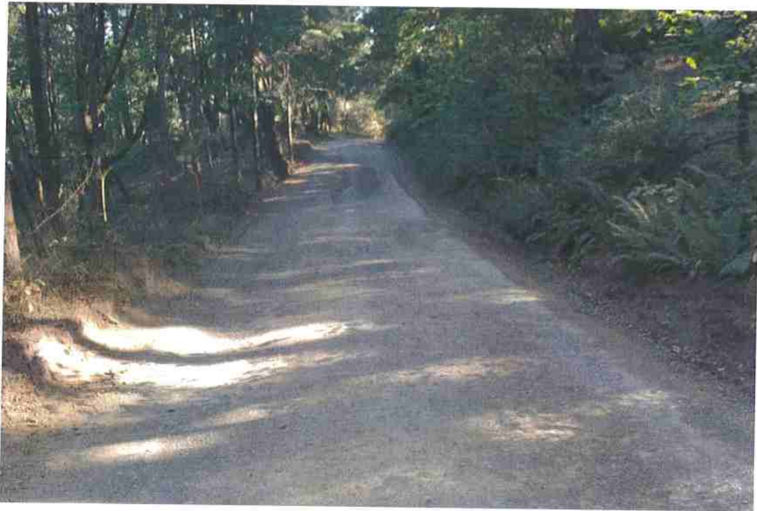
Photo 14. Mile 1.1: 18-ft road width with 2-ft shoulder; OK visibility.
