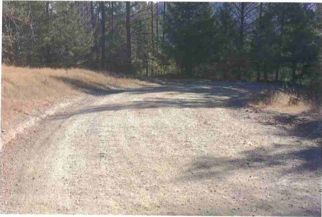
Photo 3. Mile 0.3: 20-ft road width with 2-ft shoulder.
