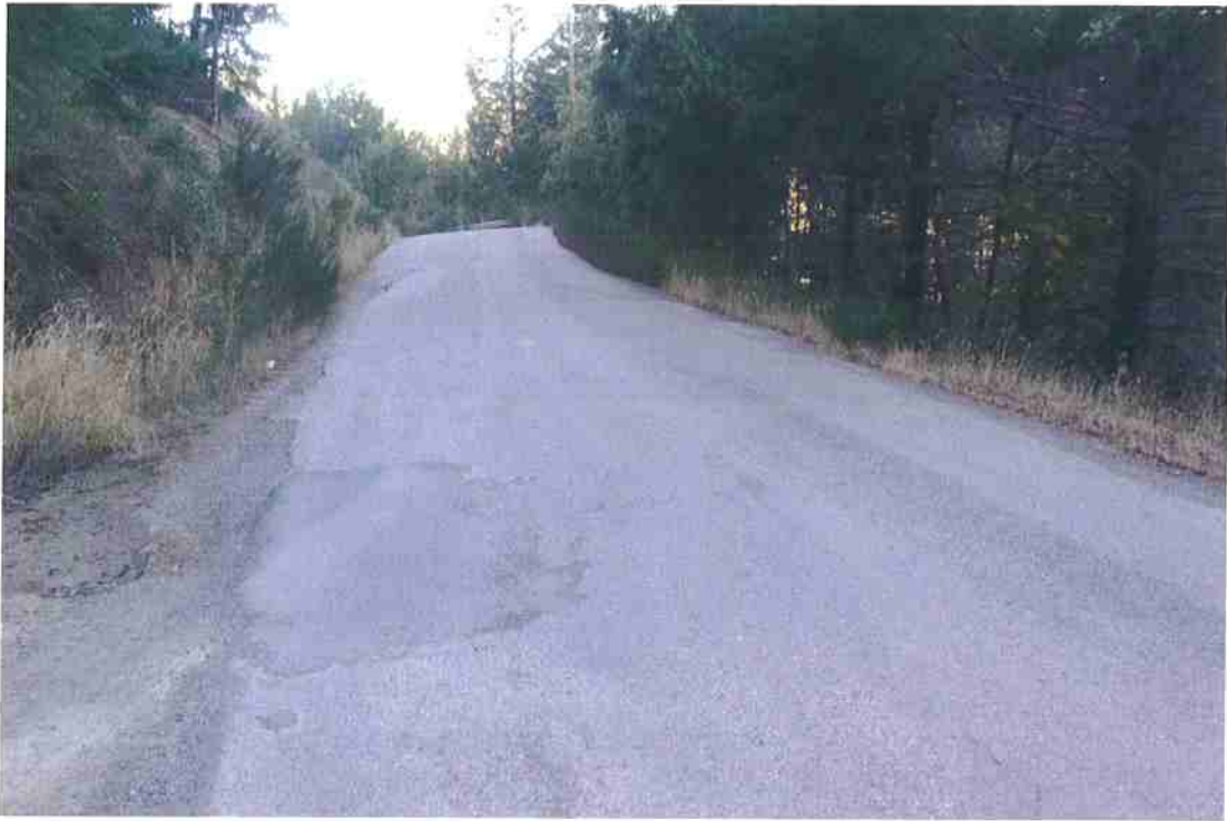
Photo 31. Mile 2.7: 20-ft road width with 2-ft shoulders.
