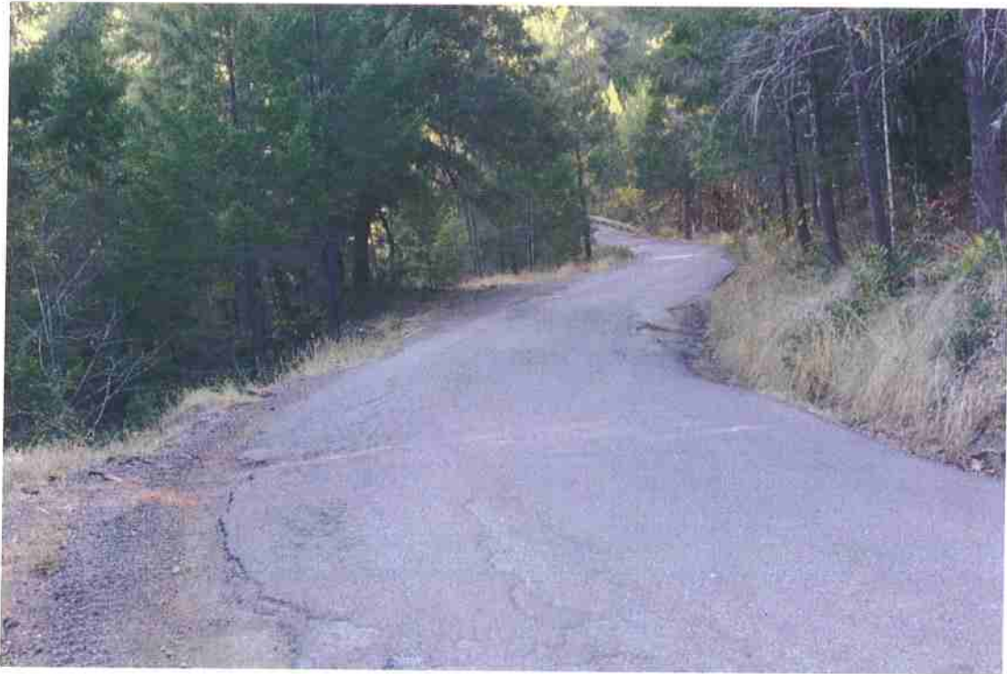
Photo 39. Mile 3.4: 16-ft road width with 1-ft shoulder. Pinch point at downgradient extent of blind corner. Potential spot to widen corner on inside to improve width and visibility.
