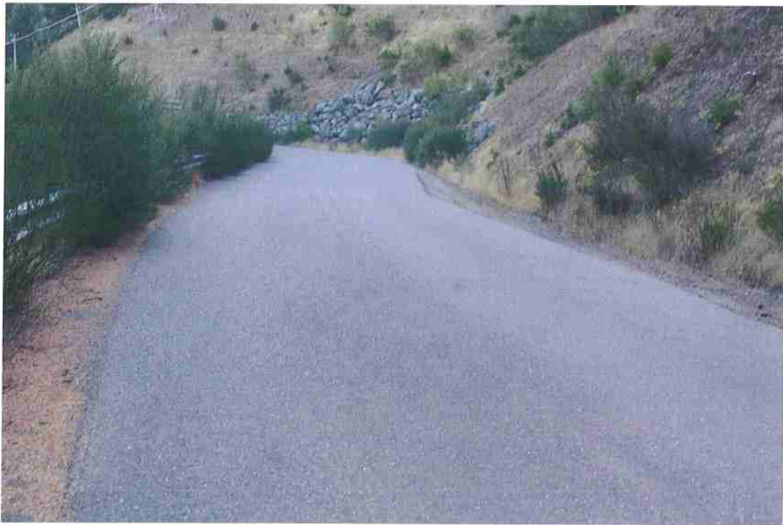
Photo 32. Mile 2.8: 18-ft road width with 1-ft shoulders.
