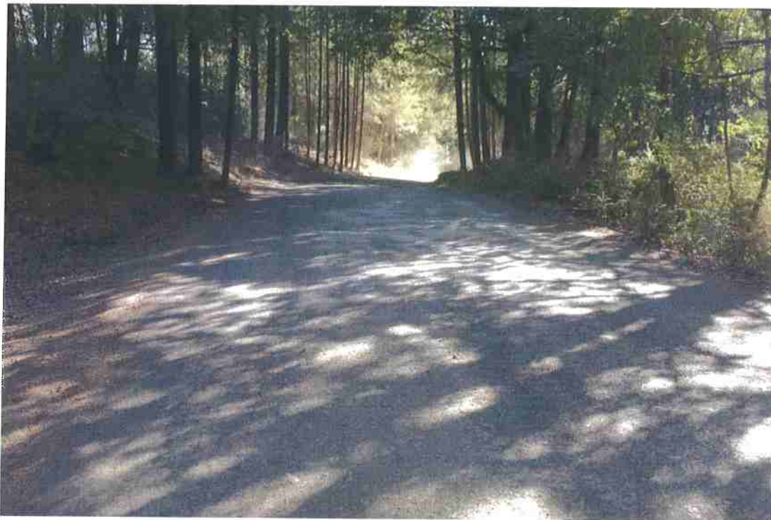
Photo 17. Mile 1.4: 20-ft road width with 2-ft shoulder.
