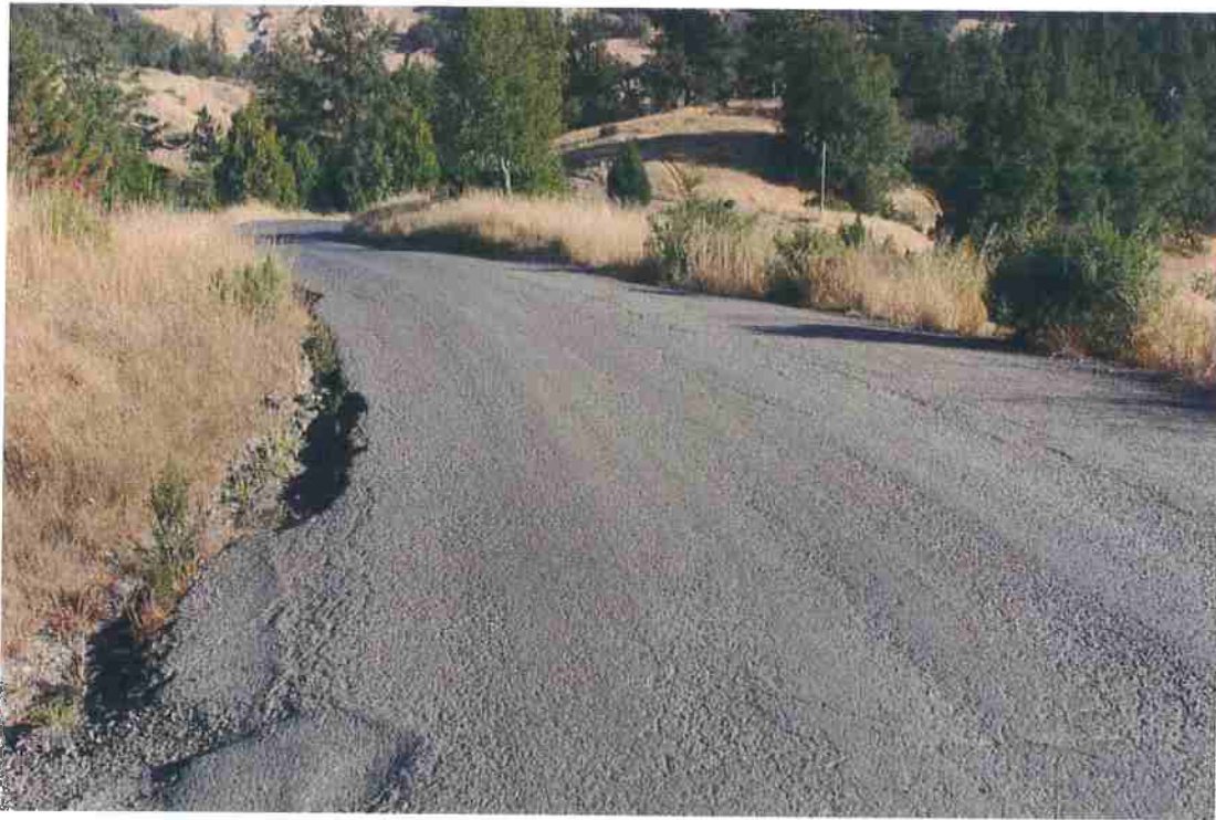
Photo 44. Mile 3.8: 18-ft road width with 1-ft shoulders.
