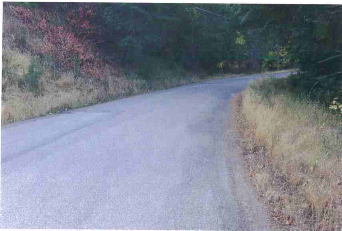
Photo 14. Mile 1.3: 22-ft road width with 2-ft shoulders.
