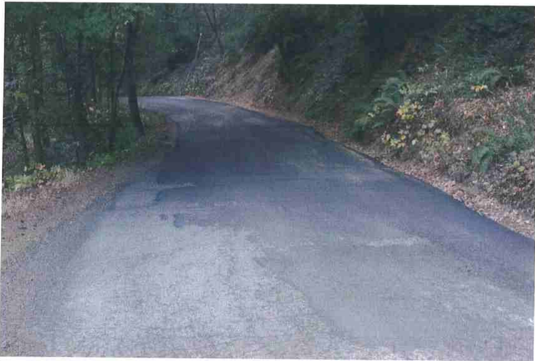
Photo 3. Mile 0.3: 18-ft road width with 1-ft shoulders.
