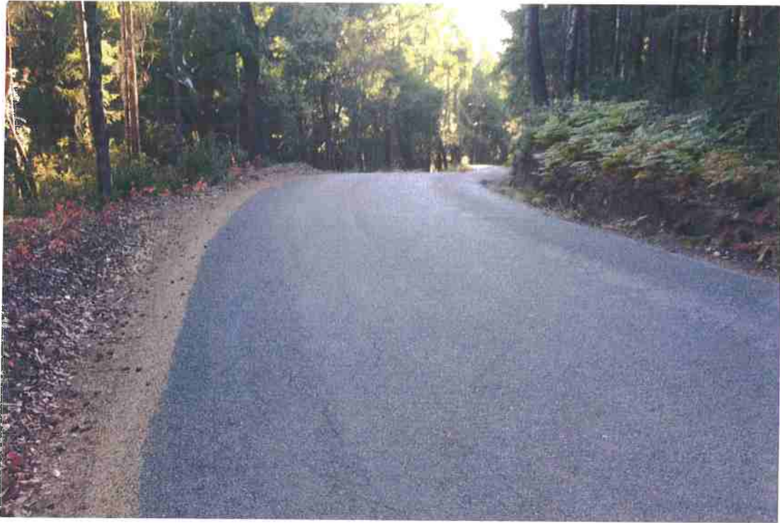
Photo 17. Mile 1.6: 20-ft road width with 2-ft shoulders.
