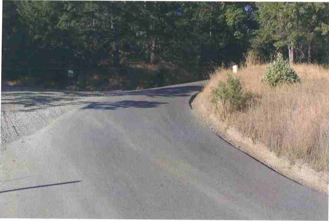
Photo 45. Mile 3.85: Blind corner at intersection with Lower Thomas Road. 16-ft road width with 1-ft shoulders. Potential location to widen corner on inside to improve visibility.
