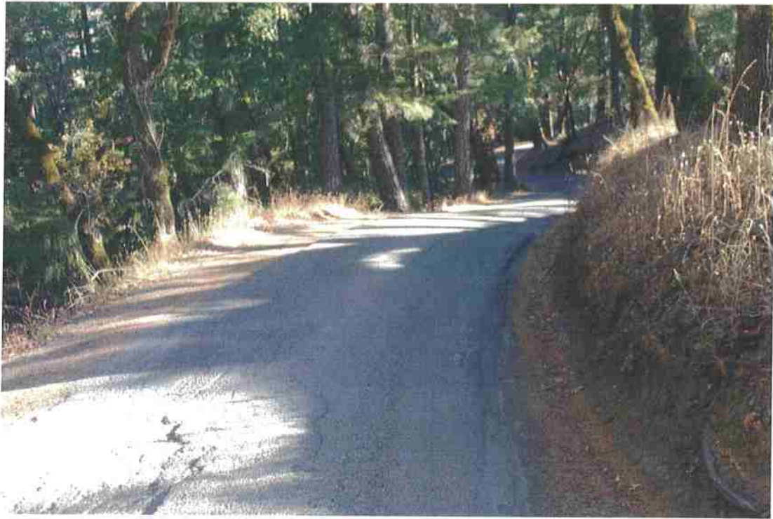
Photo 41. Mile 3.6: 12-ft road width with 2-ft shoulders. Pinch point but decent visibility with turnouts.
