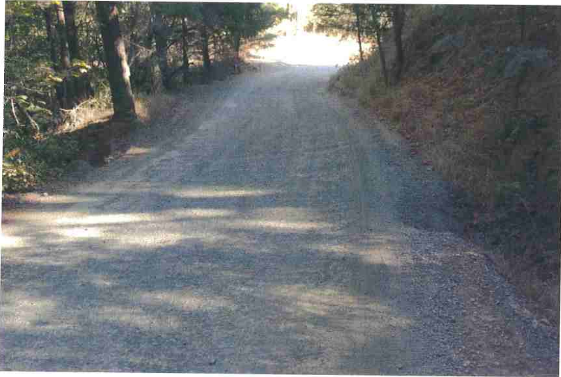
Photo 5. Mile 0.35: Pinch point at culvert; 16-ft road width with no shoulder and partial blind corner.
