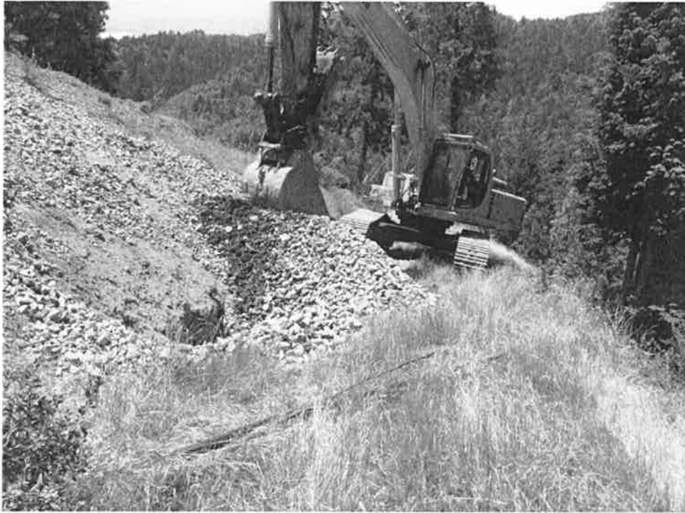
Photo 1: Excavating dry well
