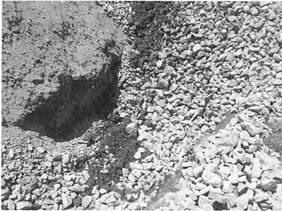
Photo 3: Moist soil at depth of 5 feet
