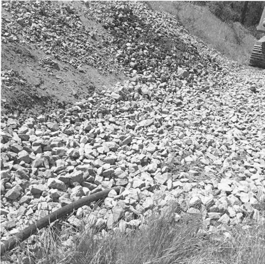
Photo 9: Completed pipe underground
