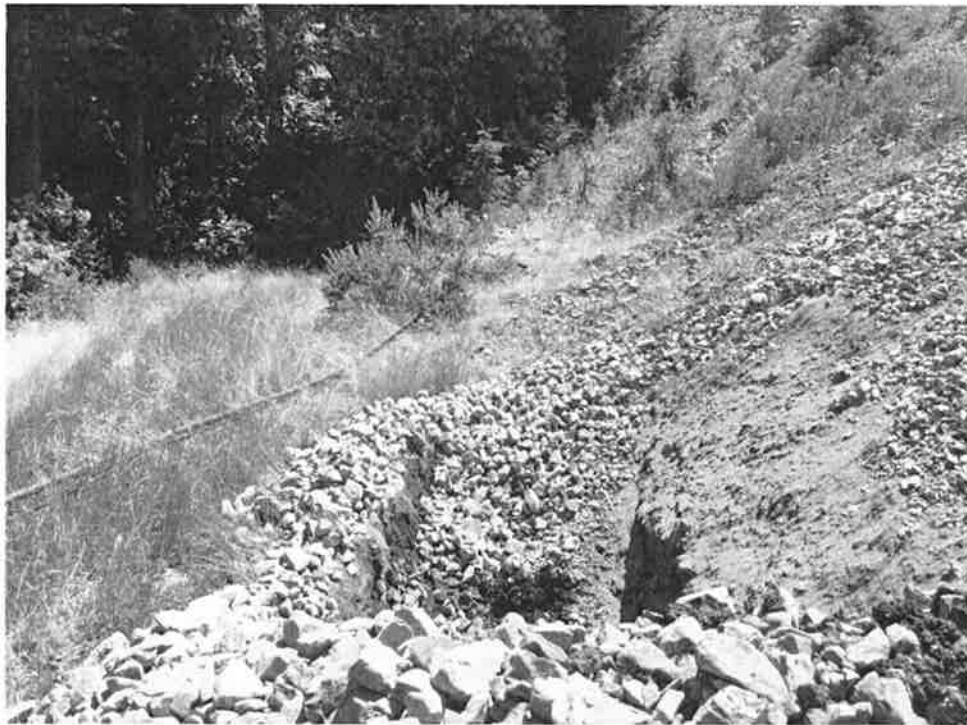
Photo 2: Excavation before pipe placement
