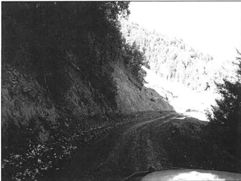
Cut bank along haul road showing full extent of serpentinite
