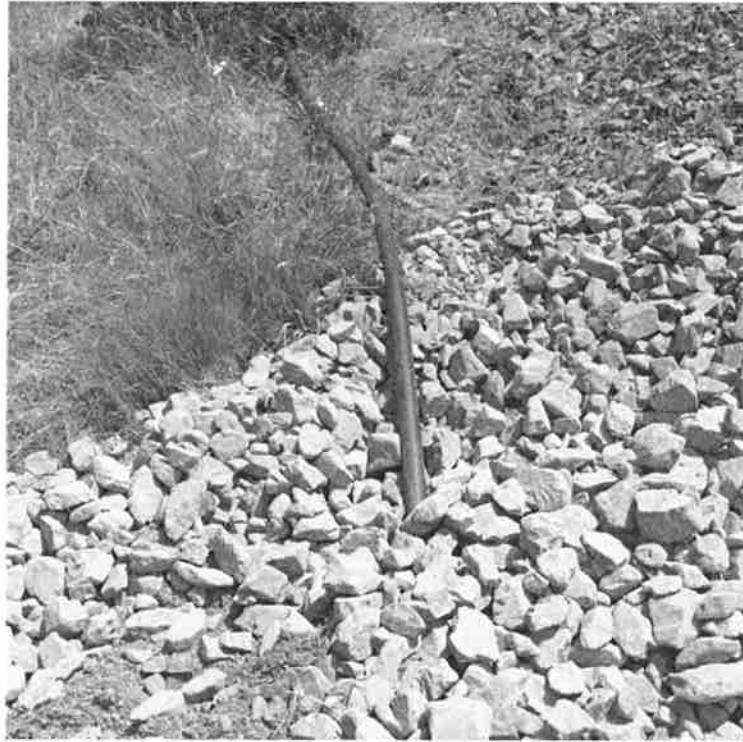
Photo 7: Completed pipe installation
