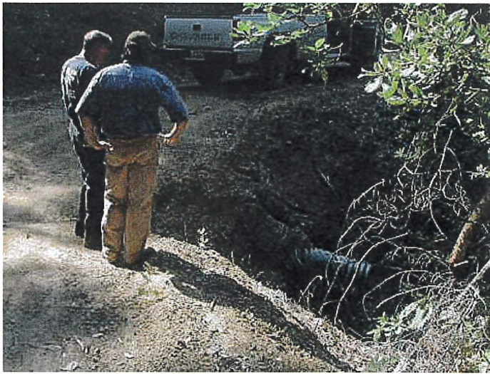
Figure 14. This fill slope erosion was caused by a plugged cross-drain inlet that diverted ditch flow over the road surface. Photo: Angela Wilson, Central Valley Regional Water Quality Control Board.
