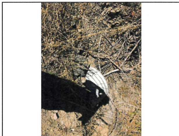
Photo #179 River Rd Looking @ Partially Clogged 36" Culvert In
