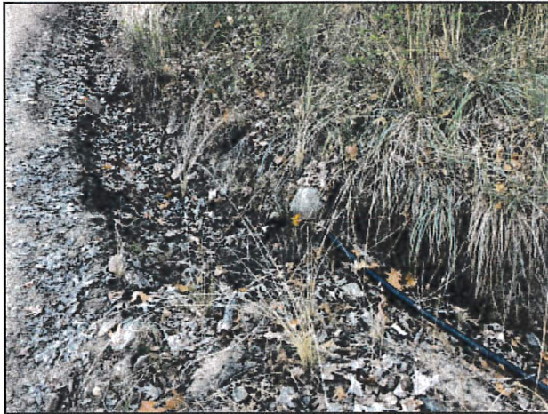
Photo #526 Private Access Rd APN 208-231-012 Looking @ Partially Clogged Culvert Out
