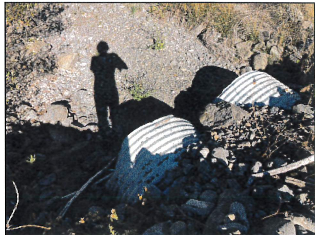
Photo #16 River Rd Looking @ Dual 36" Culverts Out
