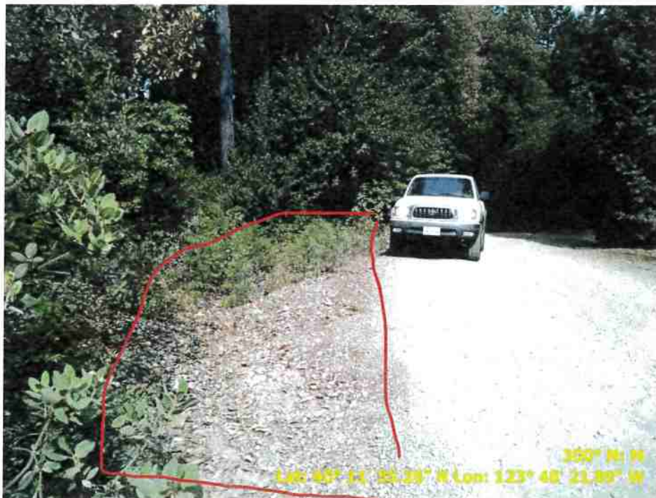
Figure 28. Photo showing a pullout that needs to be regraded and vegetation cleared.
