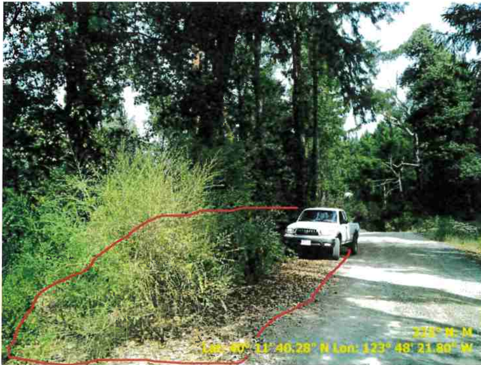
Figure 26. Photo of Road Point 94 showing a pullout that needs to be regraded and vegetation cleared.
