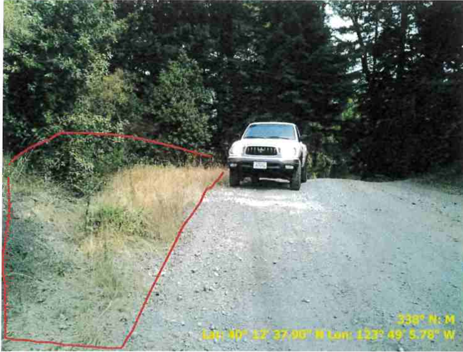
Figure 11. Photograph showing Road Point 40 which is a pullout that need to be regraded.
