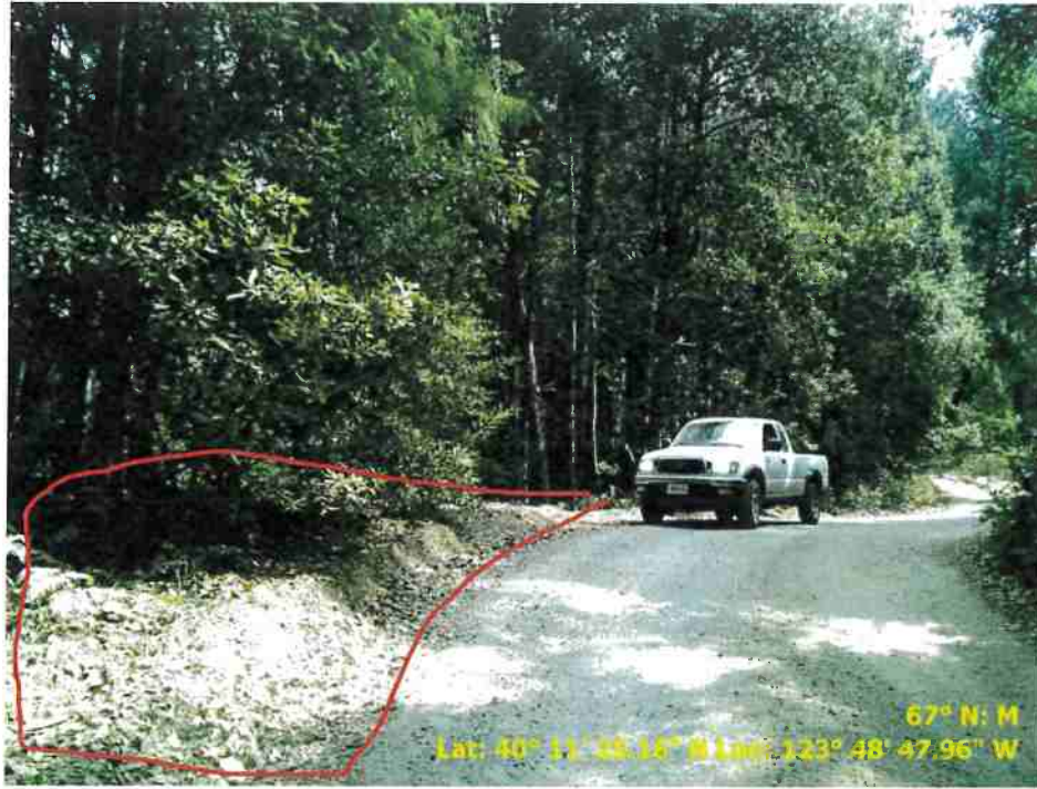
Figure 37. Photo of Road Point 119 showing a pullout that needs to be cleared of vegetation and regrading.
