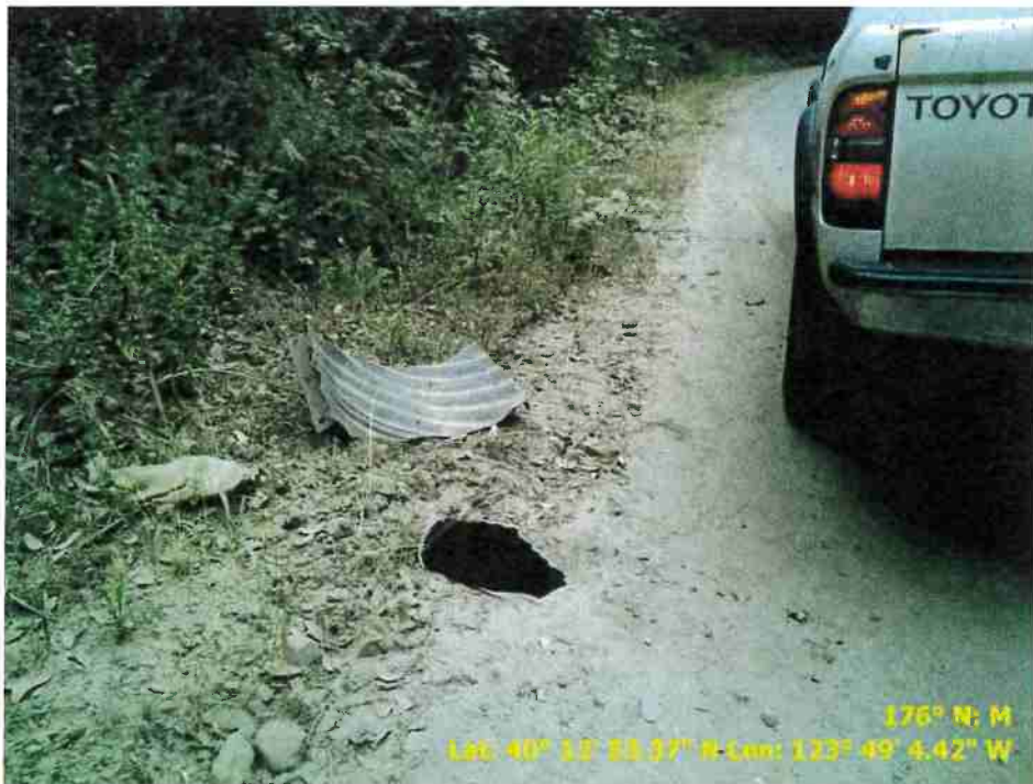
Figure 6. Road point 15 shows an 18" drainage relief culvert with an exposed opening that needs to be repaired or replaced.
