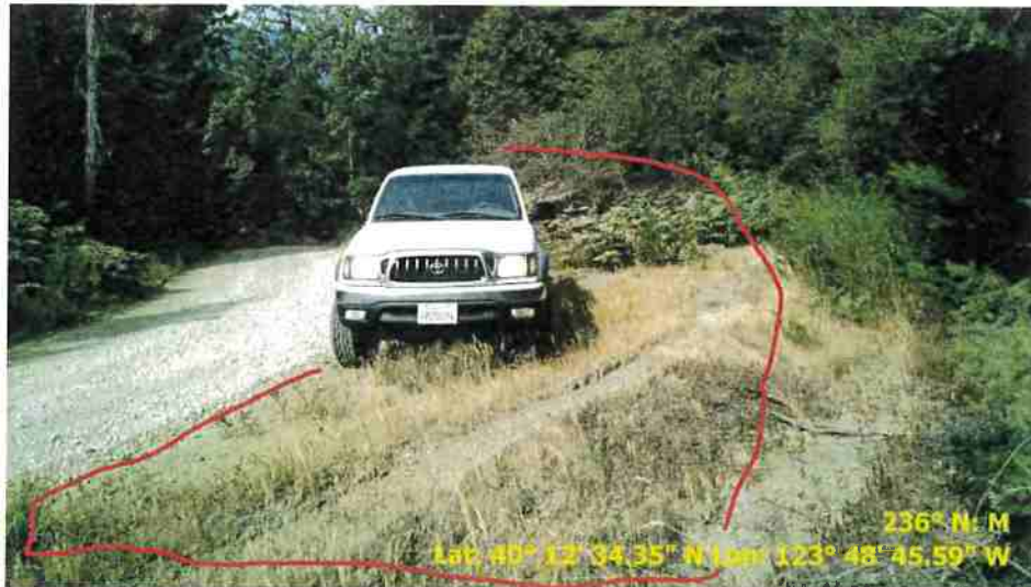
Figure 13. Photograph showing Road Point 64 which is a pullout that needs to be regraded to make room for larger vehicles.
