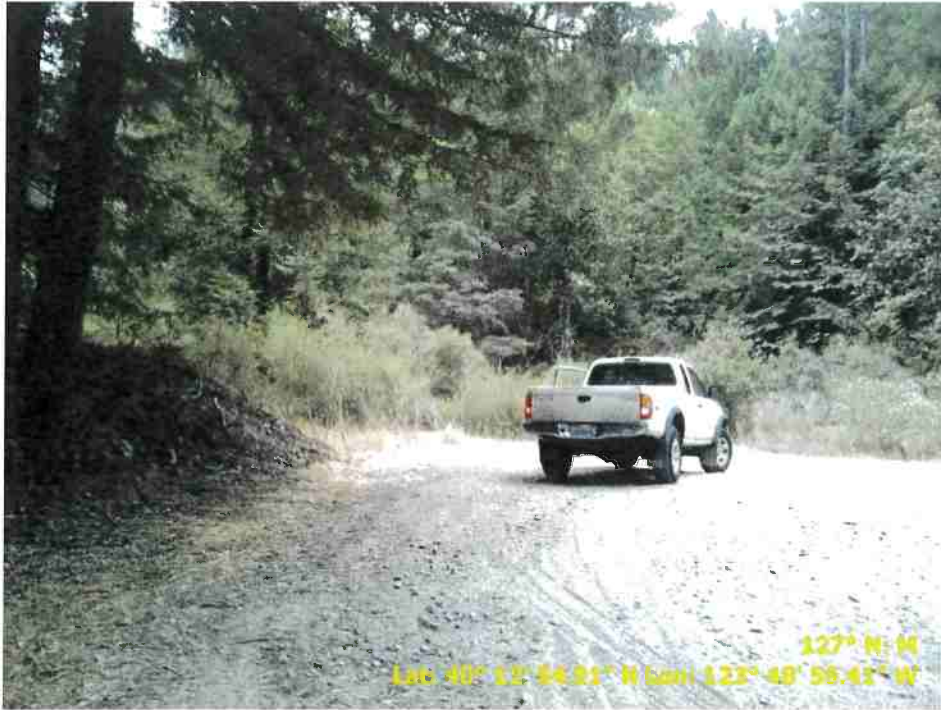
Figure 5. Photograph showing Road Point 24 which is a pullout that shall be maintained as a pullout.
