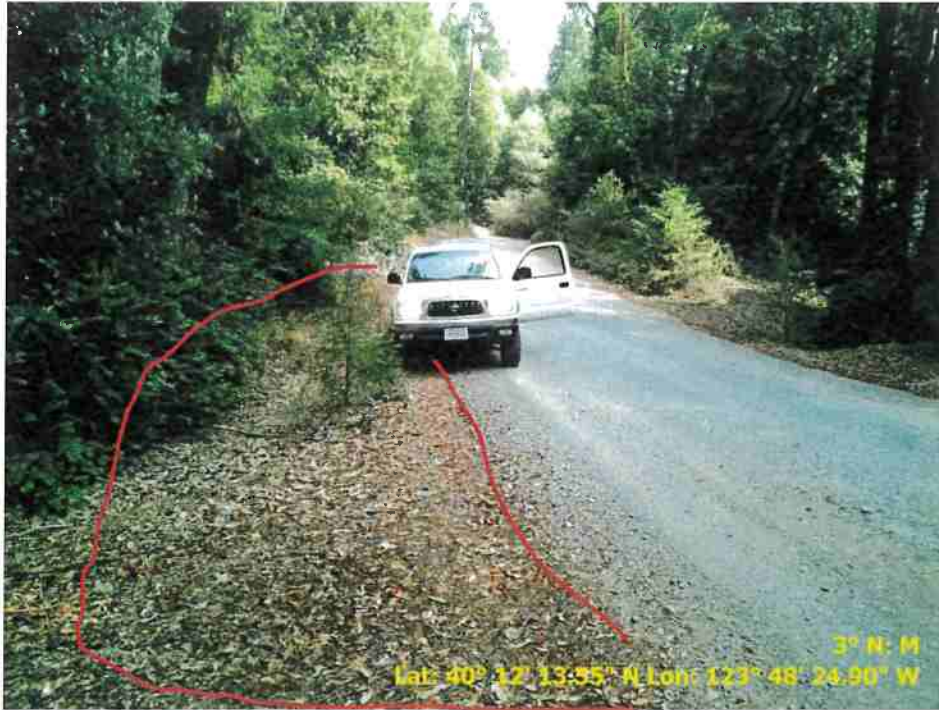
Figure 19. Photo of Road Point 79 showing a pullout that needs to be regraded and vegetation cleared.
