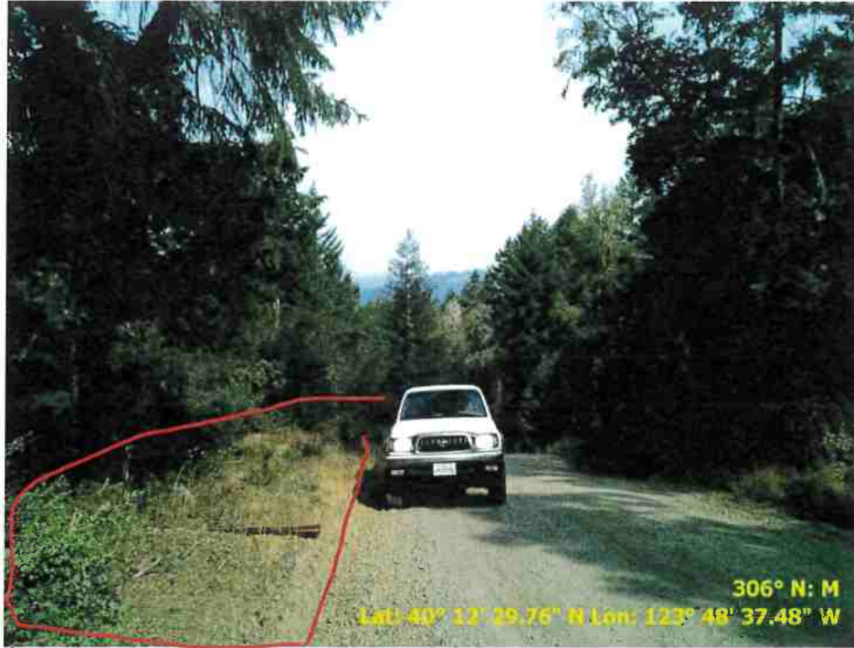
Figure 15. Photo of Road Point 71 showing a pullout that needs to be regraded.
