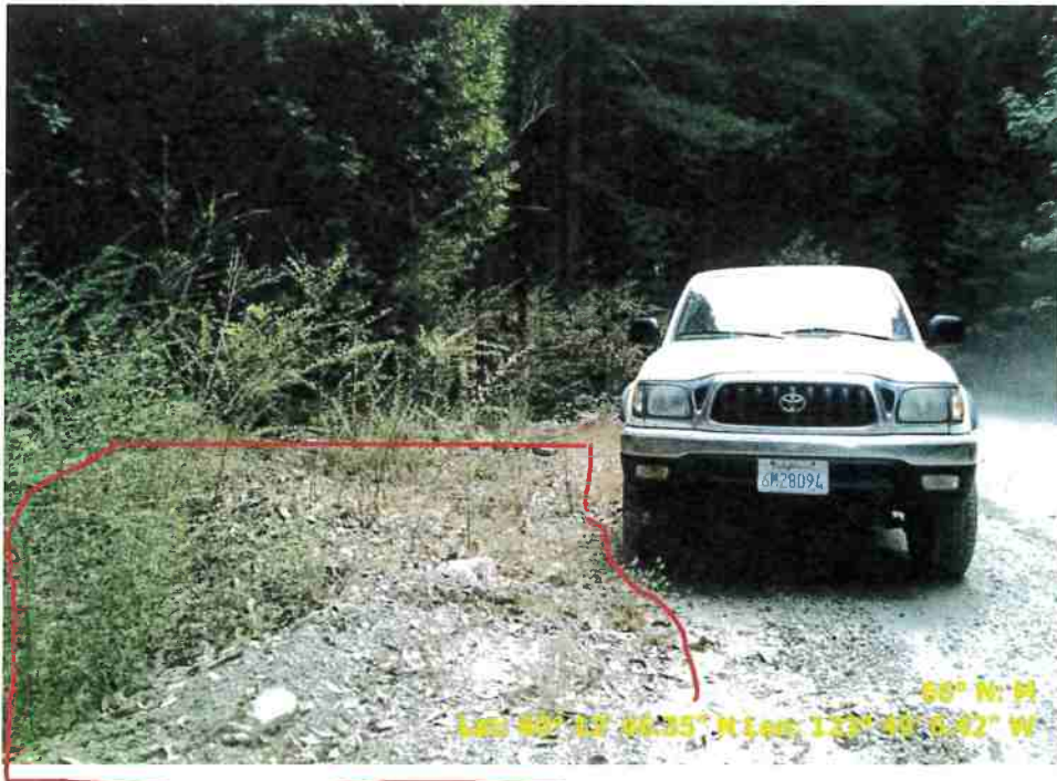
Figure 9. Photograph showing Road Point 27 which is a pullout that need to be regraded.
