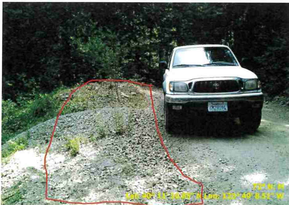
Figure 41. Photo of Road Point 133 showing a pullout that needs to be cleared of vegetation and to be regraded.
