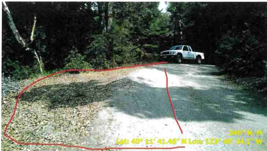
Figure 30. Photo of Road Point 103 showing a pullout that needs to be regraded.
