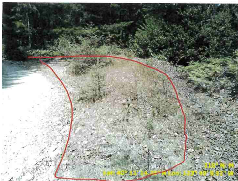
Figure 43. Photo of Road Point 301 showing water-bar/rolling dip that needs surface rock..
