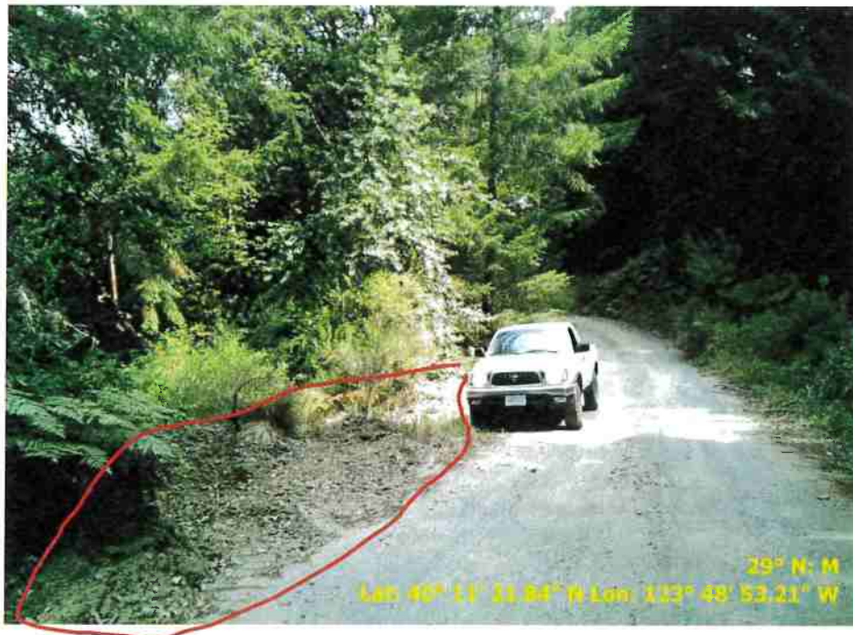
Figure 38. Photo of Road Point 123 showing a pullout that needs to be cleared of vegetation and regrading.
