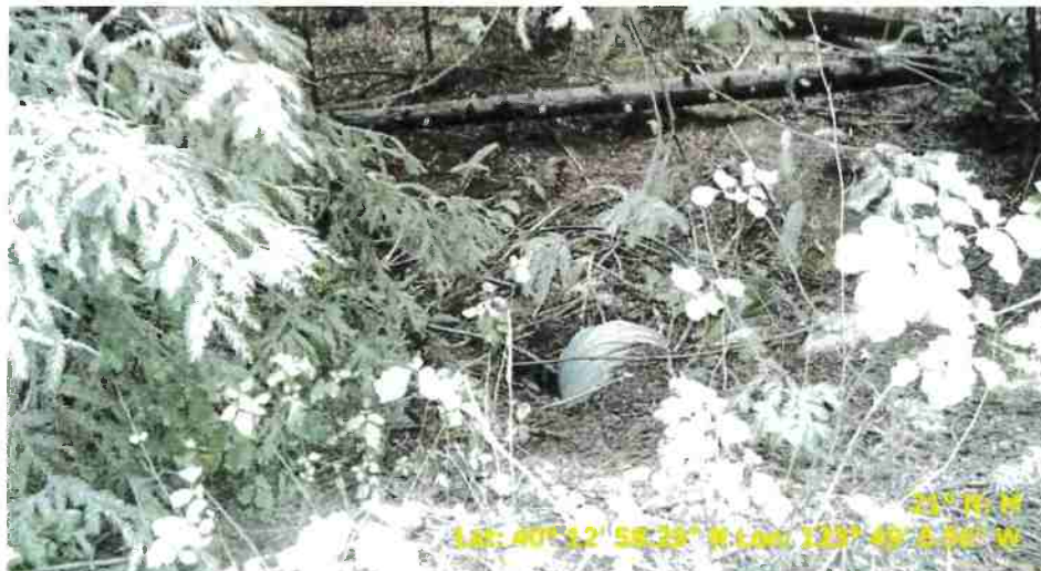
Figure 4. Road point 58 showing an 18-inch drainage relief culvert that is in good condition.
