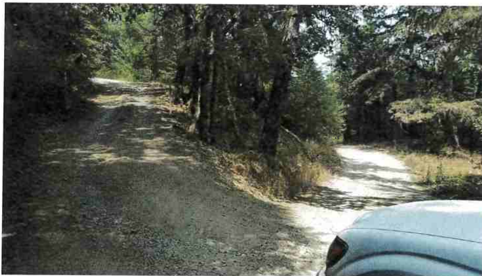
Figure 50. Road Point 202 Shows the gate at intersection of access Road 4 and the off property driveway that leads to Project 2. The start of the driveway has a slope that is approximately 18%.
