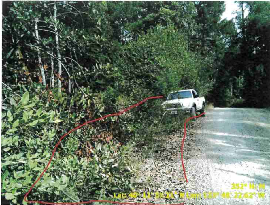
Figure 27. Photo of Road Point 91 showing a pullout that needs vegetation cleared and to be regraded.
