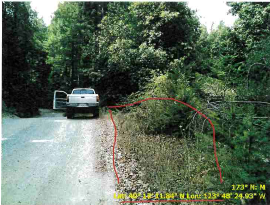
Figure 20. Photo of Road Point 80 showing a pullout that needs to be regraded and vegetation cleared.
