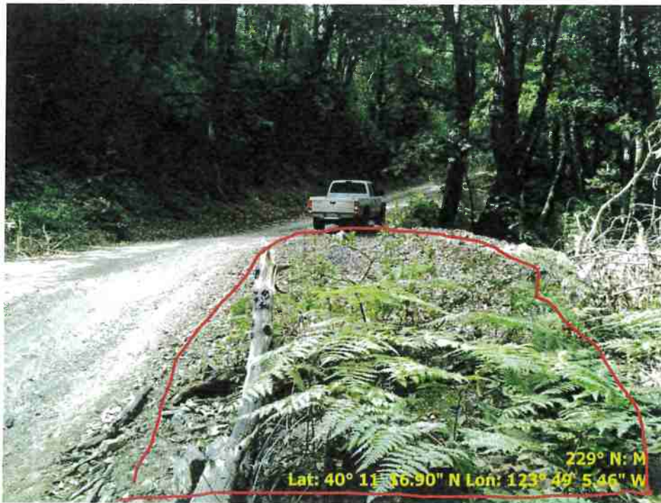
Figure 41. Photo of Road Point 133 showing a pullout that needs to be cleared of vegetation and to be regraded.
