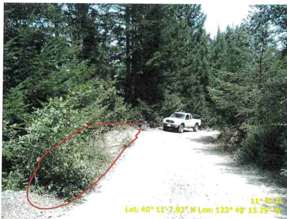
Figure 47. Photo of Road Point 150 showing a pullout that needs to be cleared of vegetation and regraded.
