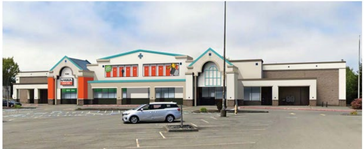
1 East Elevation East Elevation - After
