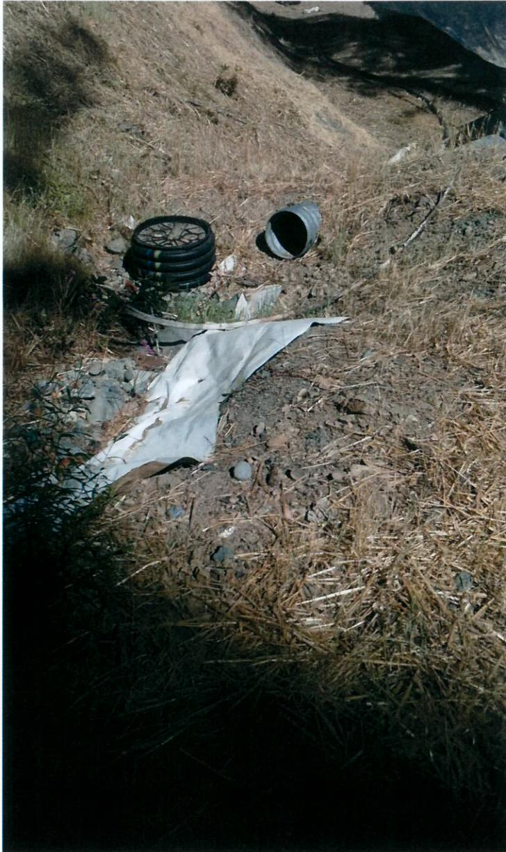
Picture 8: This is a picture of the rain catchment and the cistern that are used to fill the pond during winter. The cistern is the vertical plastic culvert in the frame. It collects drainage from a cut bank seep that is out of the frame to left. It was dry on the photo date. The 12 inch metal culvert is used to collect rain water and divert it into the pond. Photo date 9/16/2016
