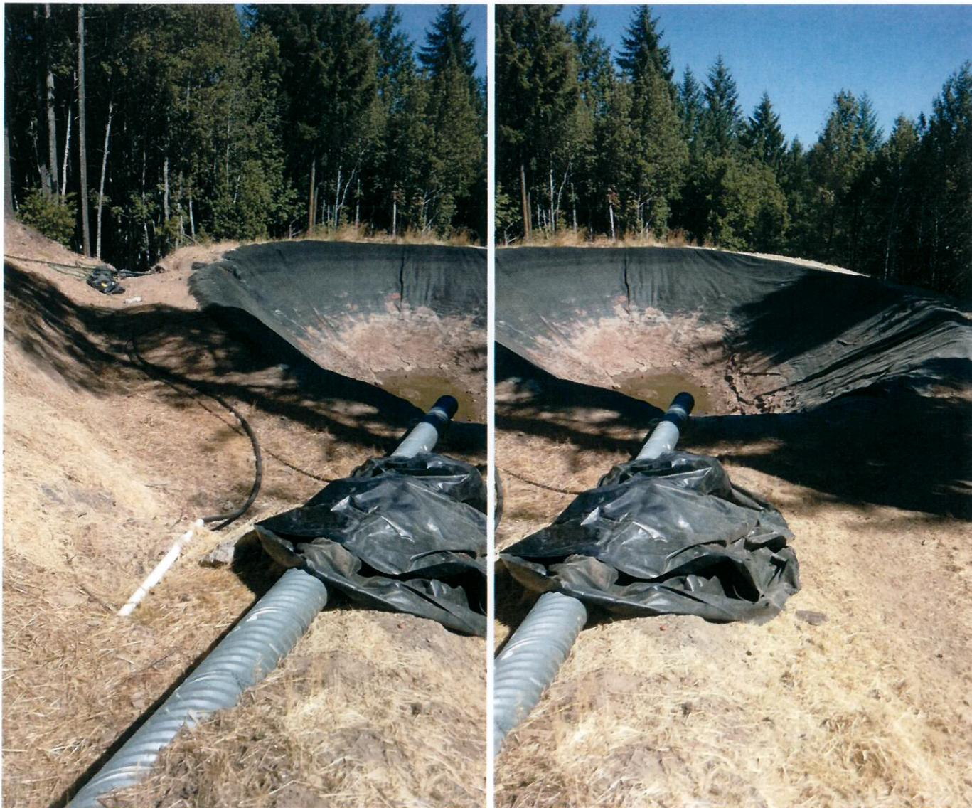
Pictures 6 and 7: These are pictures of the pond. The one inch plastic waterline in the picture on the left is attached to the cut bank seep / cistern. The waterline can be directed into the pond or taken out and directed towards the rock lined ditch as it is in the picture. Photo date 9/16/2016
