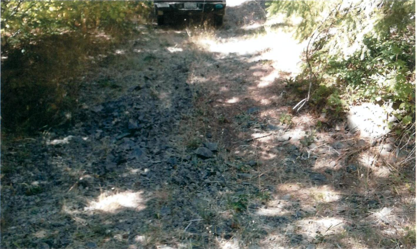
Picture 4: This is a picture of the rocked ford Class III watercourse crossing at Map Point 2. The rocked ford Class III watercourse crossings at Map Points 3 and 5 are very similar. Photo date 9/16/2016
