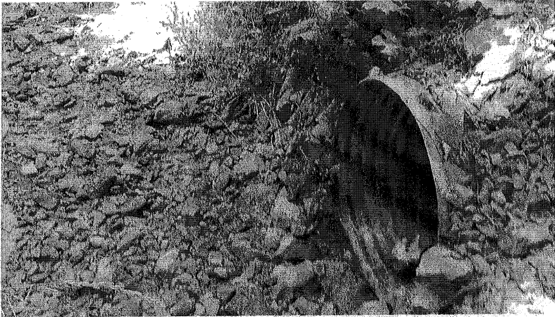
Site 04 – Class III watercourse crossing consisting of a 36” culvert.
