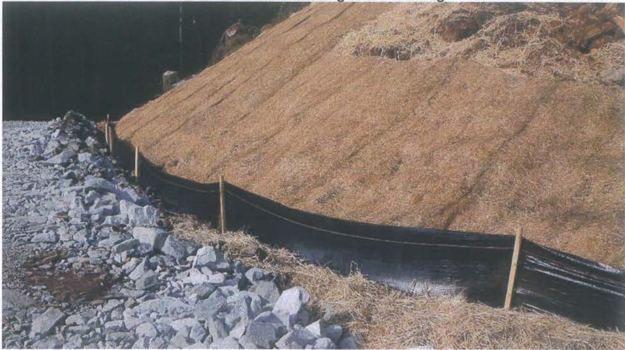
Erosion Control Matting & Silt Fencing
