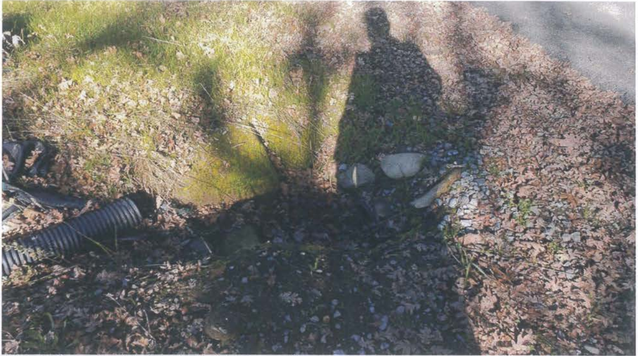
Photo looking at the inlet of the ditch relief culvert at Site 01.
