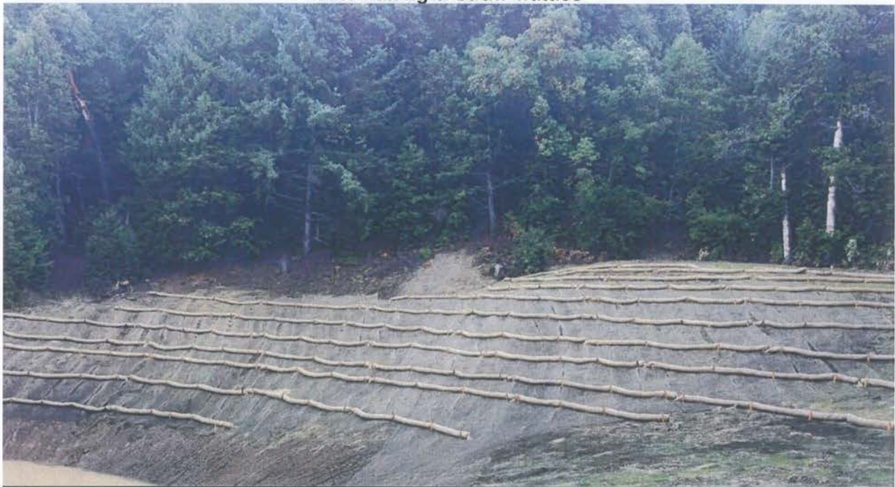
Jute netting & Straw-wattles
