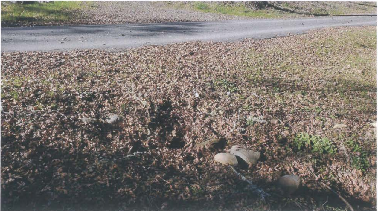
Photo looking at the outlet of the ditch relief culvert at Site 01.
