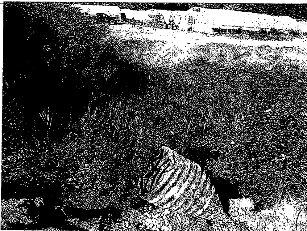
Figure 6. Looking NW at spillway from top of dam at Reservoir 1, POD 2. POU 1 is in background.
