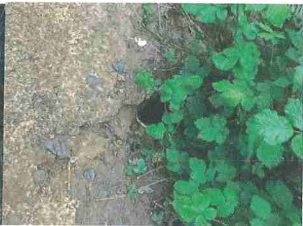
Photo #161, location 41 north end of 18" cpp Inlet.
