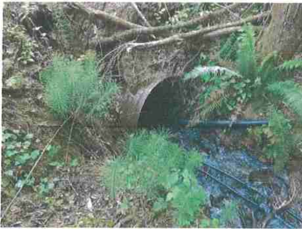
Photo #184, location 45 south east side of road near 18" cmp inlet.
