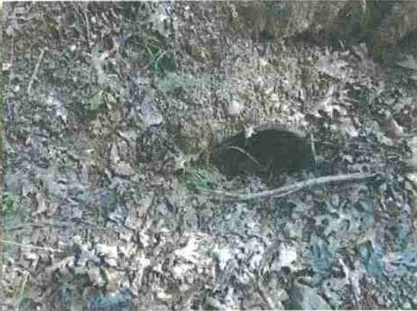
Photo #276, location 69 east end of 30" cmp inlet.
