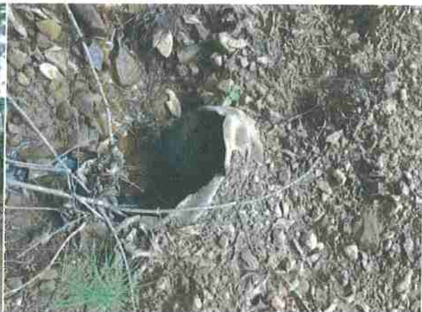
Photo #214, location 53 north side of road 18" cmp inlet.
