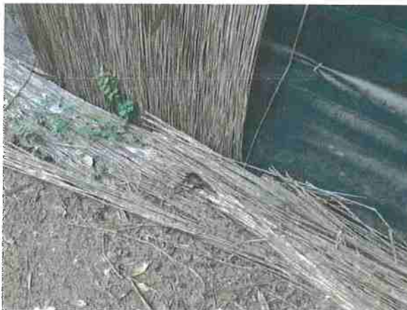
Photo #186, location 45 north west side of road near 18" cmp outlet.
