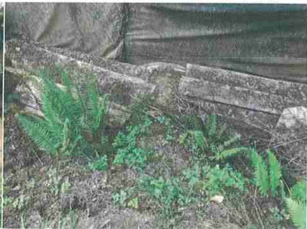
Photo #171, location 43 east 18" cmp outlet.
