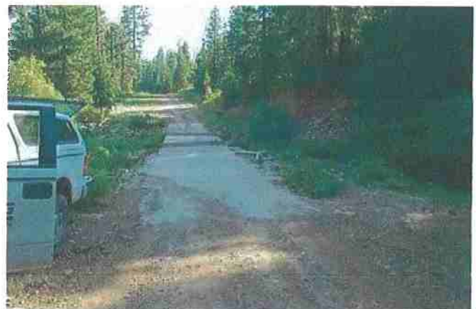
Figure 7. Concreted low-water crossing placed on bedrock outcrop in intermittent stream. Photo: Angela Wilson, Central Valley Regional Water Quality Control Board.
