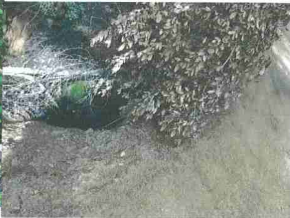
Photo #210, location 51 north side road 18" cmp inlet.
