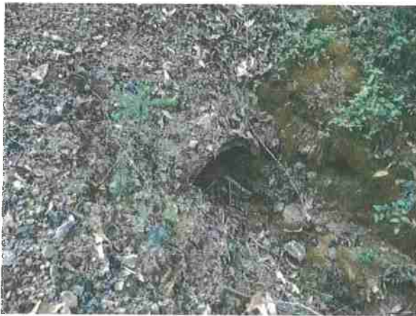
Photo #162, location 41 south end of 18" cpp outlet.
