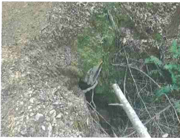
Photo #217, location 53 south side of road 18" cmp outlet.
