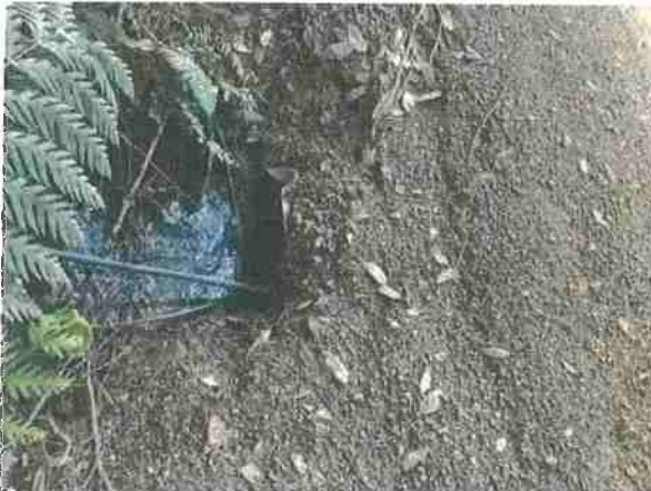
Photo #203, location 50 south side of road 18" cmp inlet.
