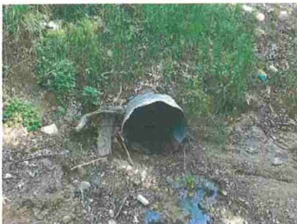
Photo #275, location 69 west end of 30" cmp outlet.
