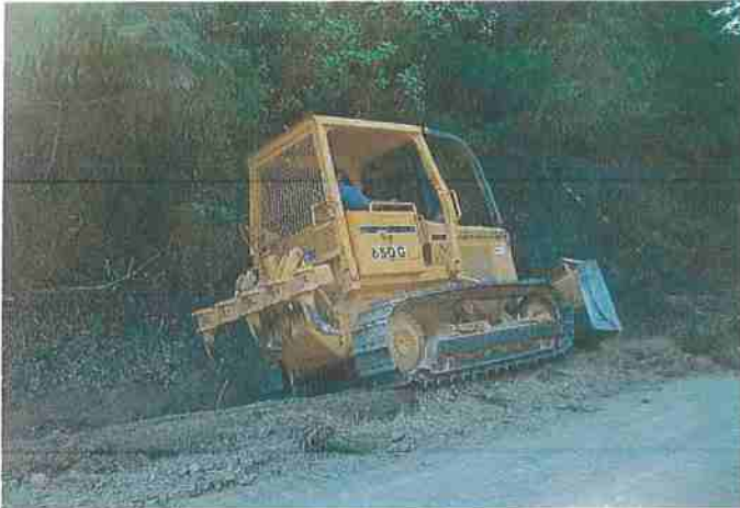
Figure 29. Bulldozer clearing out a road ditch. Photo: Jared Gerstein.
