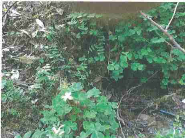
Photo #209, location 51 south side road 18" cmp outlet.
