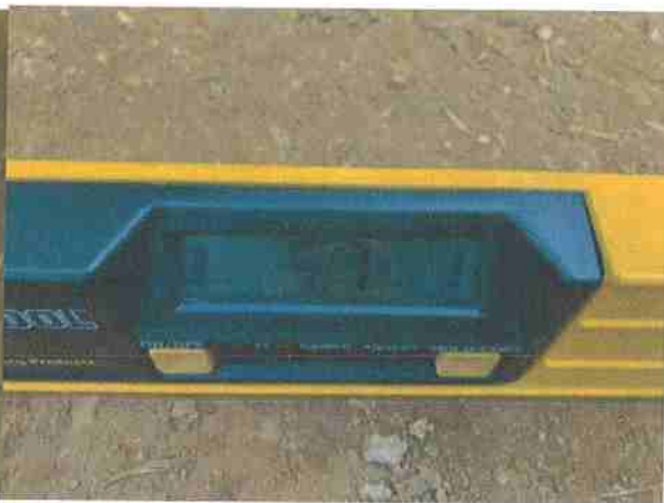
Photo #167, location 42 longitudinal slope = 5.7%.
