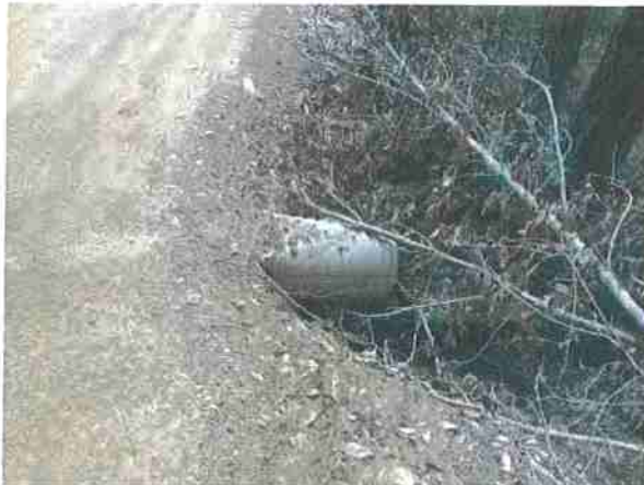
Photo #205, location 50 north side of road 18" cmp outlet.
