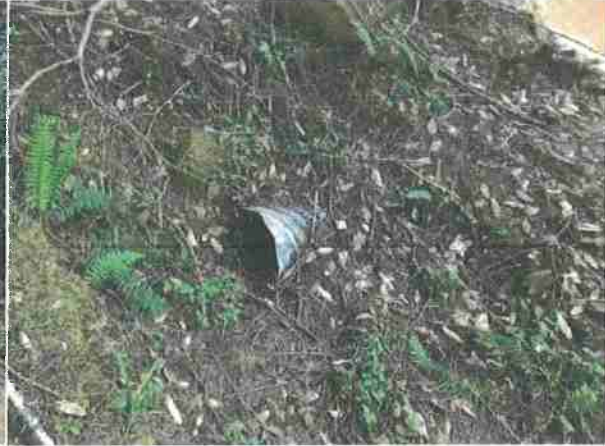
Photo #195, location 49 north end 18" cmp inlet.
