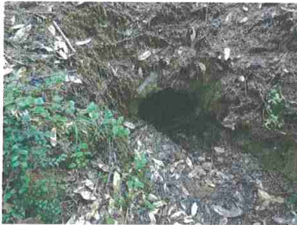
Photo #174, location 44 north 18" cmp inlet
