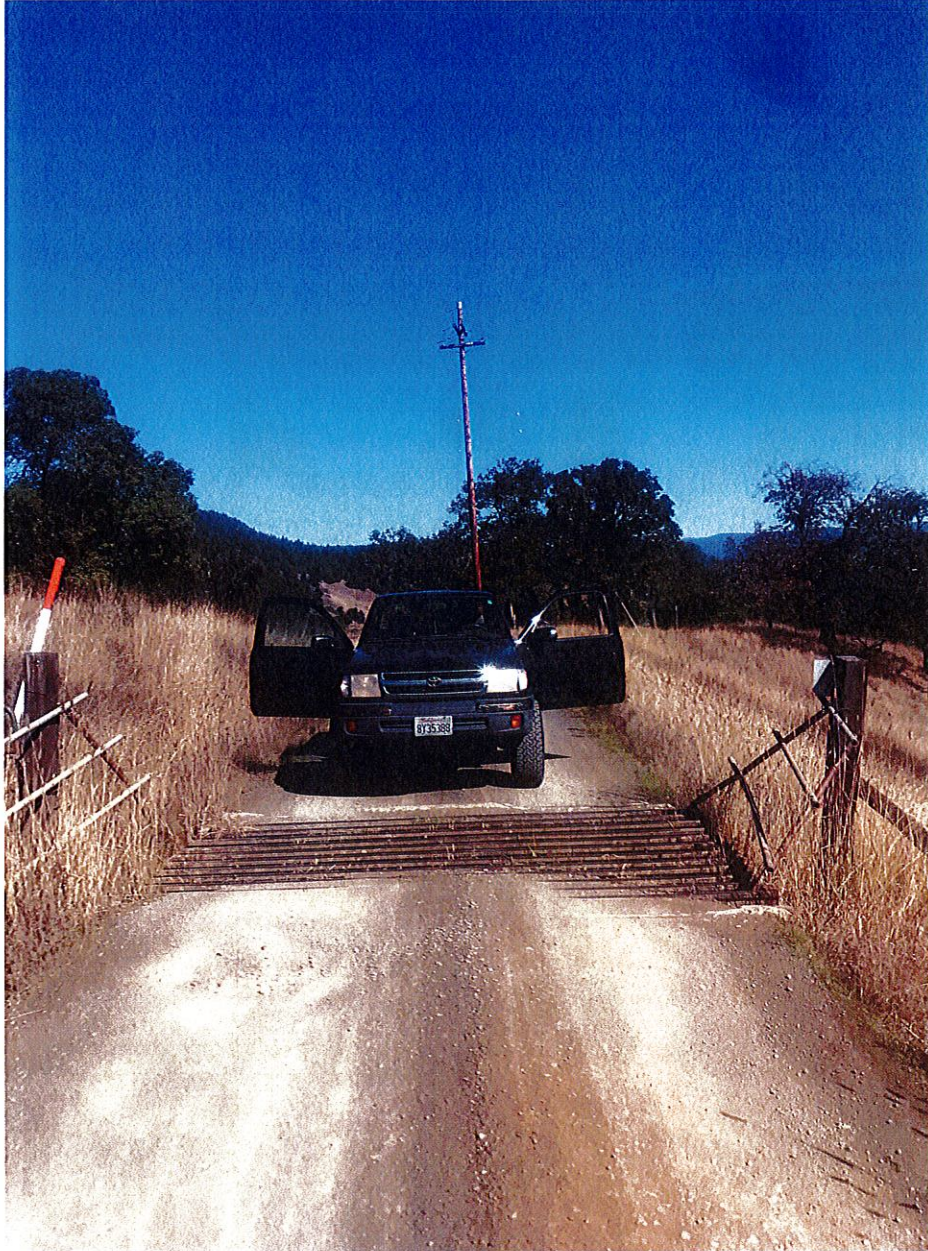
Figure 13: RP-13. Road width: 12' 3" at cattle guard.
