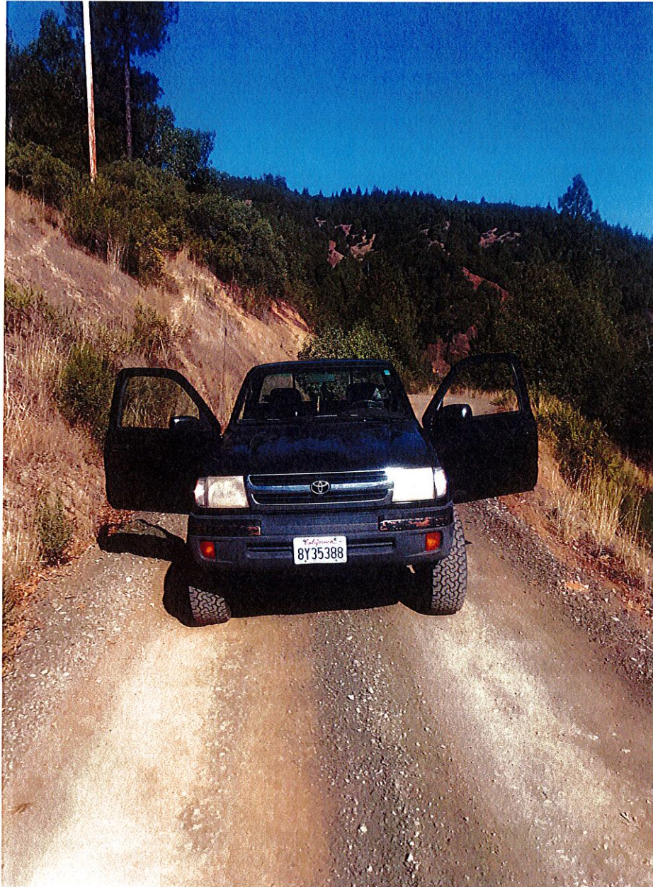
Figure 8: RP-8. Road width: 12'03". Turnout located at PR-9.
