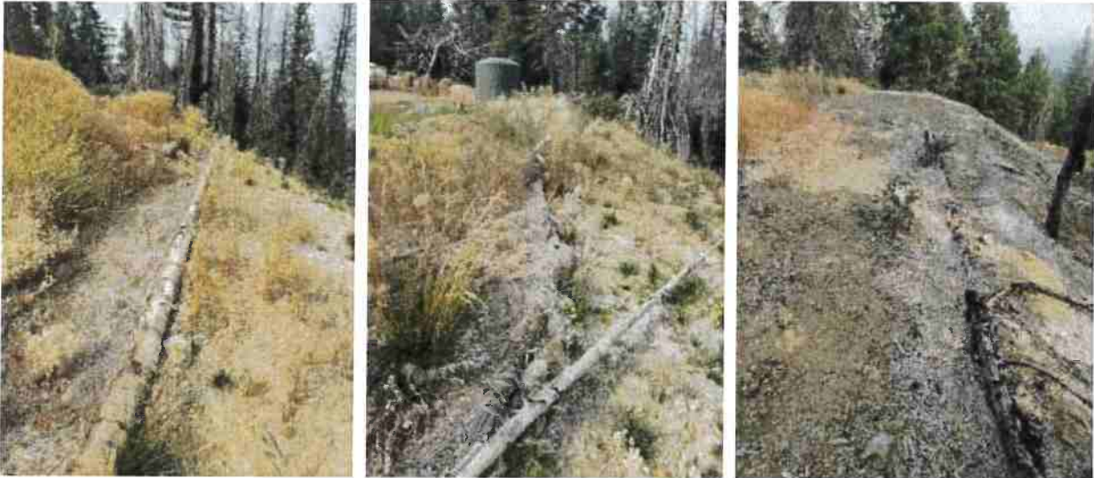
Photo 6a-c. Straw wattle on edge of cultivation flat, to be replaced where no longer functioning
