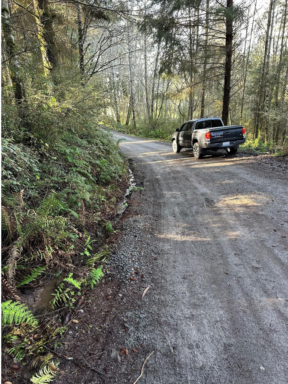
Figure 16: RP 6. Inboard ditch.
