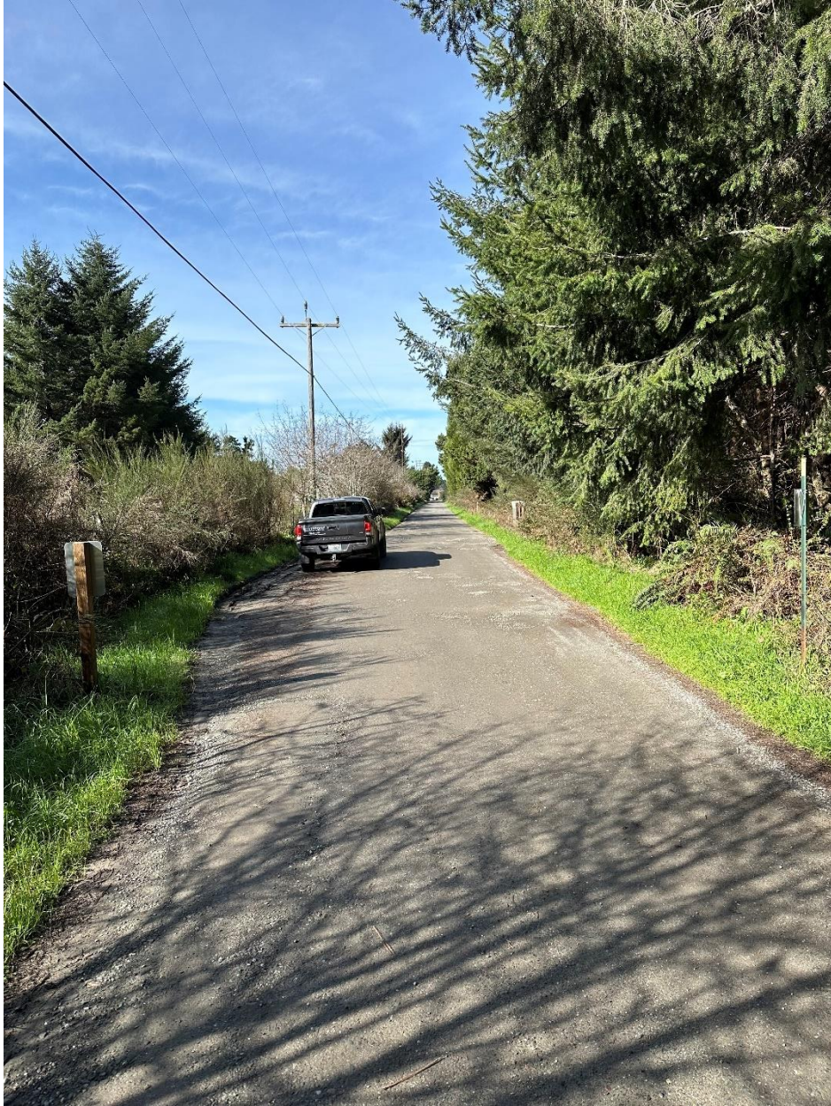
Figure 6: RP 3. Hooven Road transitions from an average width of 16 feet to an average width of 13 feet. Photo Taken facing west, vehicle traveling west, parked in turnout.
