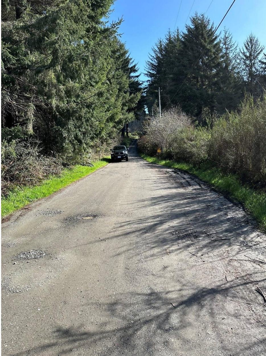
Figure 7: RP 3. Hooven Road transitions from an average width of 16 feet to an average width of 13 feet. Photo Taken facing east, vehicle traveling west.
