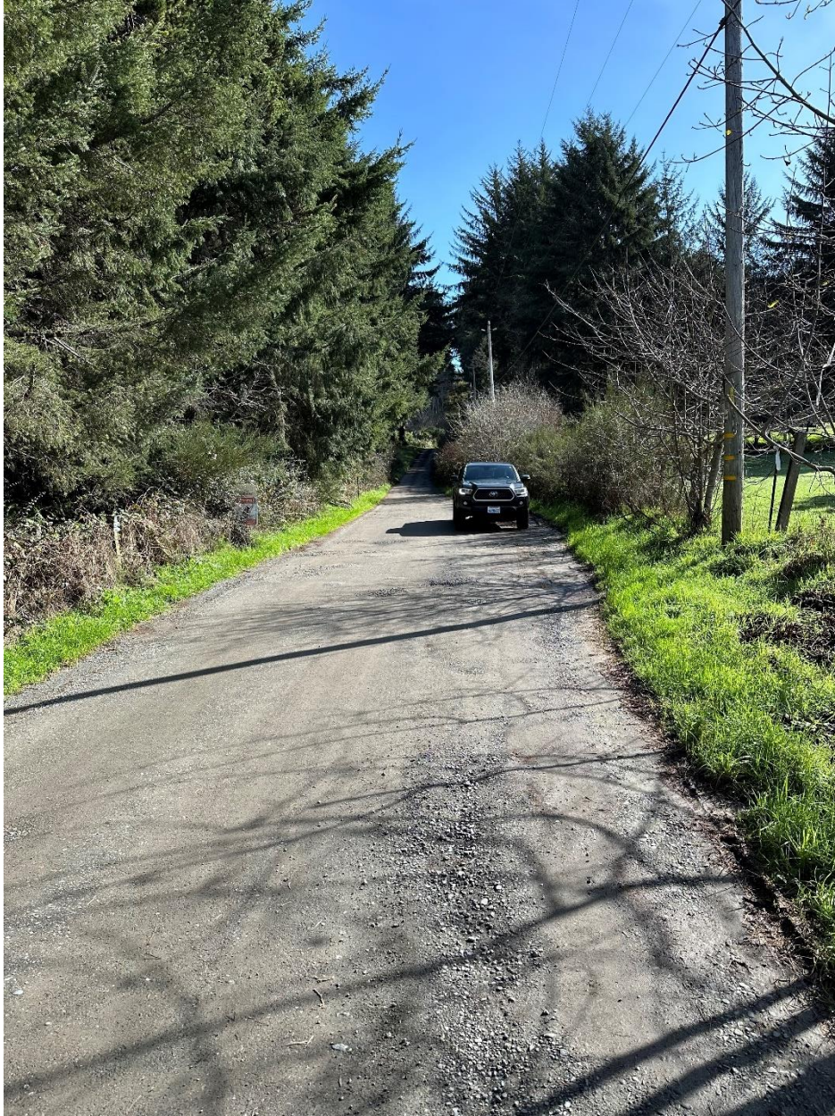
Figure 5: RP 3. Hooven Road transitions from an average width of 16 feet to an average width of 13 feet. Photo Taken facing east, vehicle traveling west, parked in turnout.
