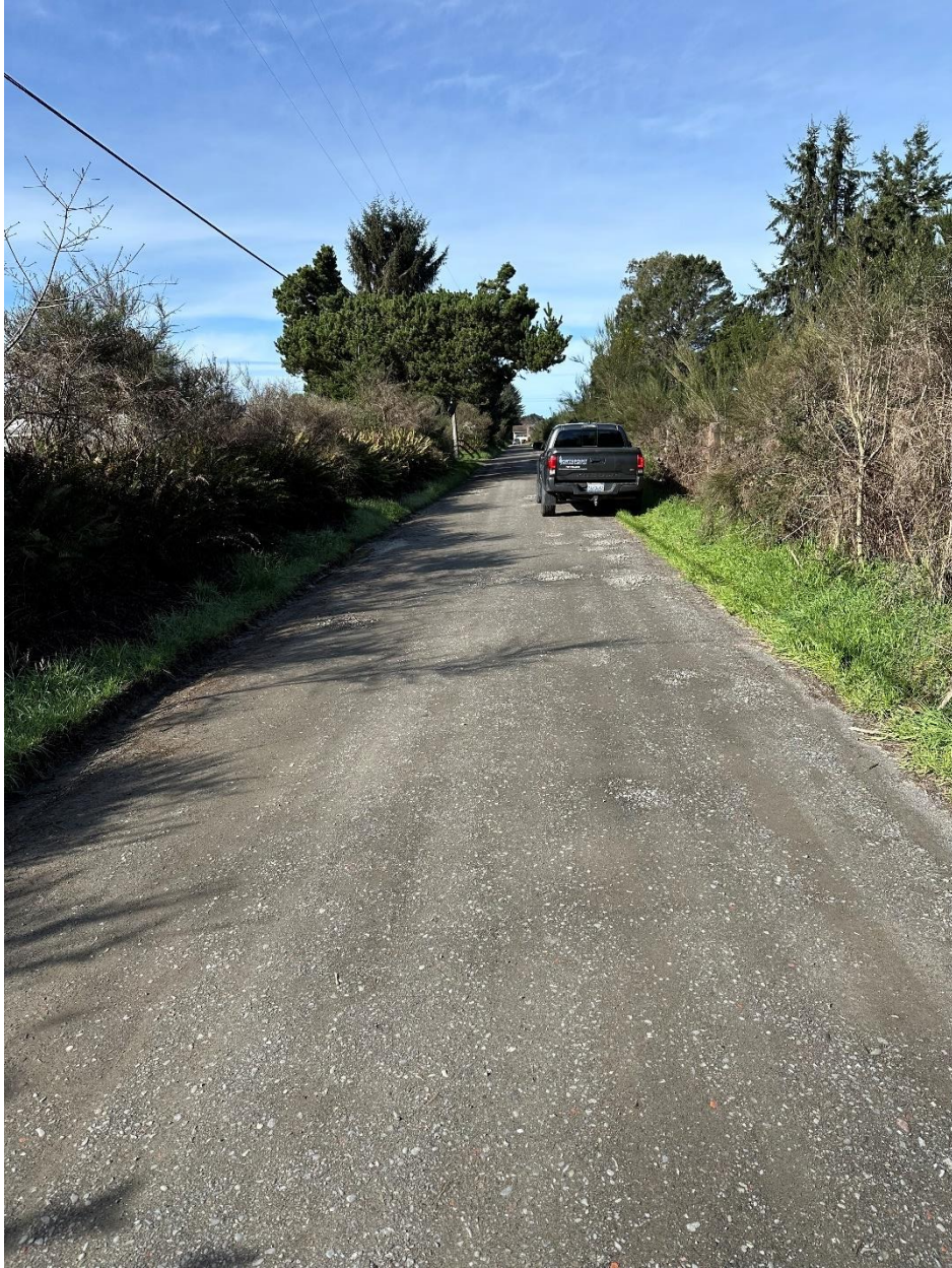
Figure 4: RP 2, typical section of Hooven Road. RP 2, typical section of Hooven Road. Photo Taken facing west, vehicle traveling west.
