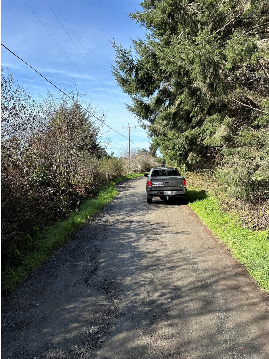
Figure 8: RP 3. Hooven Road transitions from an average width of 16 feet to an average width of 13 feet. Photo Taken facing west, vehicle traveling west.
