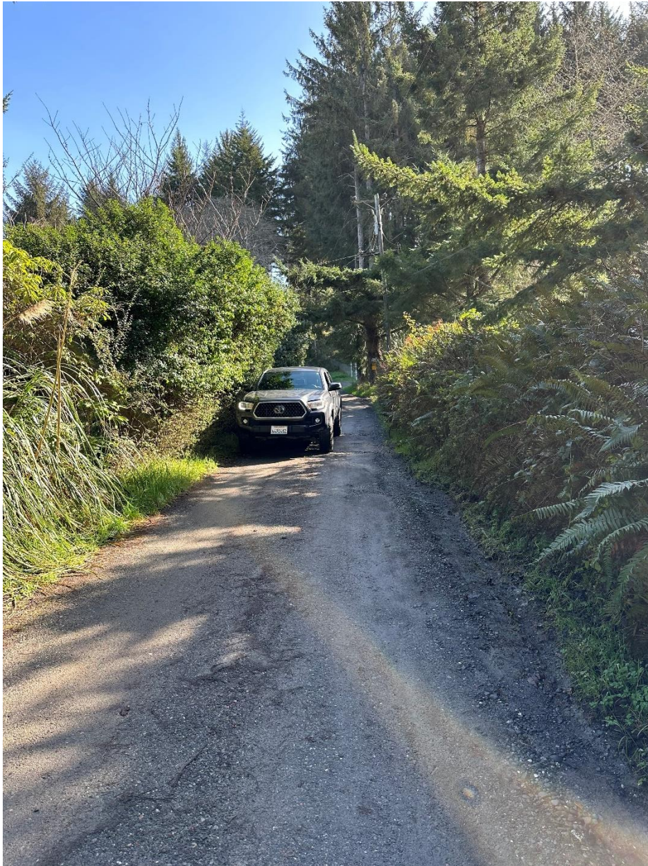
Figure 9: RP 4, pinch point. Vegetation restricts roadway width. Photo Taken facing east, vehicle traveling west.
