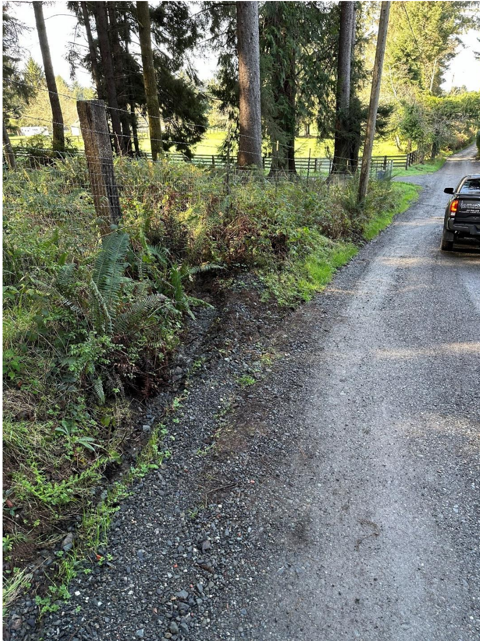
Figure 13: RP 5. Discharge of inboard ditch.
