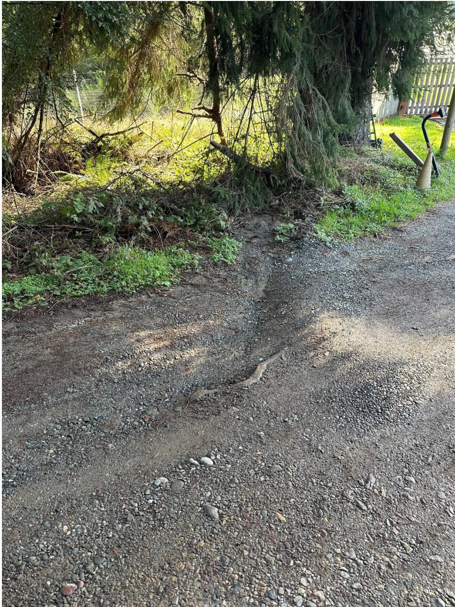
Figure 29: RP 12. Lead-out ditch.
