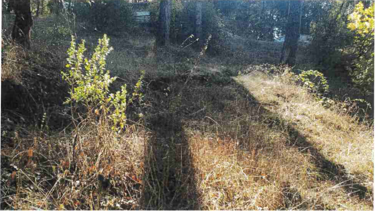
Photo of surface cracks at Site 06.
