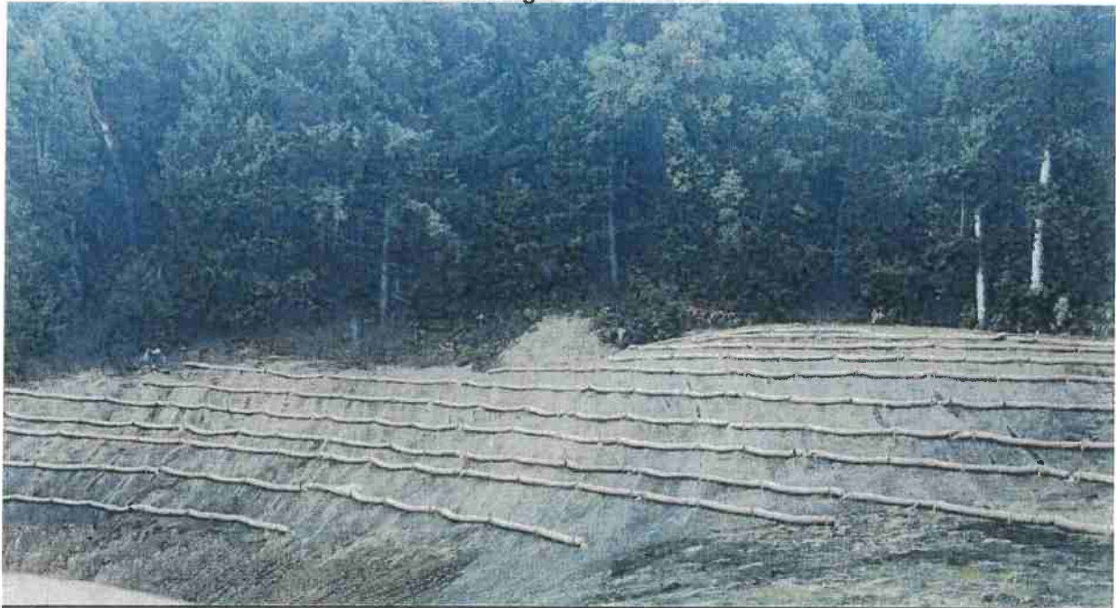
Jute netting & Straw-wattles
