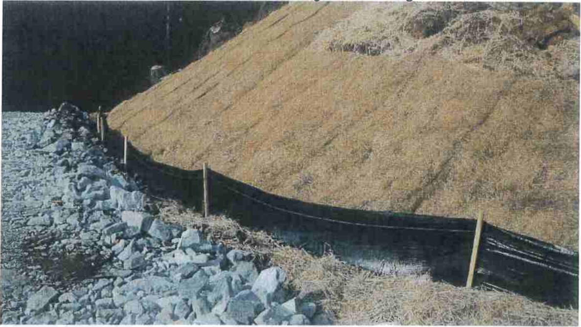
Erosion Control Matting & Silt Fencing
