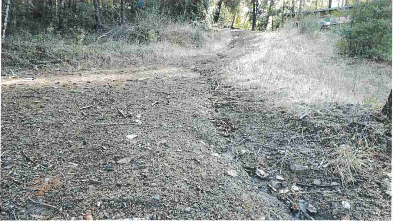
Photo looking up grade at concentrated road surface runoff that is coming from Site 04 and is draining into surface cracks at Site 06.
