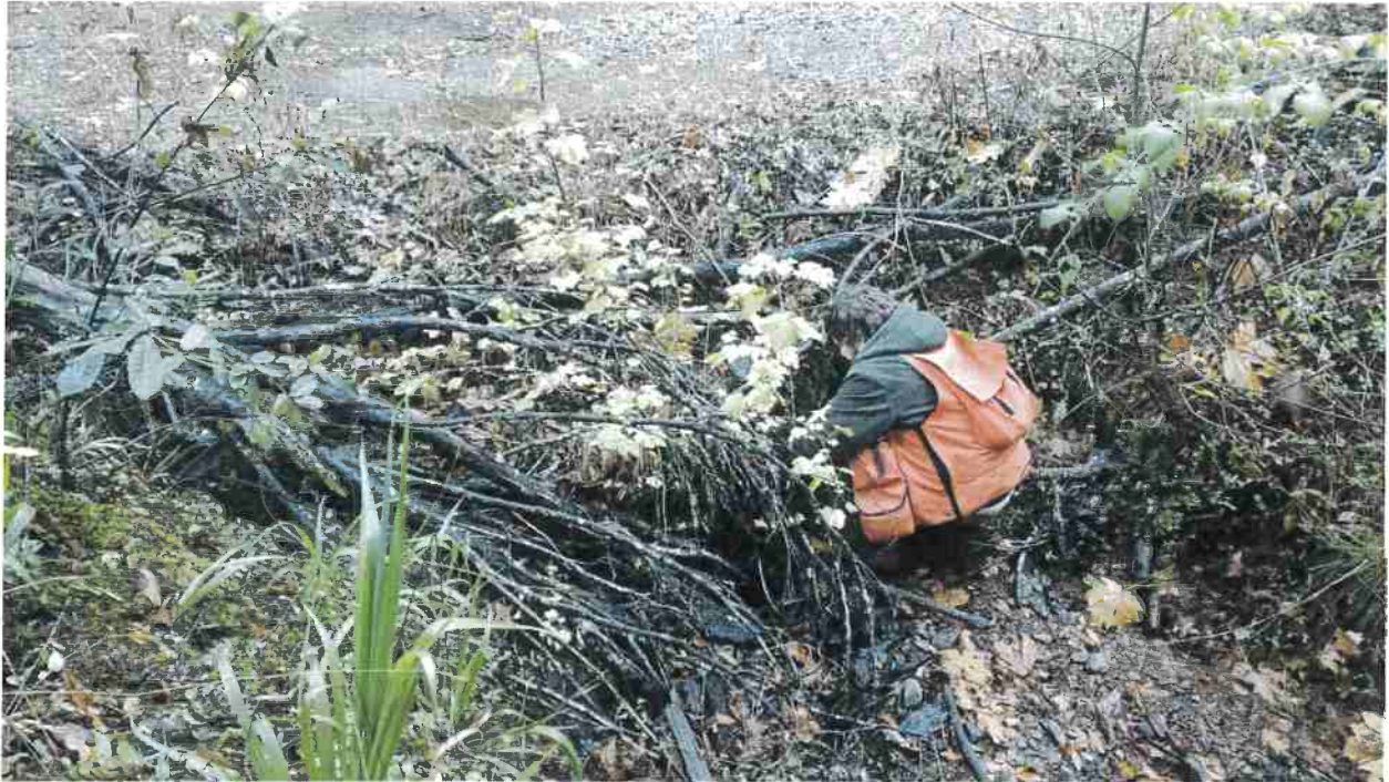
Photo looking at the inlet of the watercourse crossing at Site 13.
