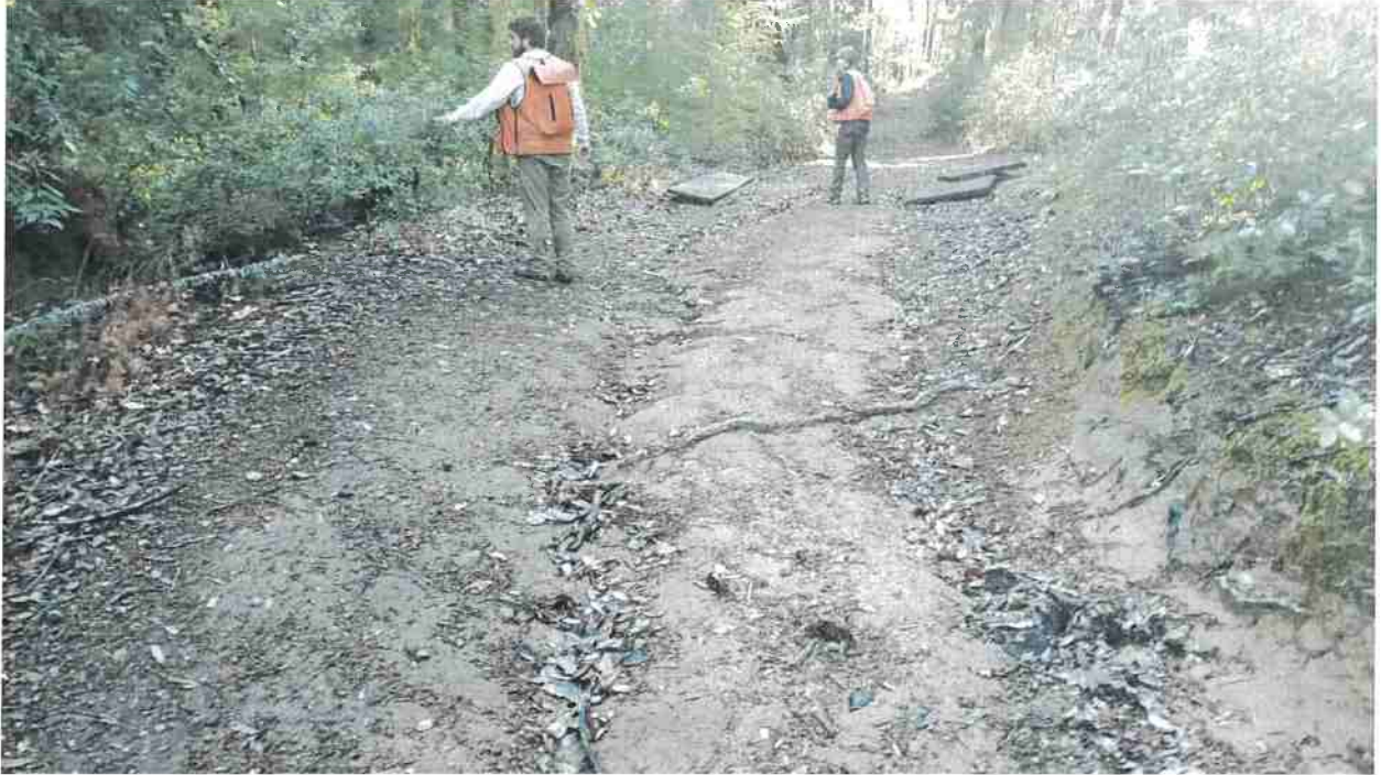
Photo looking up grade at Site 10.
