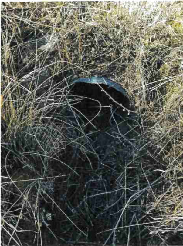
Photo looking at the inlet of the watercourse crossing at Site 17.
