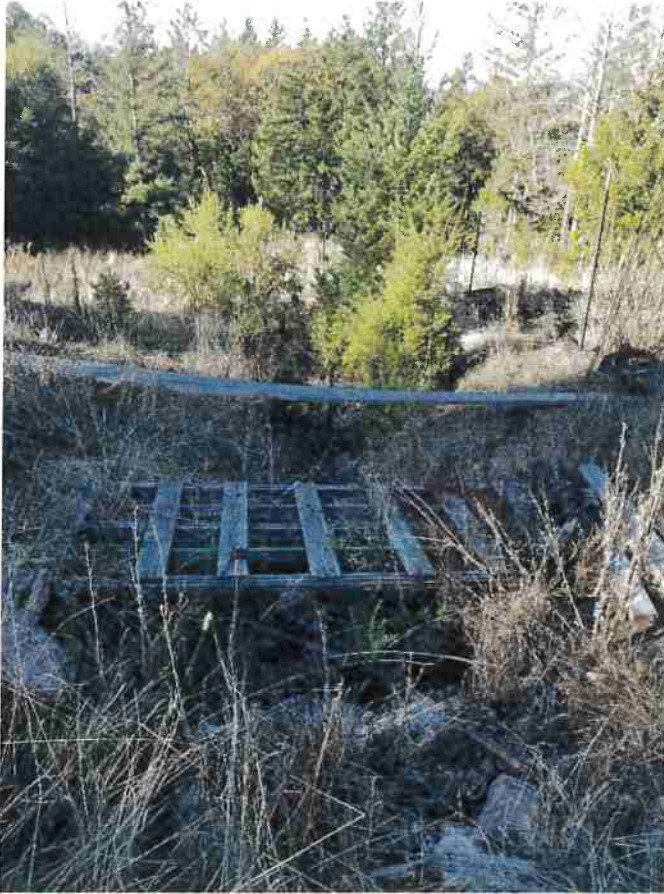
Photo looking down channel from the watercourse crossing at Site 18.
