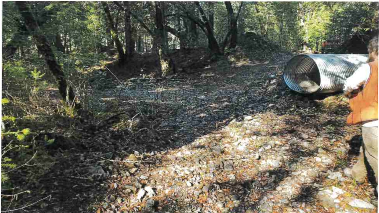
Photo looking down stream at Site 03.
