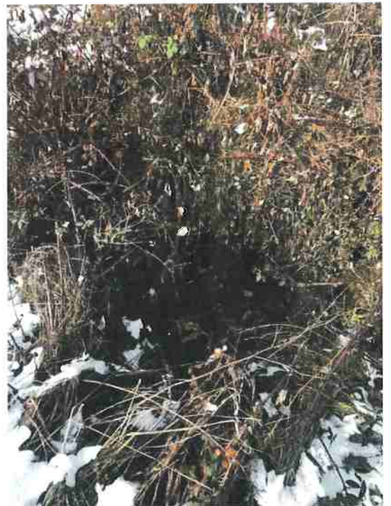
Culvert through road to cultivation area
