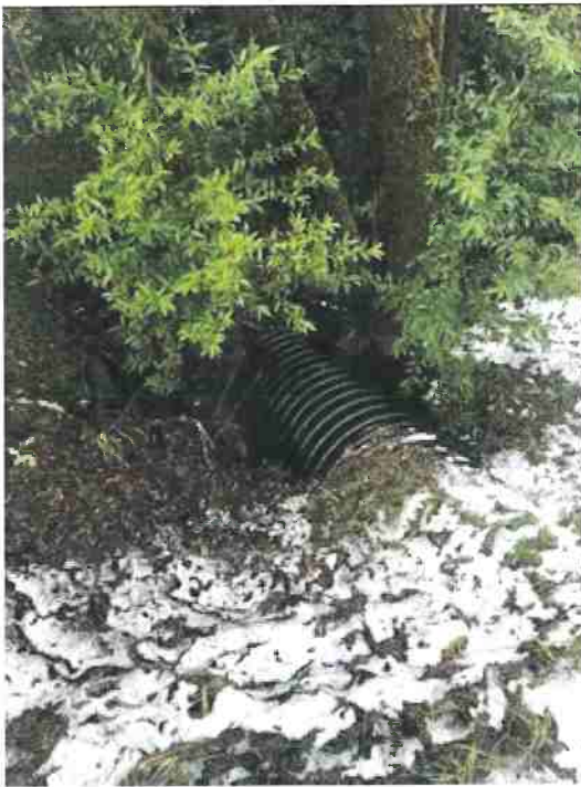
Stream Crossing Culvert near decommissioned greenhouses
