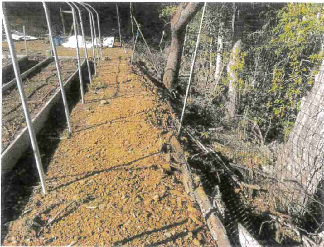
Picture 12: Cultivation Area 5. Perched unstable fill along northern boundary. Photo date 2-8-2019.
