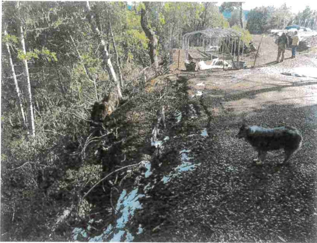
Picture 11: Cultivation Area 5. Perched unstable fill in northwest corner. Photo date 2-8-2019.
