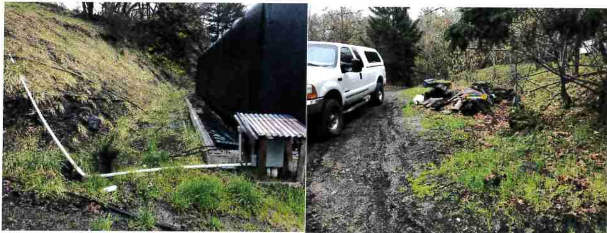
Photo #11 Access Road @ Building Looking West on South Side
