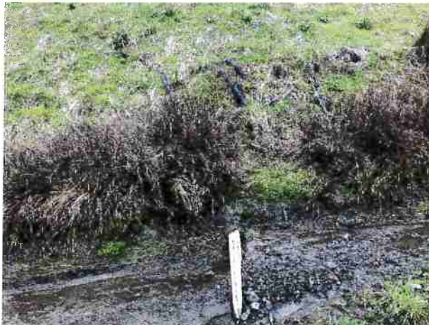
Photo #47 Access Road Looking East at Subsurface Drain
