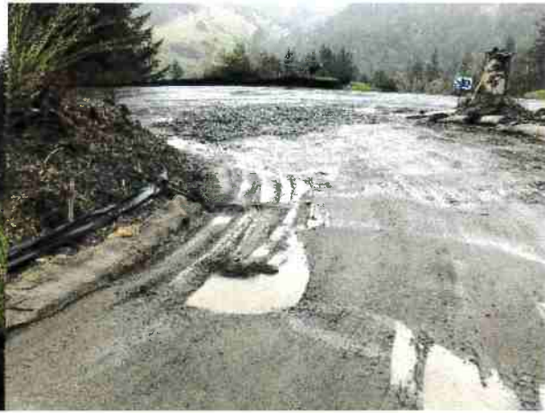
Photo #2 Access Road and Hwy 36 Looking North
