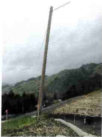
Photo #19 Slope & PP in Hwy 36 Const.
