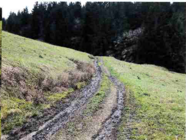
Photo #46 Access Road Looking South
