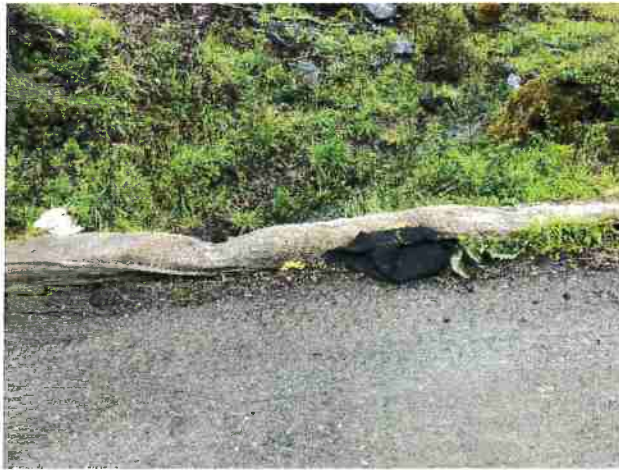
Photo #3 Access Road and 18" Culvert Discharge
