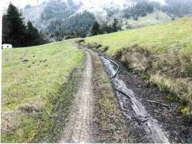
Photo #31 Access Road Looking North
