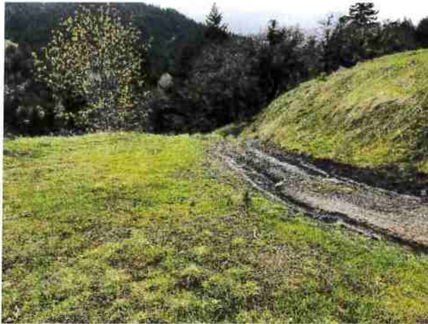
Photo #45 Access Road Looking Northeast @ Curve w/ Pullout
