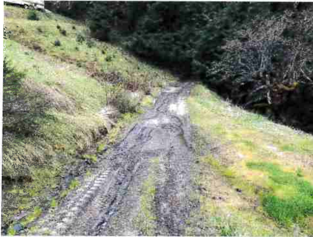
Photo #21 Access Road Looking Southwest
