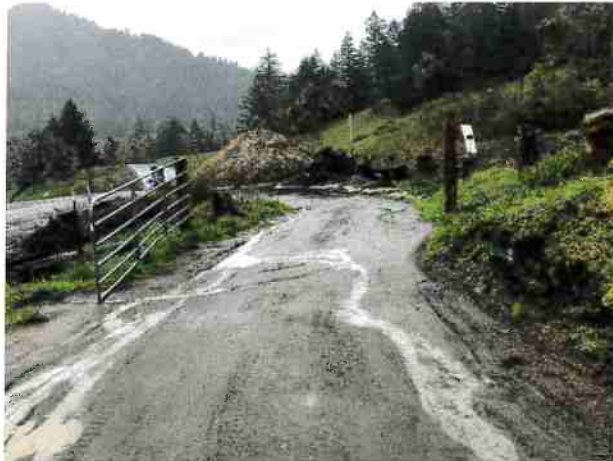
Photo #5 Access Road Looking North
