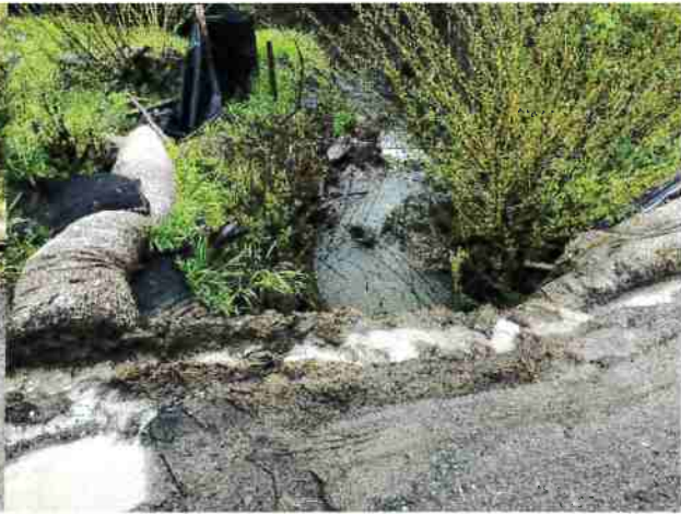
Photo #4 Access Road and 18" Culvert Discharge Inlet
