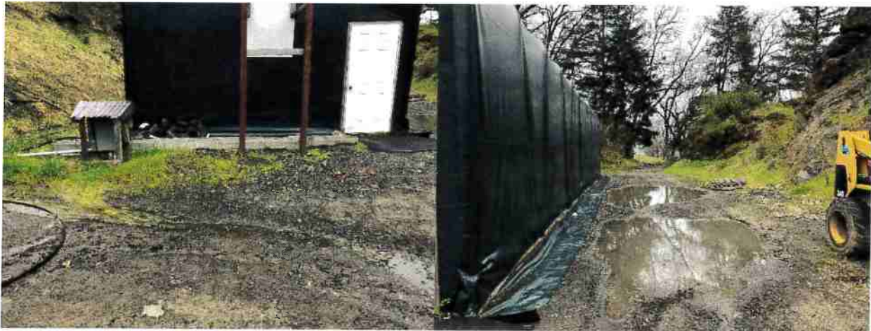
Photo #9 Access Road @ Building Looking West
