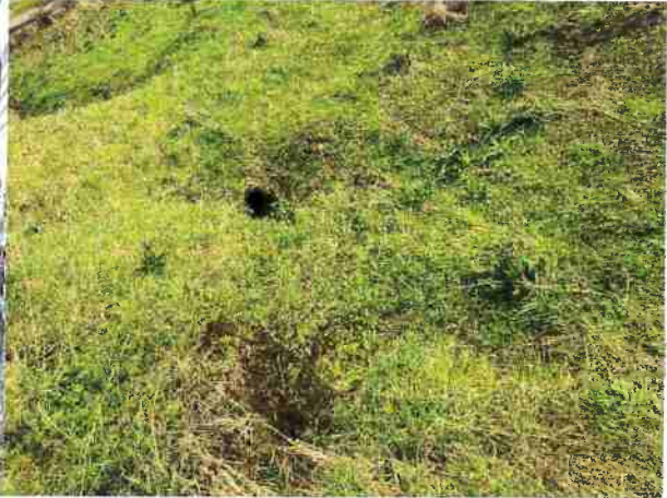
Photo #26 Access Road 12" Culvert Discharge
