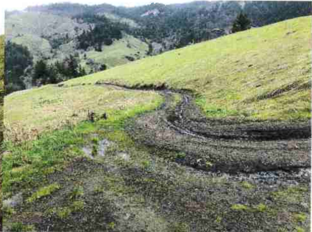
Photo #34 Access Road Looking West @ Curve w/ Pullout
