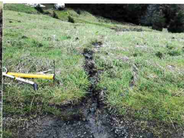
Photo #48 Access Road Looking West @ Other Side of Drain
