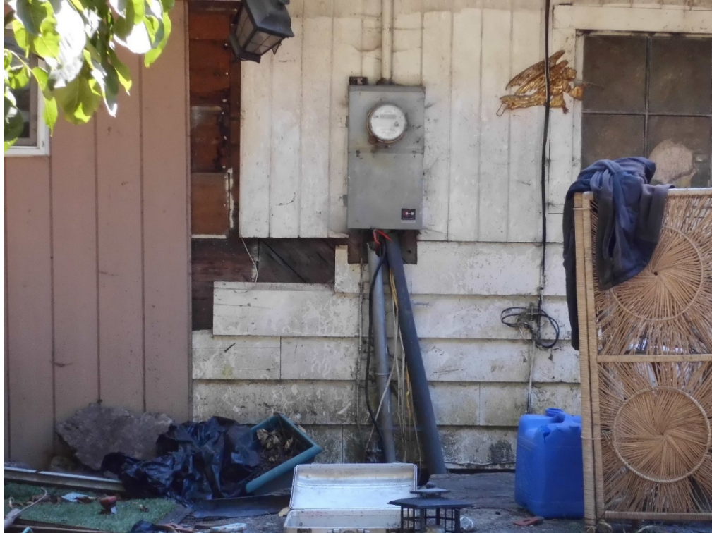
Before Abatement 8/31/2018 - Dangerous electrical service connection
