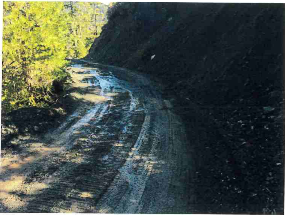
Photo 9. MP9 - Road surface at small fill crossing.
