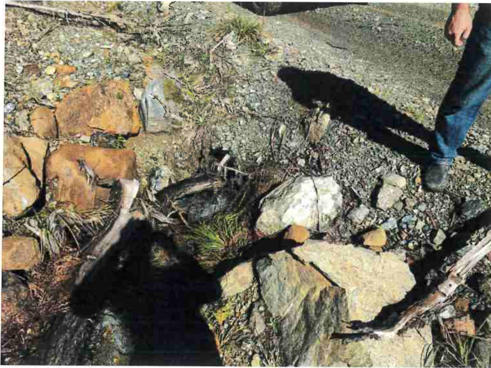
Photo 3. MP7 - Culvert inlet.
