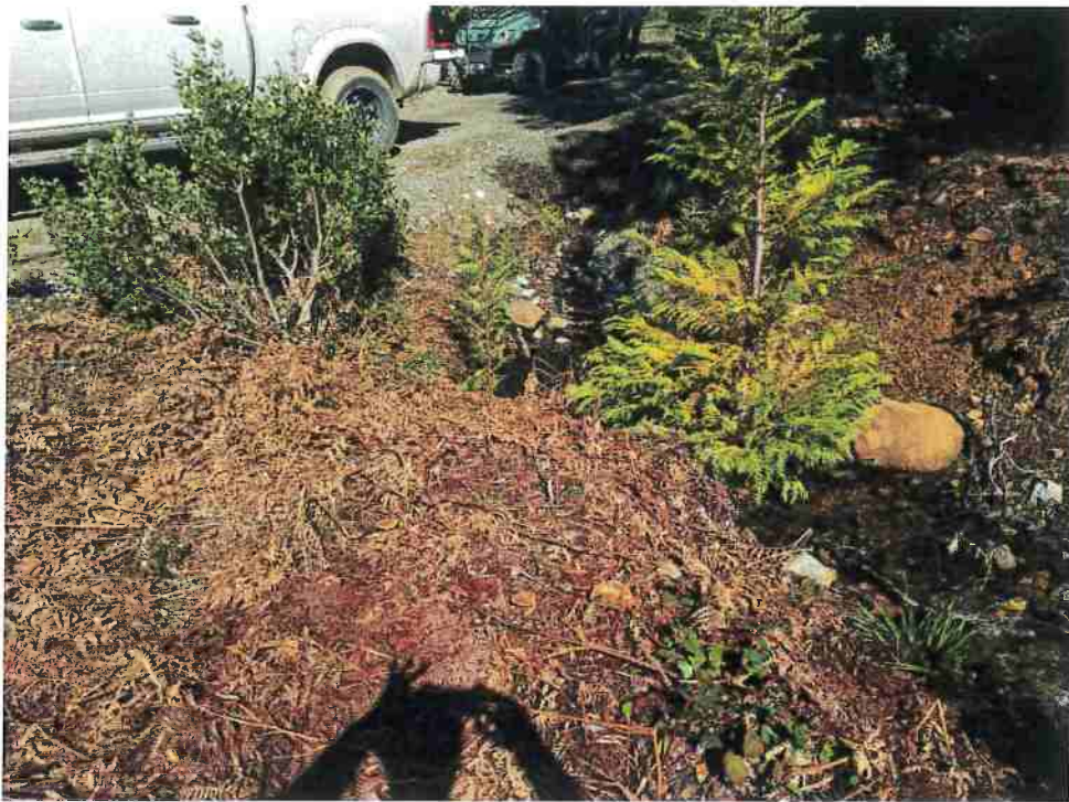
Photo 5. MP8 - Channel upstream from 18" culvert inlet.
