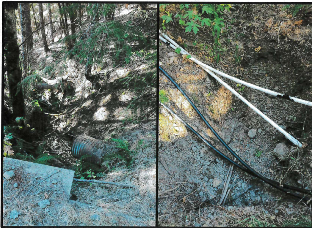
Image 10 - Culvert bottom and top
