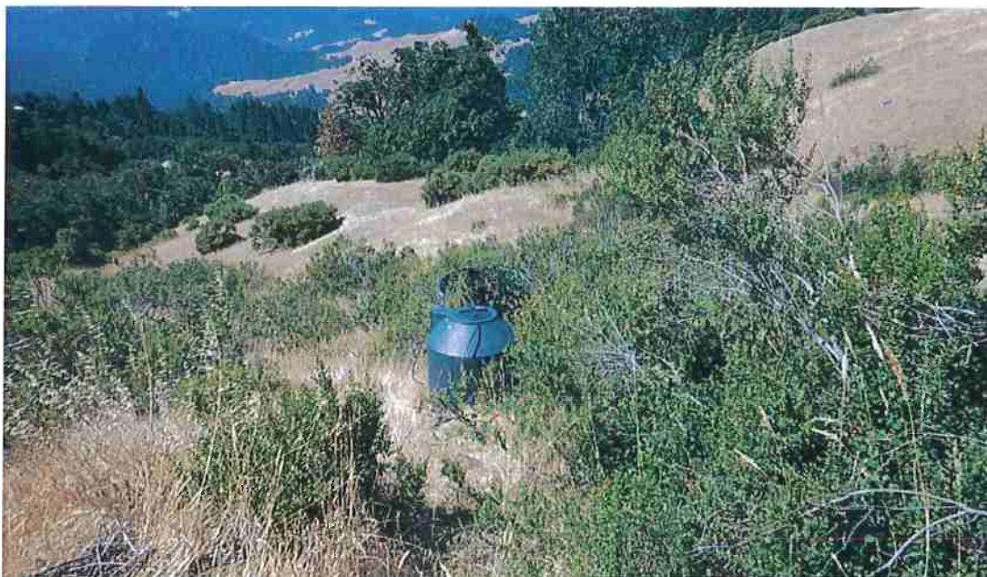
Photo 10: 300gal and 500gal tanks at previous stream diversion. Corrective Action 5.
