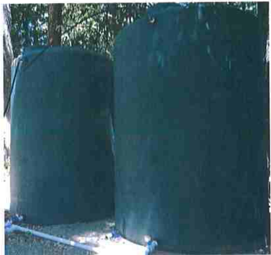
Photo 19: Well and two 5,000gal tanks
