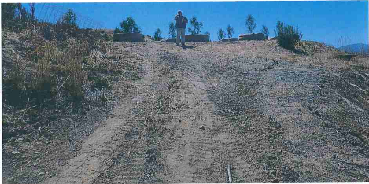
Photo 7: Looking upslope at Garden #3; runoff from this garden comes down this stretch and connects to ditch. Corrective Action #8
