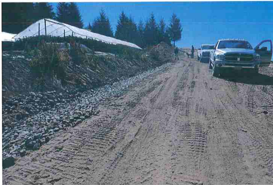
Photo 4: Looking up road from 24” culvert at ditch runoff from grow area 1. Will need to redesign flat drainage away from stream. Corrective Action 2.
