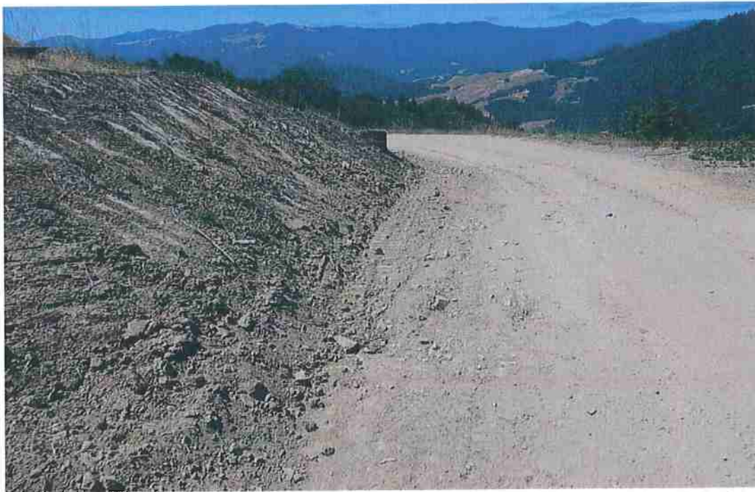
Photo 8: Looking down main road. Runoff from Garden #3 (Photo 7) delivers to inboard ditch here and into stream below.
