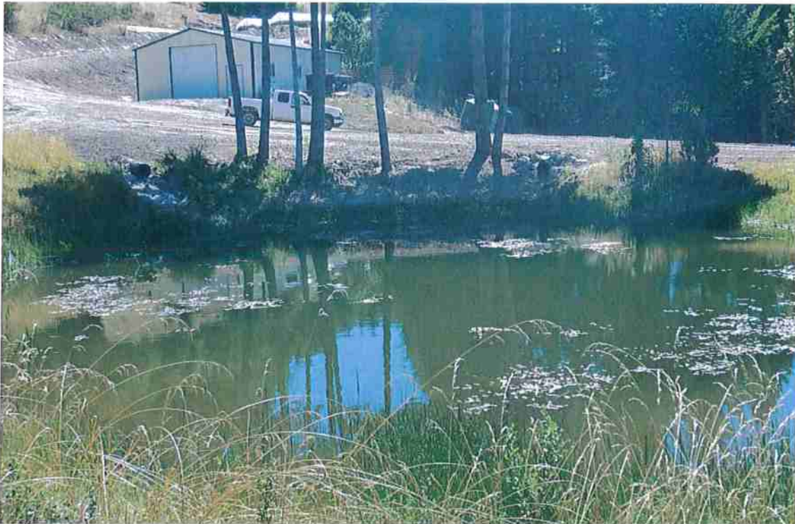
Photo 13: Aesthetic pond. Input DRC on left, overflow culvert on right. Storage and processing building and tilted tanks (Corrective Action 7) in background.
