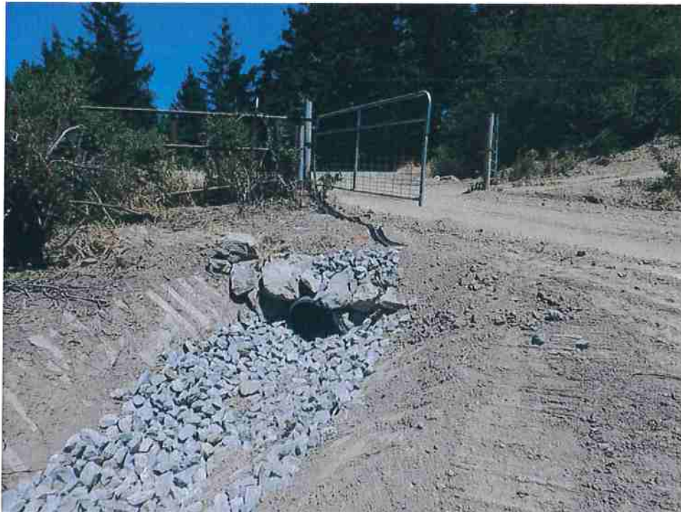
Photo 22: Looking up at DRC outlet at gate.
