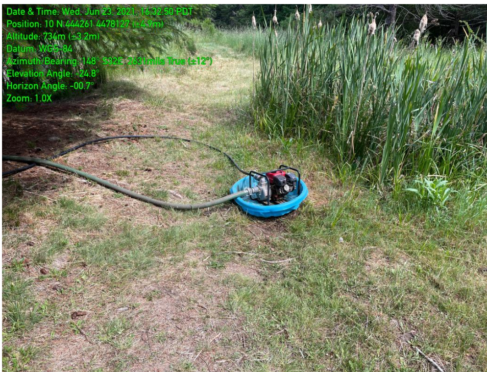
4.0 Pump for Water Diversion at POD 2
