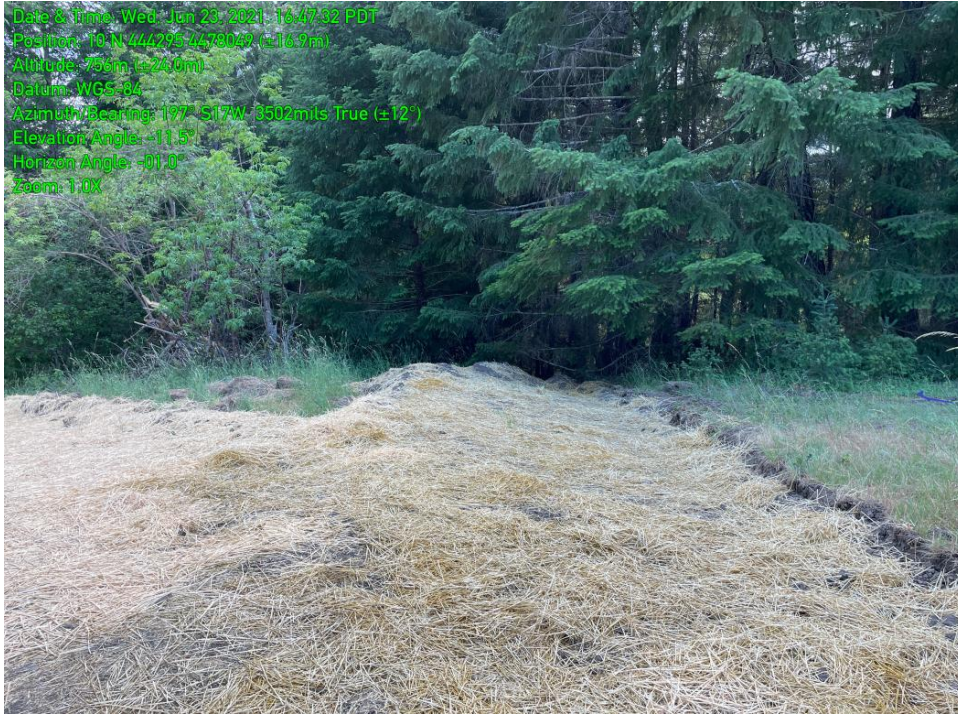
9.0 Mulched Area of Disturbed Soils
