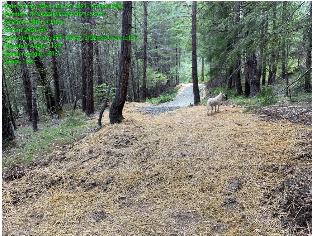
11.0 Mulched Soils and Rocked Road
