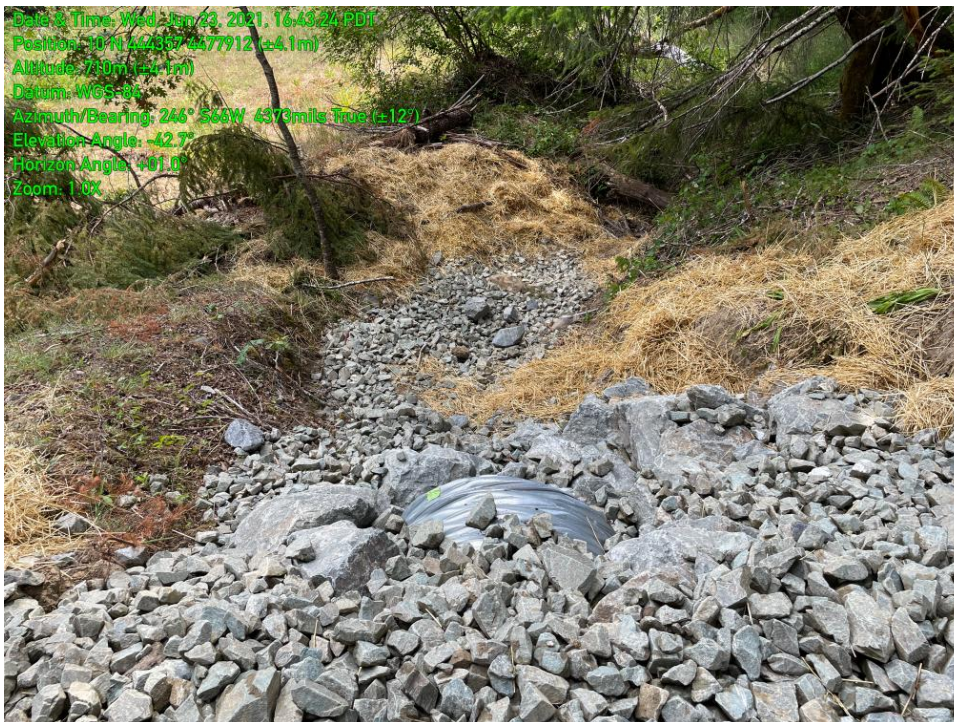
8.0 New Drainage Culvert and Rocked Drainage Area
