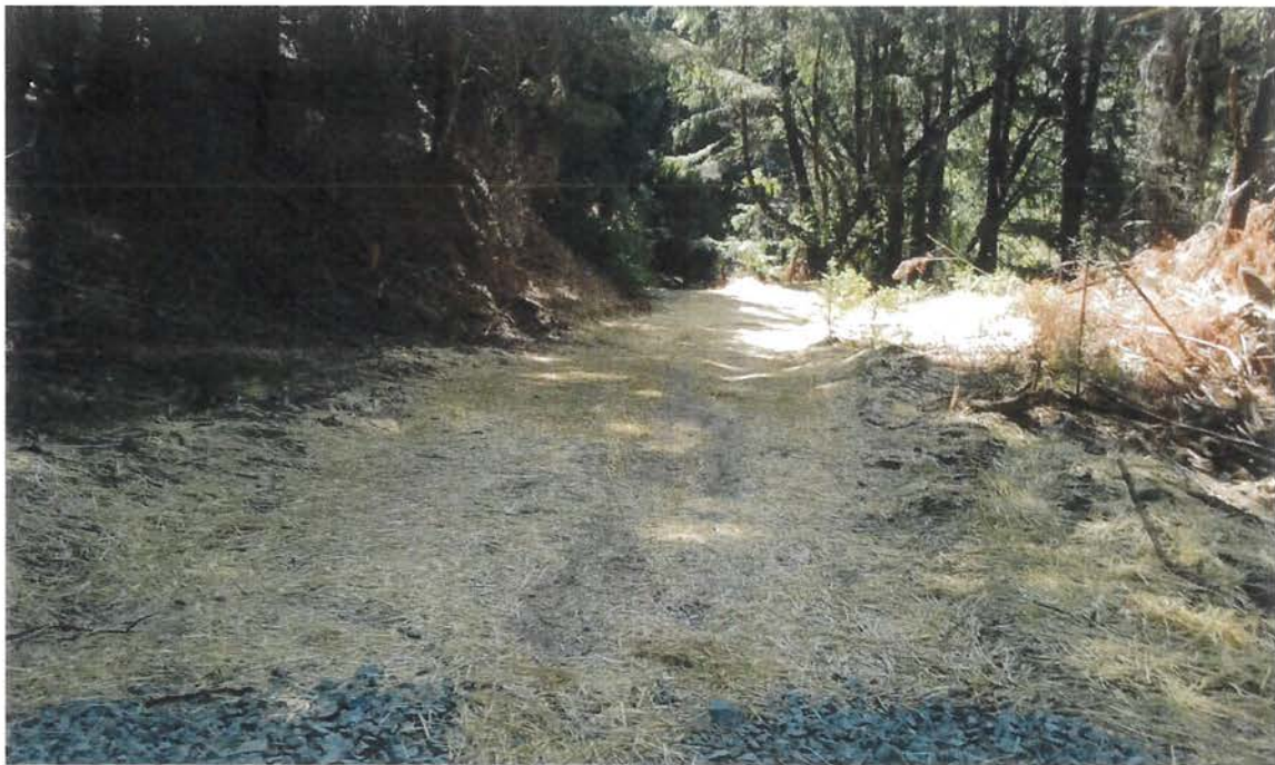
Photos show an example of the dirt surfaced seasonal road on the property. The roads were graded with rolling dips installed recently. Following grading, straw was placed for erosion control. The cultivator shall continue to maintain and grade road surfaces as necessary in the future to keep up a functioning, outsloped drainage pattern in the future. Photo date 9/9/2021.
