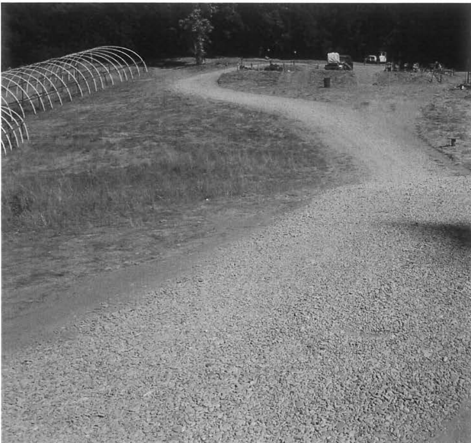
Photos show an example of the rocked, permanent road surfaces throughout the majority of the property. The cultivator shall continue to maintain and grade road surfaces as necessary to keep up a functioning, outsloped drainage pattern in the future. Photo date 9/9/2021.
