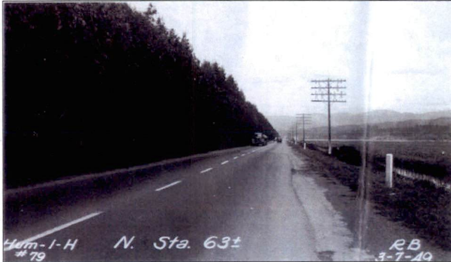
Plate 3: 1949 view of west section of tree row. Note the two-lane US 101 Highway. Field on right is current location of Mid-City Auto World. 15
