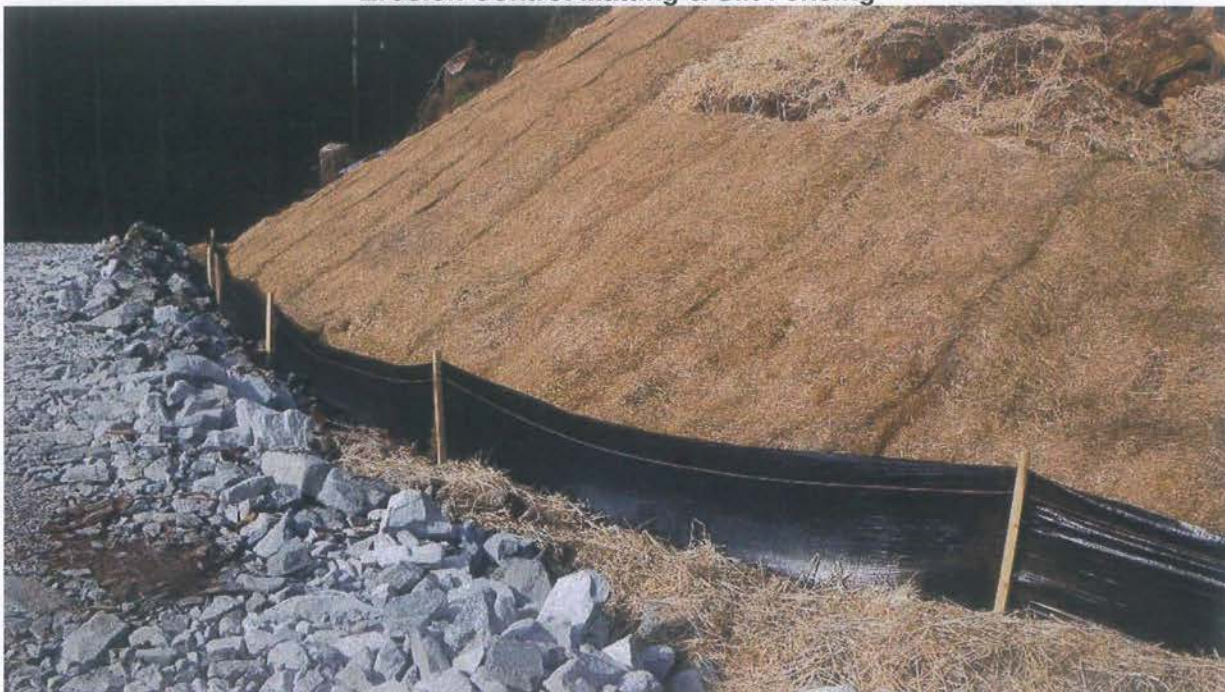
Erosion Control Matting & Silt Fencing
