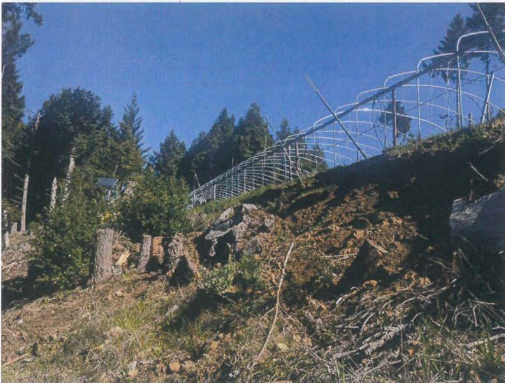
Site 17 where the Cultivator shall install Gabion cages to reinforce the fill slope.
