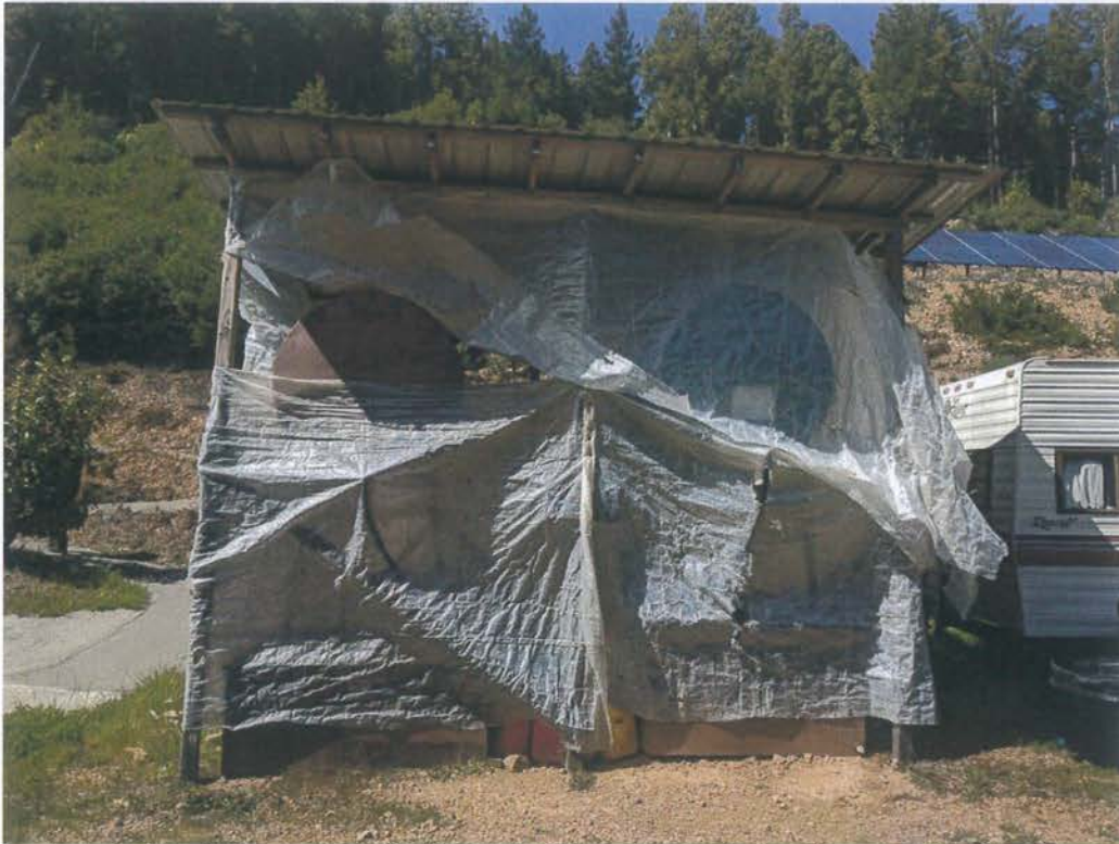
Inadequate diesel storage at Cultivation Area A. The structure lacks adequate side cover from precipitation.
