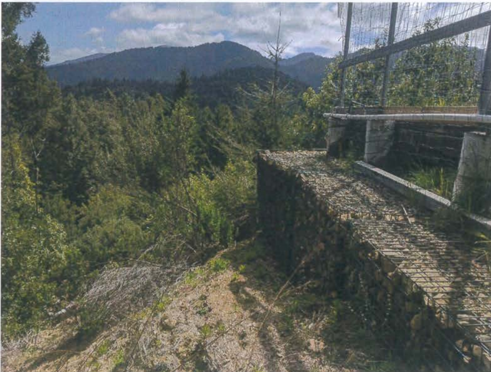
Site 10 with Gabion cages installed to reinforce the fill slope.
