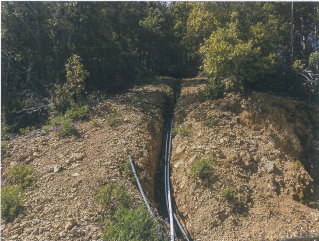
Site 09 with an open trench for a water line that shall be filled in.
