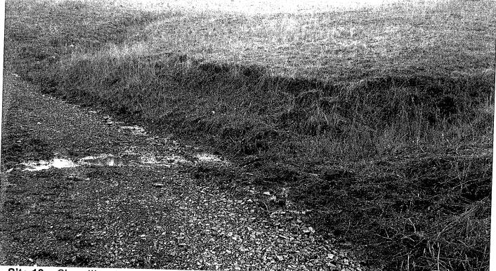
Site 13 – Class III watercourse crossing consisting of a rock ford. It has been recommended to install additional rock consisting of 3-6" minus on the 15 feet of inside ditch.
