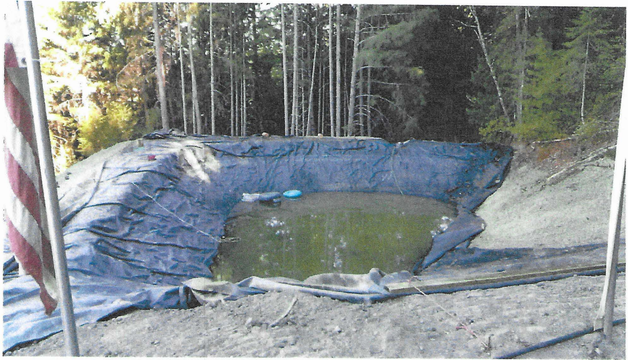
Picture 8: This is a photograph of the off-stream pond located on the property. At the time of this photograph the eastern edge was in disrepair however the landowner has repaired this and anchored the pond liner. The pond is approximately 73 feet long and 68 feet across holding an approximate 170,000 gallons. Photo date: 08/11/2016
