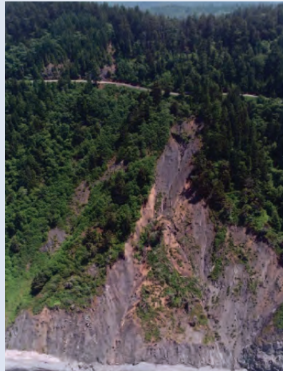
Gully erosion at Last Chance Grade, Highway 101, Del Norte County (left panel) and diagram of processes affecting the site (right panel) from CalTrans (2014)
