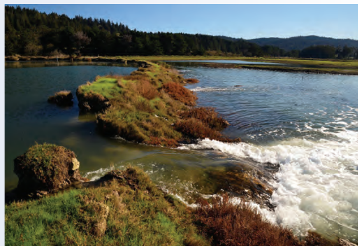
Dike overtopped during a king tide tidally inundating low-lying lands in southern Humboldt Bay (Photo: Aldaron Laird)
