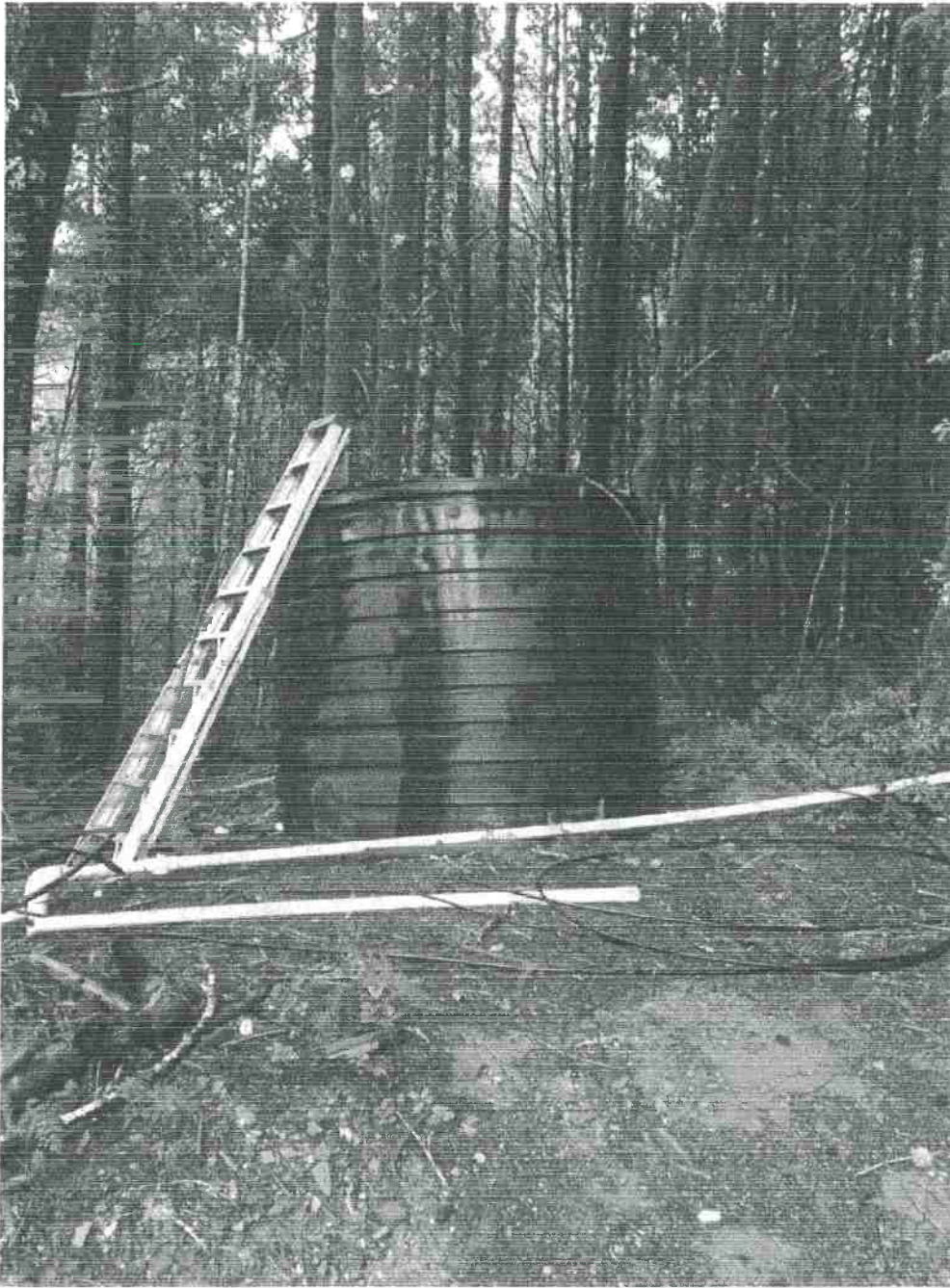
Picture 4: This is a photo of a 2,500 gallon storage tank, which provides water to the residence. Photo Date 12-23-2015.
