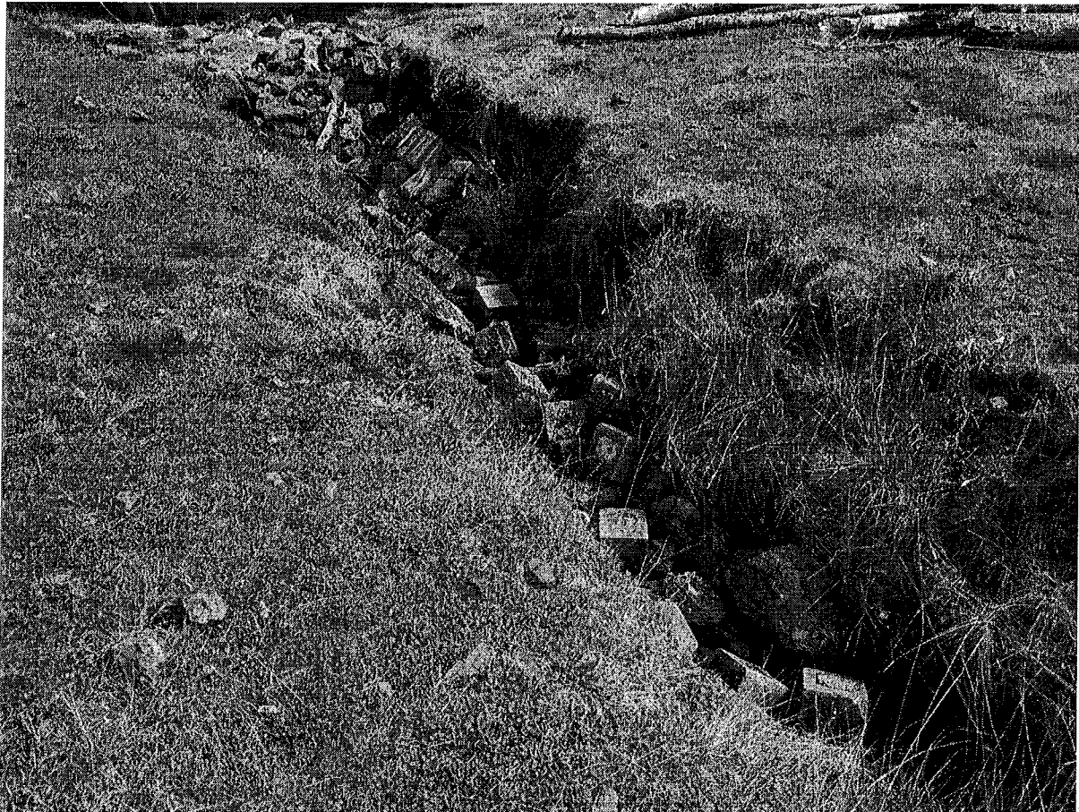
Photograph #32 – View of spillway associated with onstream pond
