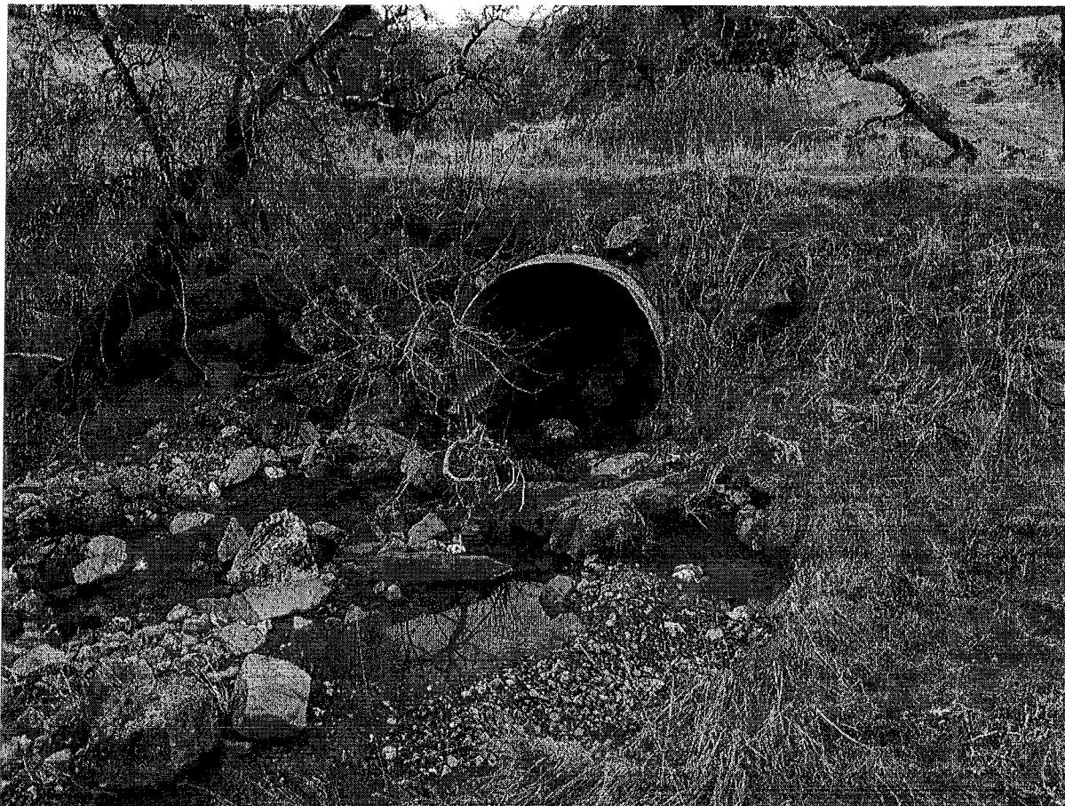
Photograph #26 – At Stream Crossing #12 view upstream; invert embedded
