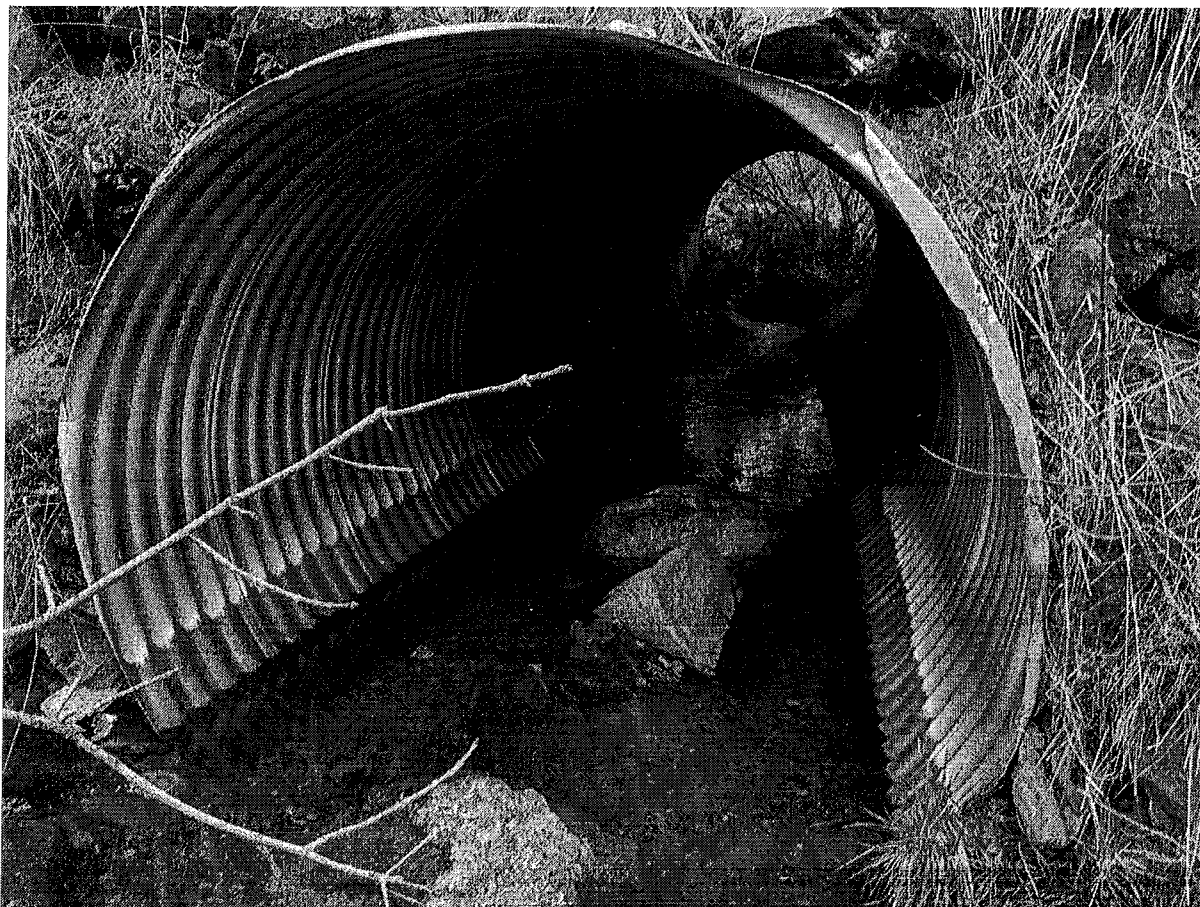
Photograph #28 – At Stream Crossing #12 view upstream of embedded invert
