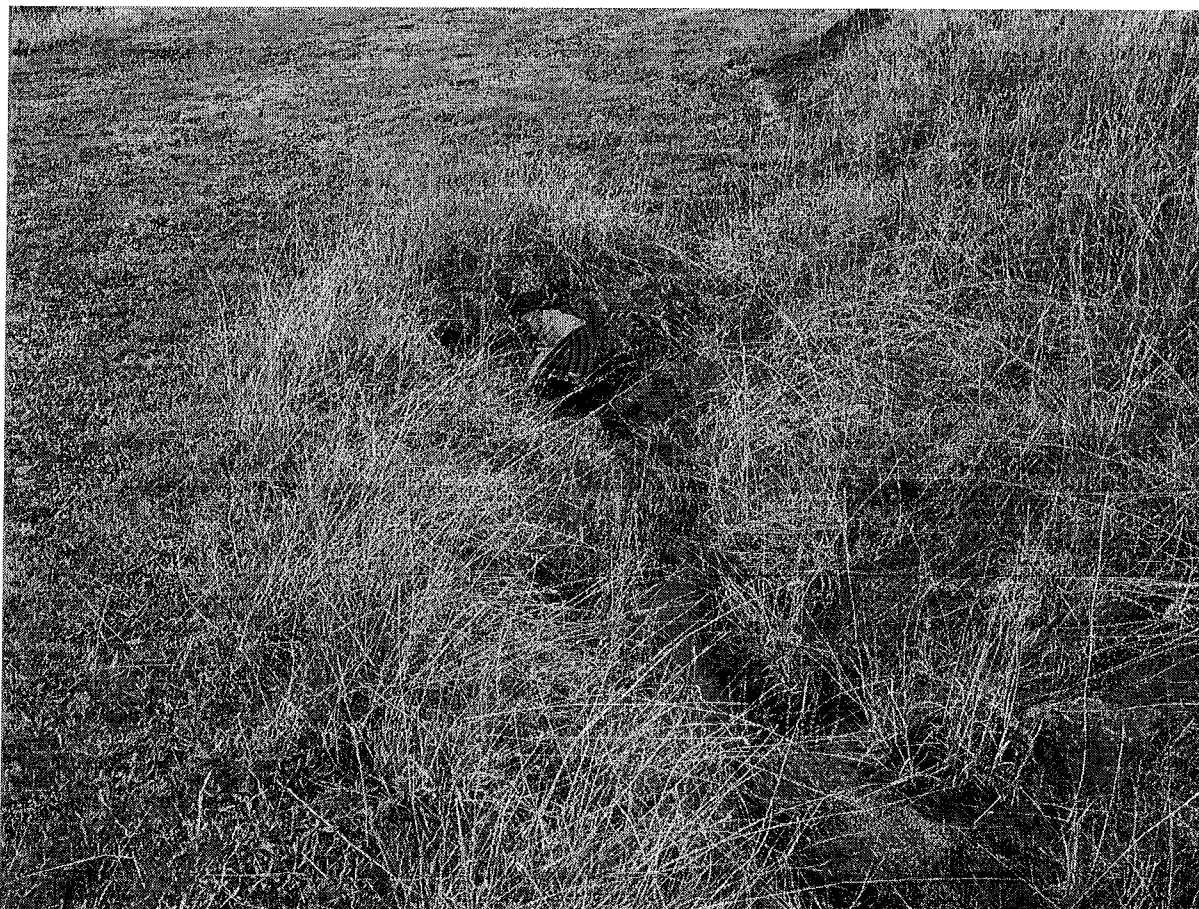
—Photograph #25— At Stream Crossing #11 view downstream; culvert inlet
