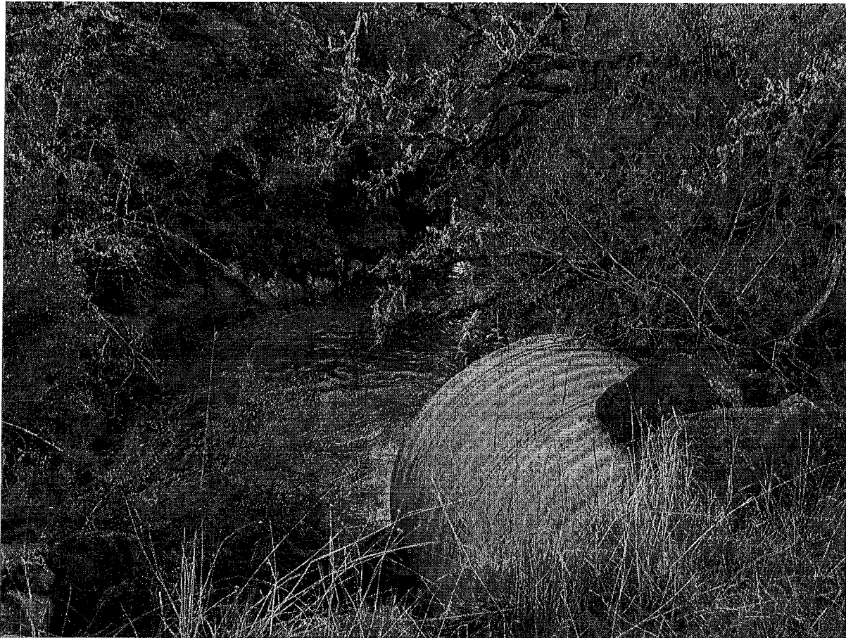
Photograph #21 – At Stream Crossing #10 view downstream
