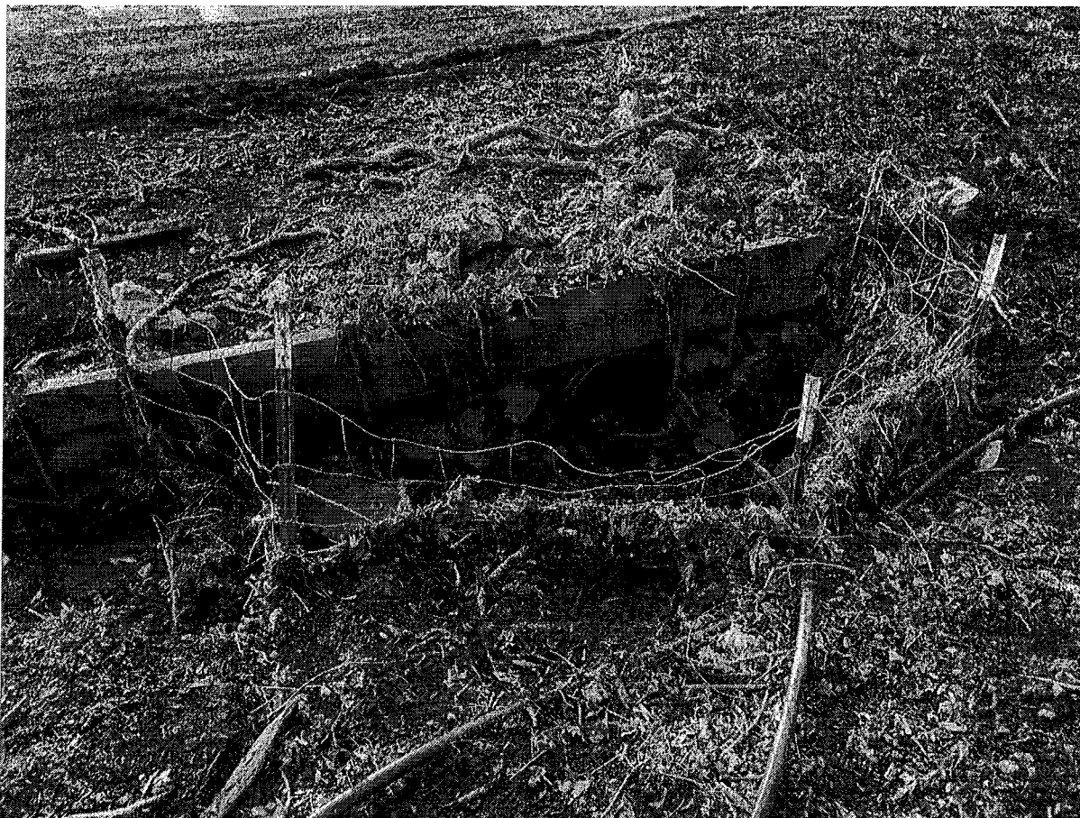
Photograph #18 – At Stream Crossing #8 looking downstream at inlet of 18" PCC
