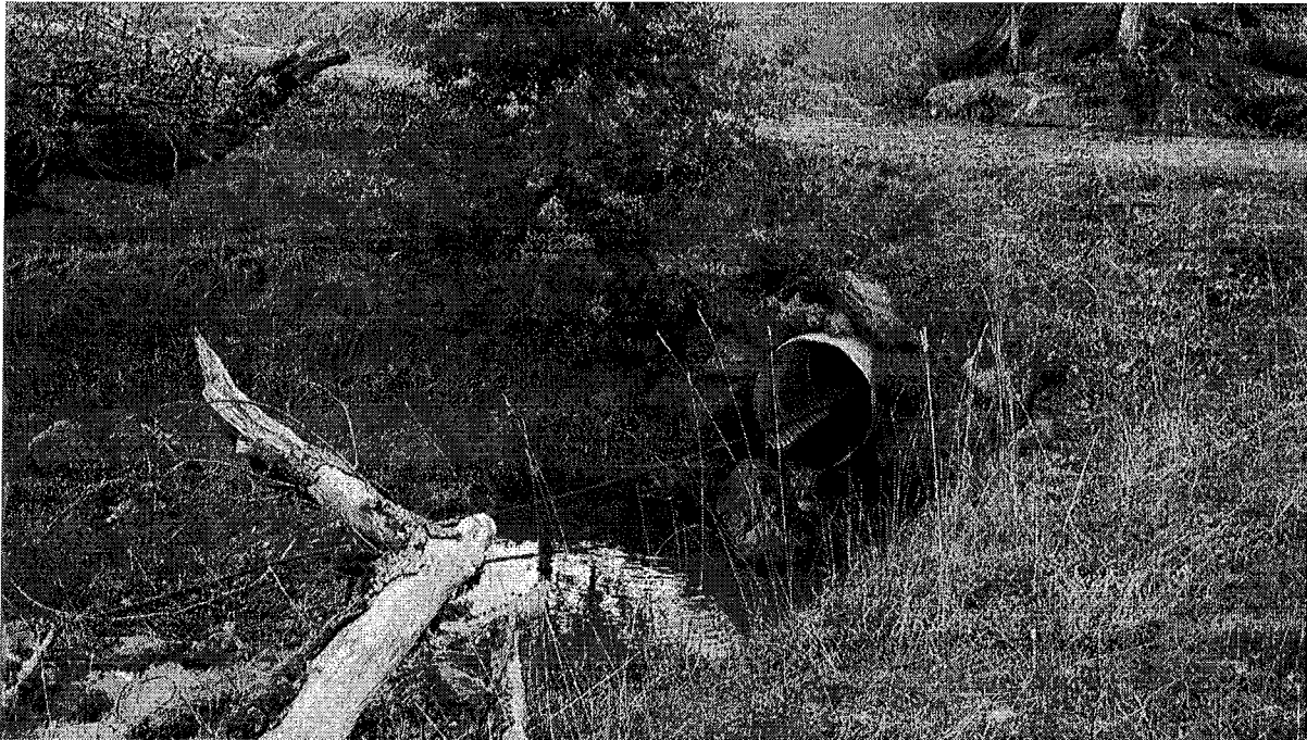
Photograph #5 – View of Stream Crossing #3 looking upstream
