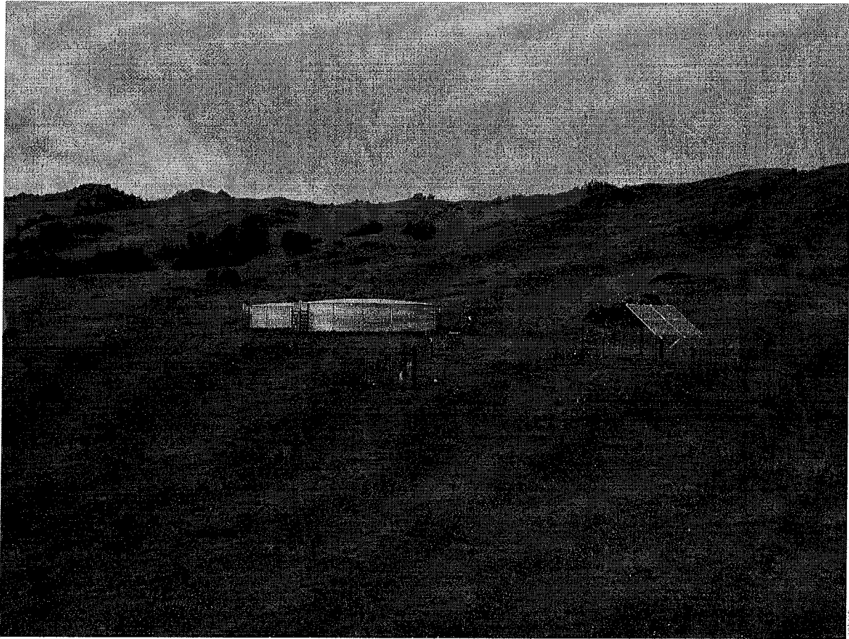
Photograph #37 – Additional water storage (2x 50,000-gallon tanks) and groundwater well in foreground.
