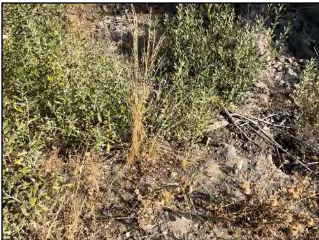
Photo #15 Unnamed Main Rd Looking @ Clogged 18" Culvert In
