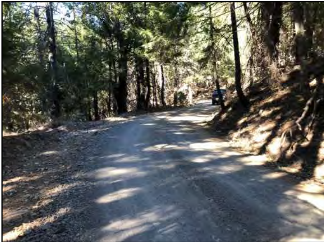
Photo #87 Unnamed Main Rd @ Pullout Looking NE @ Curve
