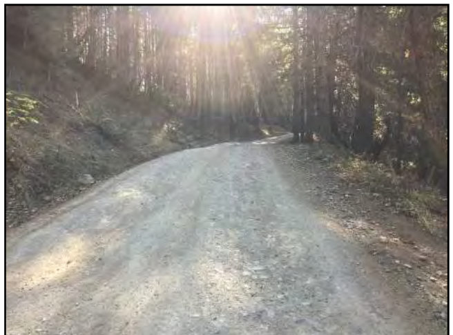
Photo #66 Unnamed Main Rd @ Pullout Looking SW @ Curve
