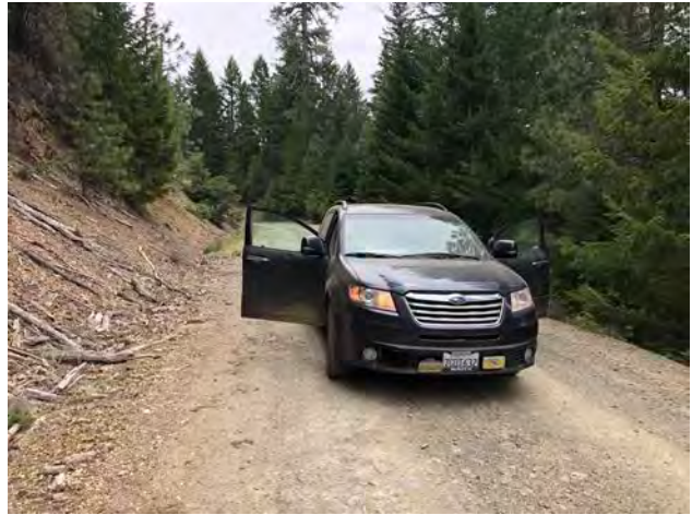
Photo #92 Access Road Looking S @ Unstable Hill
