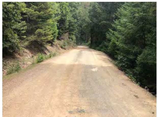
Photo #78 Access Road Looking E
