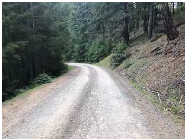
Photo #120 Access Road @ Curve Looking E
