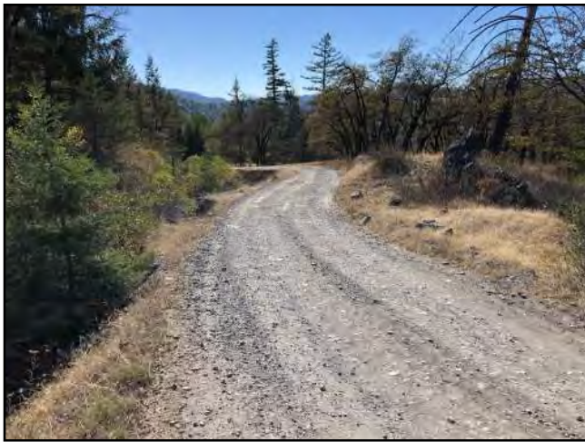
Photo #13 Unnamed Main Rd @ Pullout Looking SW @ Curve
