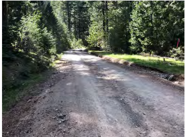
Photo #224 Access Road @ Curve Looking W
