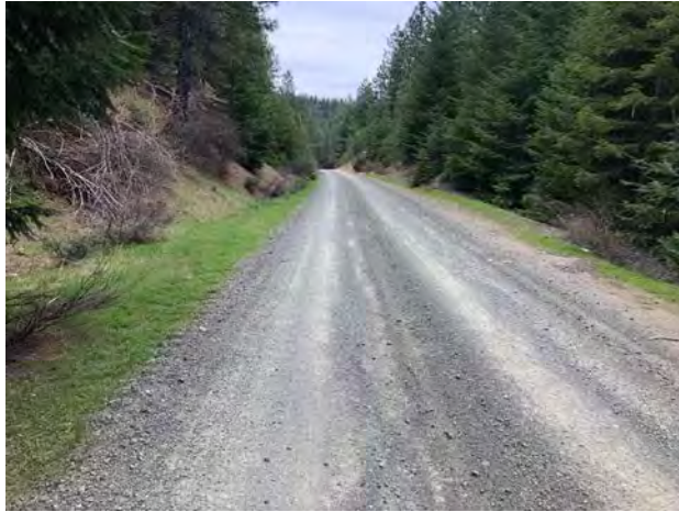
Photo #105 Access Road Looking South
