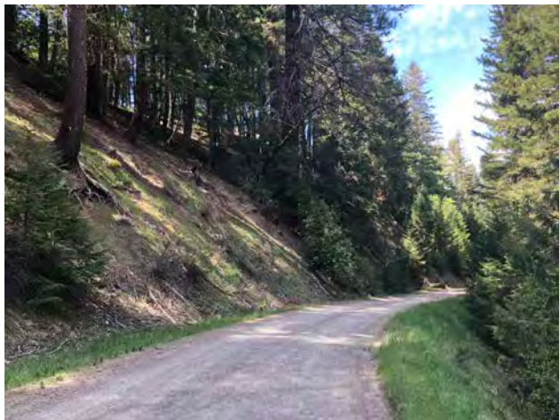
Photo #239 Access Road @ Curve Looking N
