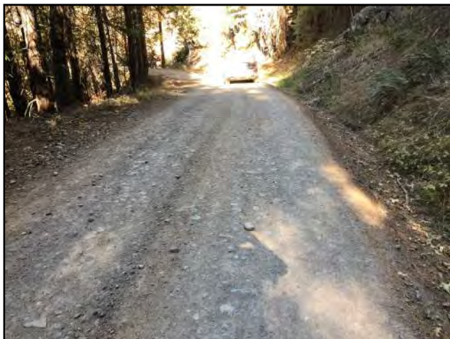
Photo #65 Unnamed Main Rd @ Pullout Looking NE @ Curve
