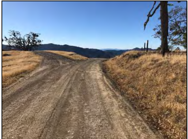
Photo #112 Unnamed Main Rd @ Driveway Looking SW
