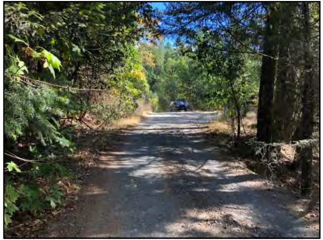
Photo # 449 Unnamed Main Rd @ Pullot Looking SE
