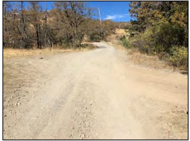
Photo #2 Unnamed Main Rd & Quad Trail w/ Turnaround Looking North @ Curve
