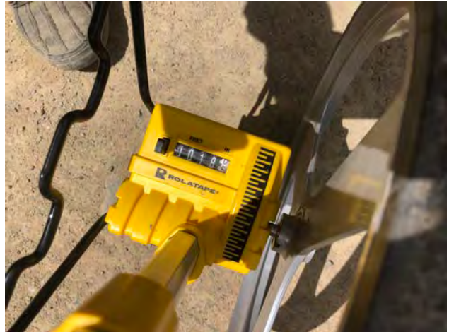
Photo #134 Access Road Width 18'
