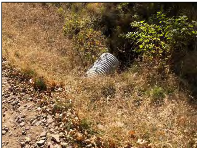
Photo #53 Unnamed Main Rd Looking @ 18" Culvert Out
