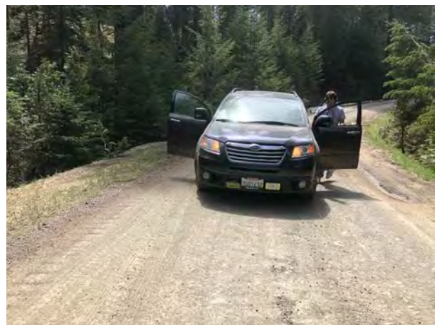
Photo #168 Access Road Looking SW
