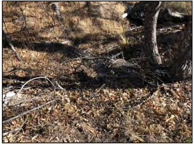
Photo #122 Unnamed Main Rd Clogged 18" Culvert In
