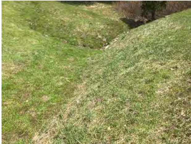
Photo #175 Access Road Looking @ Culvert In
