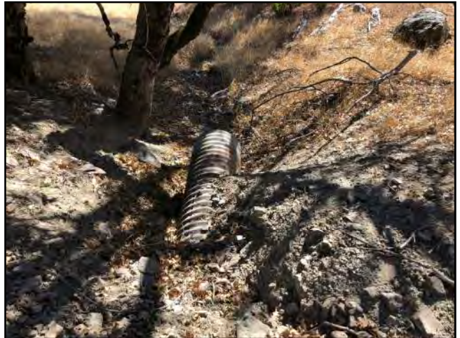
Photo #100 Unnamed Main Rd Looking @ 18" Culvert Out
