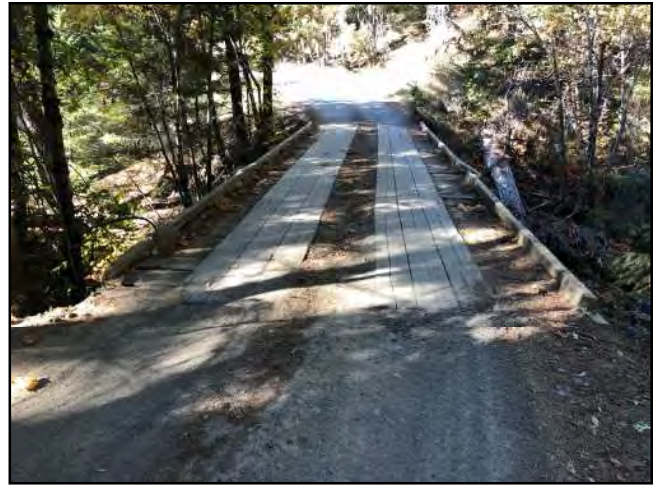
Photo #68 Unnamed Main Rd @ Railroad Car Bridge Looking SE
