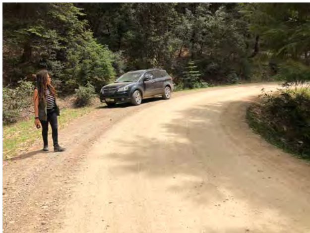
Photo #77 Access Road @ Curve Looking NE w/ Pullout
