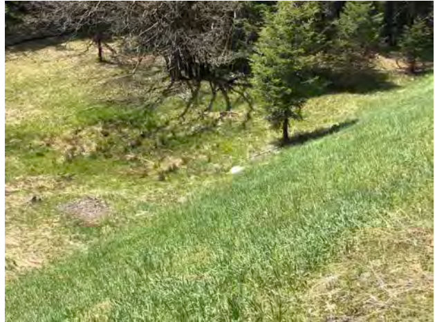
Photo #184 Access Road Looking @ Culvert In
