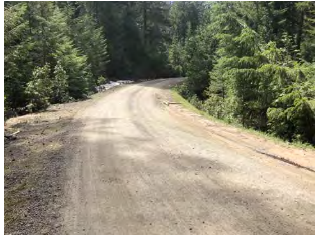
Photo #166 Access Road Looking SW @ Curve w/ Pullout
