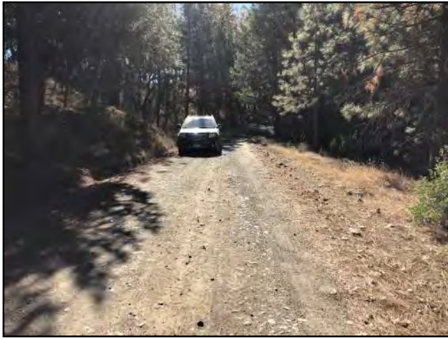
Photo #49 Unnamed Main Rd @ Pullout Looking SW @ Curve
