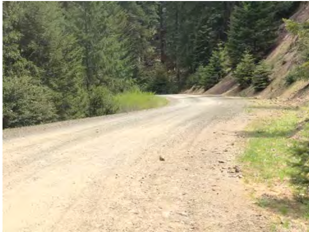
Photo #127 Access Road @ Curve Looking SE w/ Pullout
