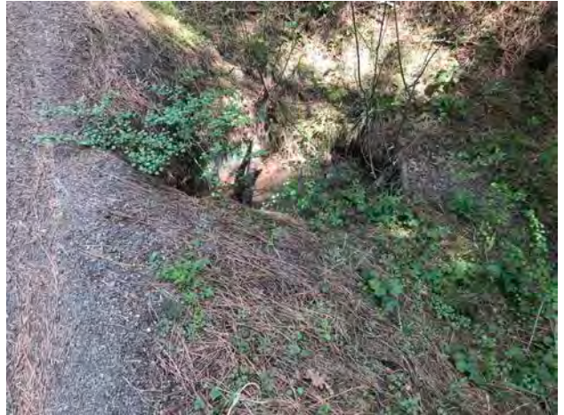
Photo #262 Access Road Looking @ Culvert Out
