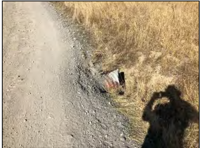
Photo #34 Unnamed Main Rd Looking @ 18" Culvert In
