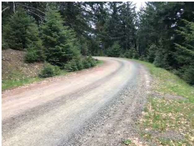
Photo #113 Access Road Looking SW @ Curve w/ Pullout
