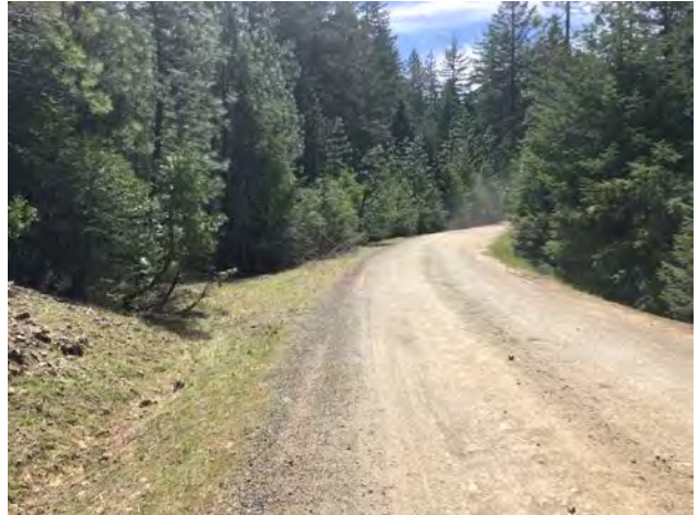
Photo #148 Access Road Looking SW @ Curve
