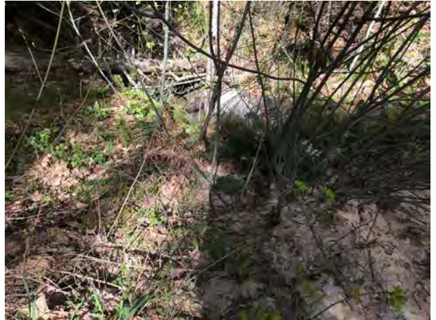
Photo #268 Access Road Looking @ Culvert Out
