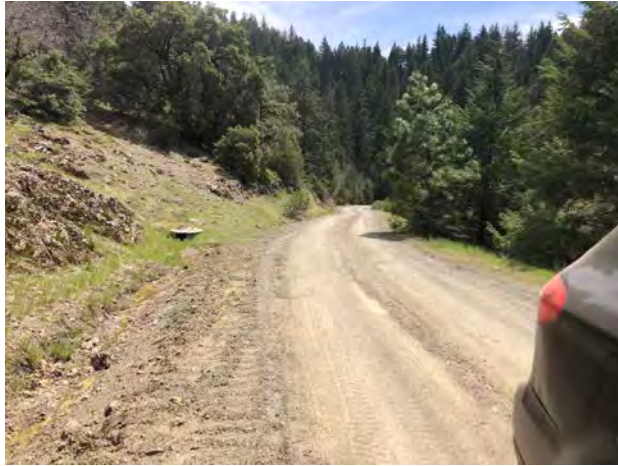
Photo #135 Access Road @ Curve Looking S w/ Pullout
