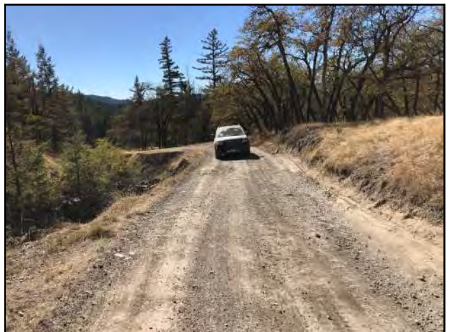
Photo #12 Unnamed Main Rd @ Pullout Looking South @ Curve
