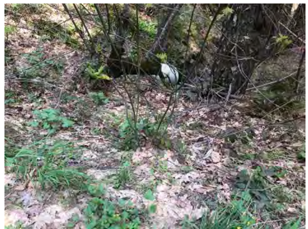
Photo #270 Access Road Looking @ Culvert Out
