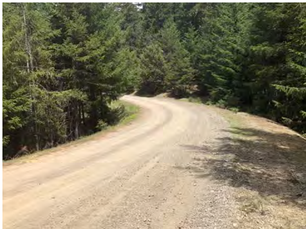
Photo #131 Access Road @ Curve Looking NE w/ Pullout
