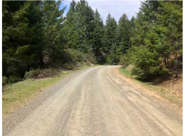
Photo #154 Access Road @ Curve Looking N
