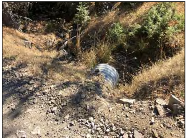
Photo #94 Unnamed Main Rd Looking @ 18" Culvert Out
