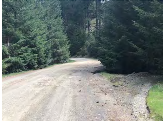
Photo #196 Access Road @ Curve Looking SE w/ Pullout
