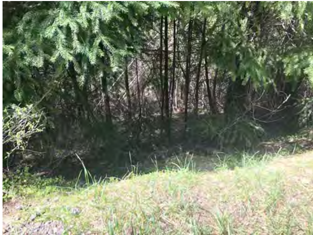
Photo #211 Access Road Looking @ Culvert Out
