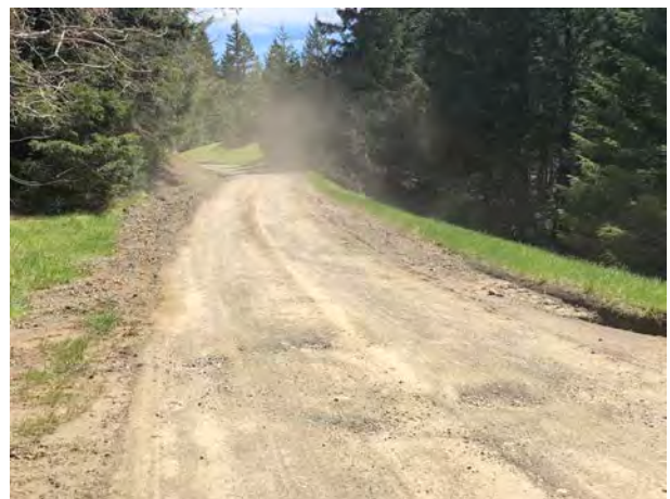
Photo #180 Access Road Looking SE @ Curve
