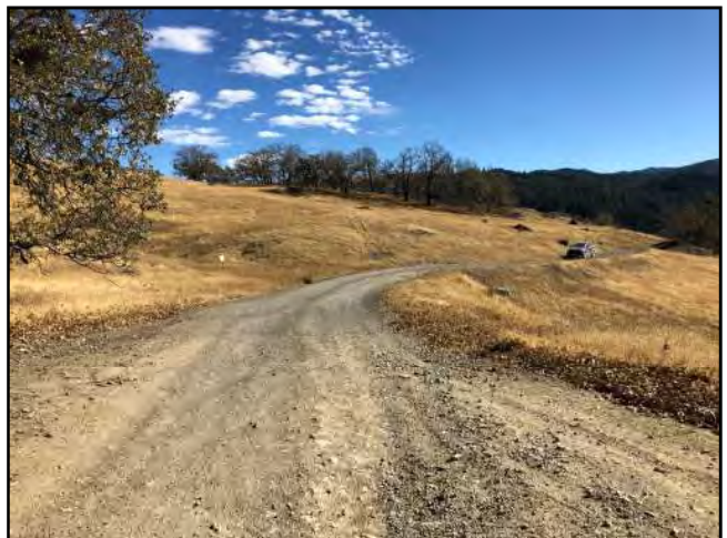
Photo #36 Unnamed Main Rd @ Intersection of Private Access Rd Looking SE @ Curve
