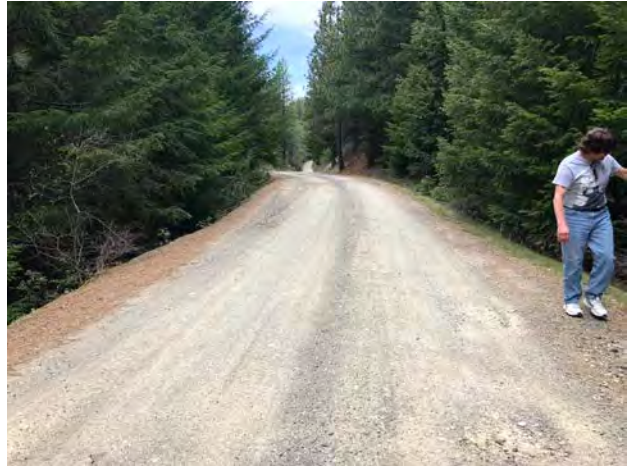
Photo #94 Access Road Looking NW @ Curve
