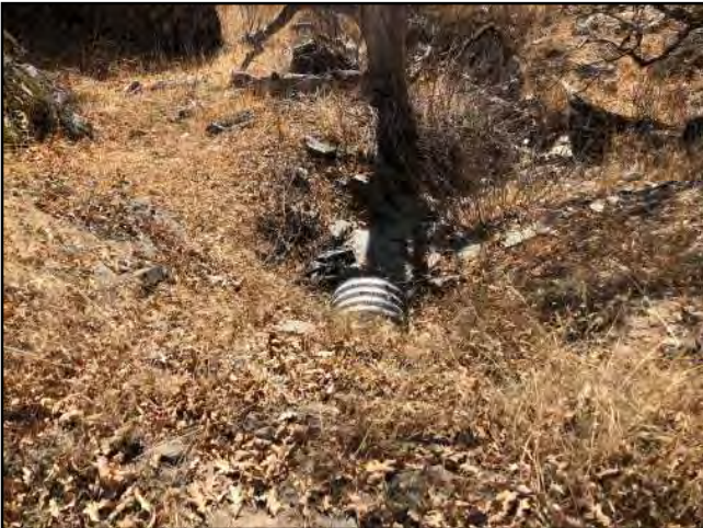
Photo #27 Unnamed Main Rd Looking @ 18" Culvert Out
