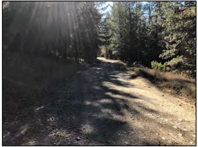
Photo #50 Unnamed Main Rd @ Curve w/ Pullout Looking SW
