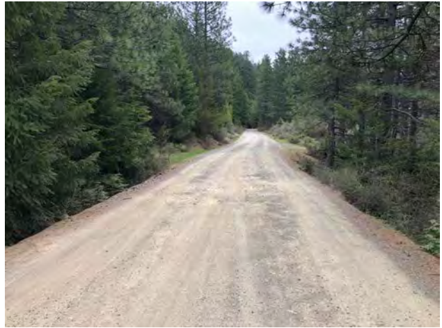
Photo #98 Access Road Looking SE
