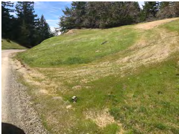
Photo #173 Access Road Looking NW @ Driveway
