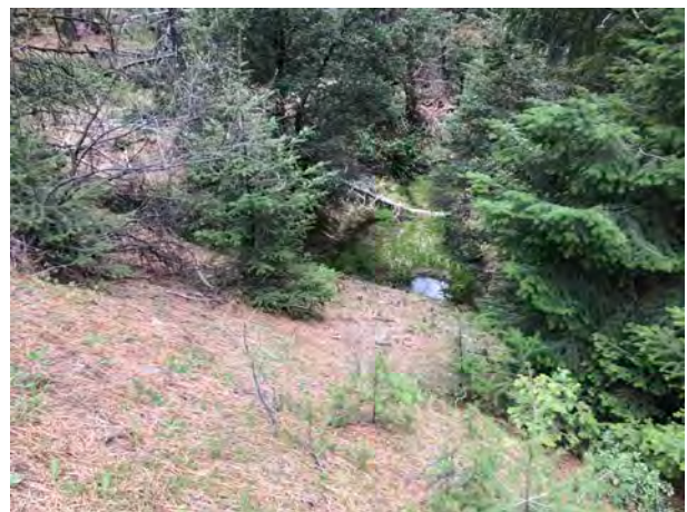
Photo #96 Access Road Looking @ Culvert In
