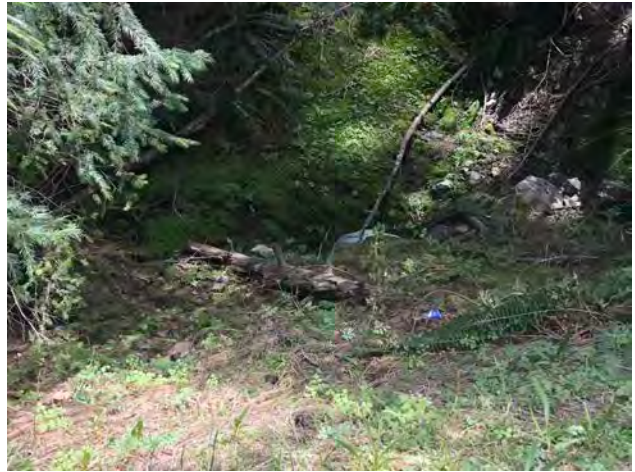
Photo #194 Access Road Looking @ Culvert In
