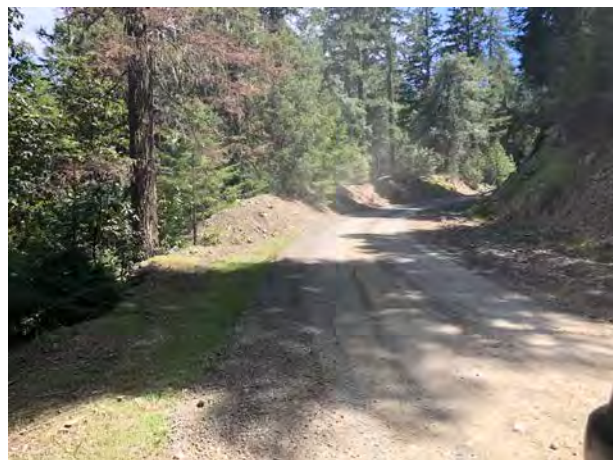
Photo #228 Access Road @ Curve Looking S w/ Pullout
