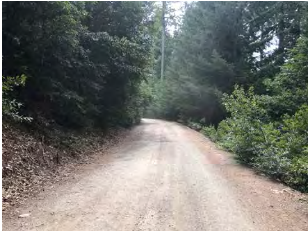
Photo #85 Access Road @ Curve Looking SW
