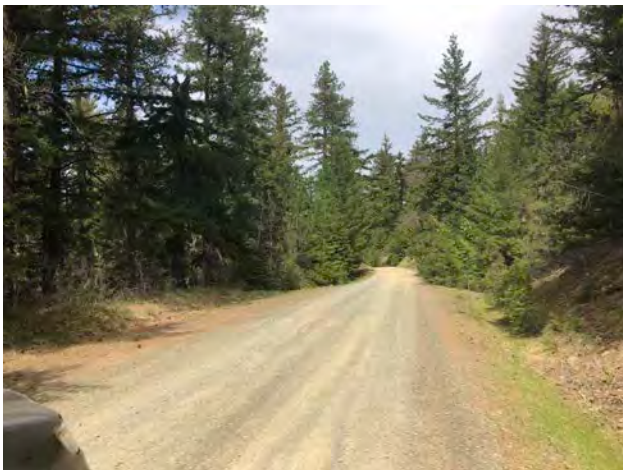
Photo #149 Access Road Looking NE @ Curve w/ Pullout
