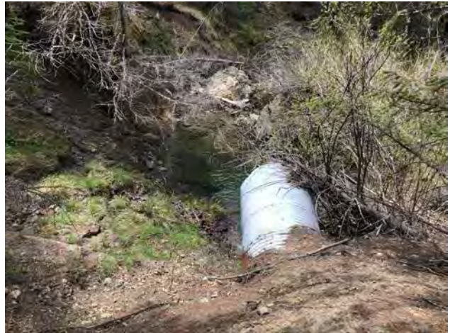
Photo #68 Access Road Looking @ Culvert Out
