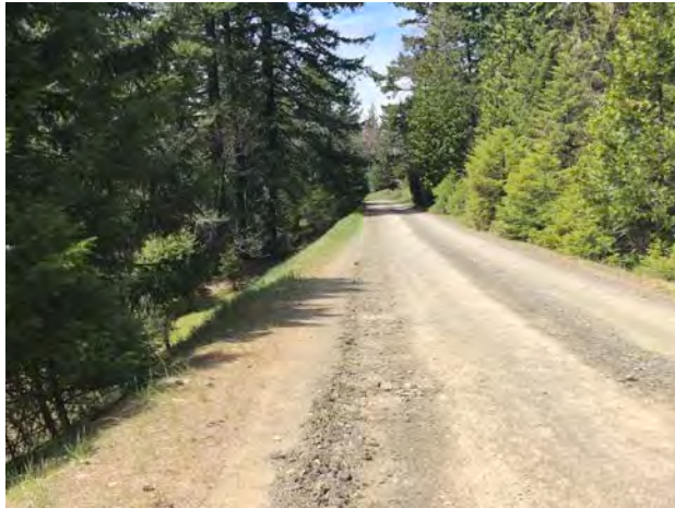
Photo #181 Access Road looking NW w/ Pullout
