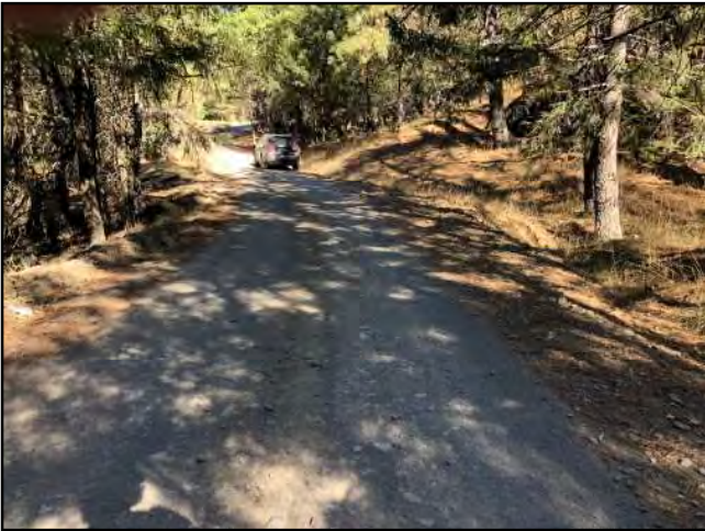
Photo #45 Unnamed Main Rd @ Pullout Looking NE @ Curve
