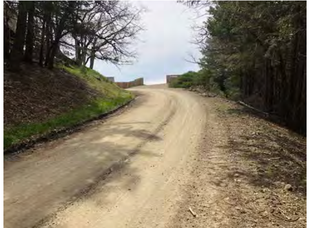
Photo #58 Access Road Looking SW @ Curve w/ Pullout
