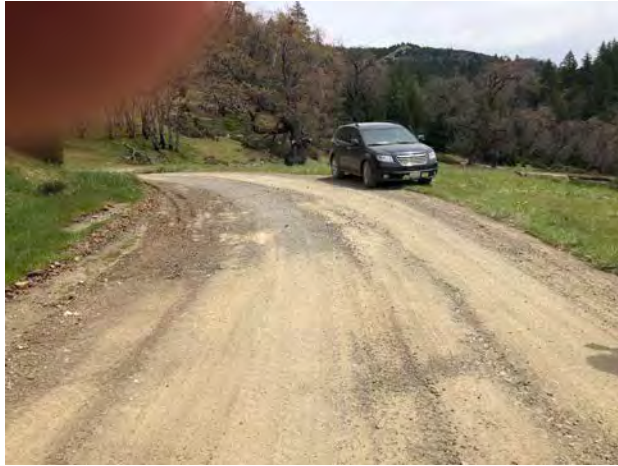
Photo #57 Access Road @ Curve Looking SE w/ Pullout
