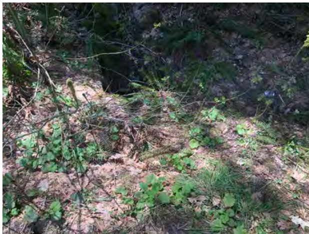
Photo #269 Access Road Looking @ Culvert In
