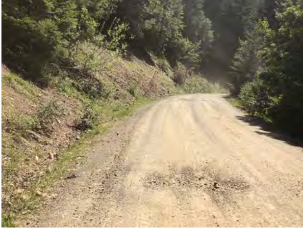
Photo #279 Access Road @ Curve Looking SW
