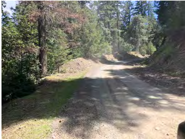
Photo #229 Access Road @ Curve Looking NE w/ Pullout
