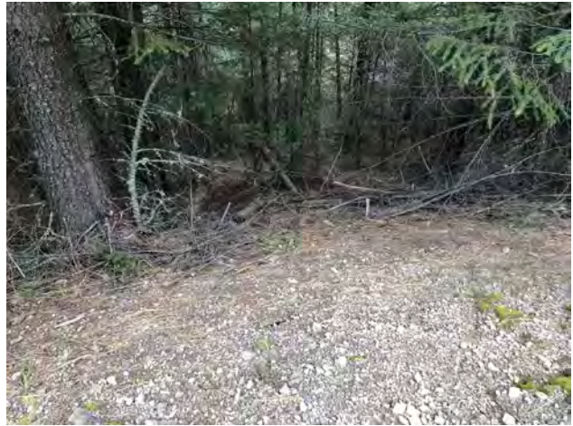
Photo #104 Access Road Looking @ Culvert Out
