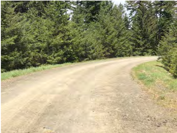
Photo #187 Access Road Looking NE @ Curve w/ Pullout
