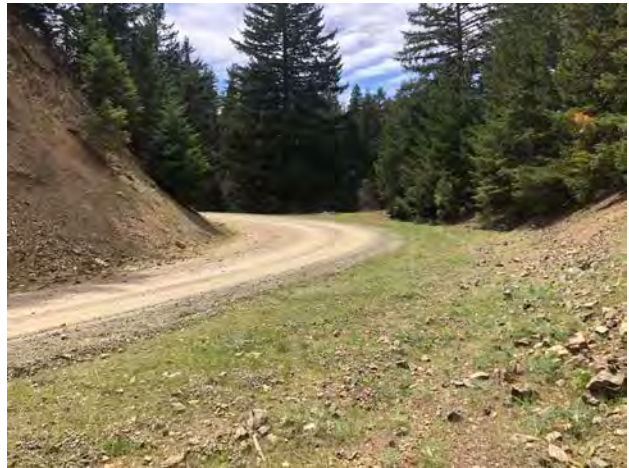
Photo #130 Access Road @ Curve Looking SW w/ Pullout
