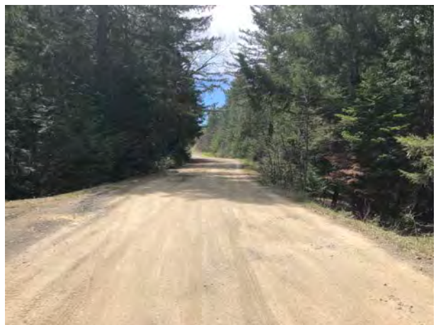
Photo #144 Access Road Looking SW
