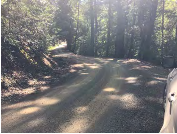
Photo #277 Access Road @ Curve Looking SW w/ Pullout
