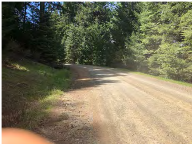
Photo #215 Access Road @ Curve Looking NW w/ Pullout
