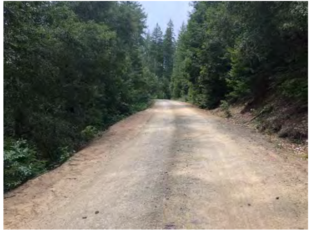
Photo #80 Access Road Looking W
