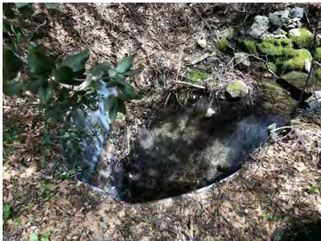
Photo #71 Access Road Looking at Culvert In
