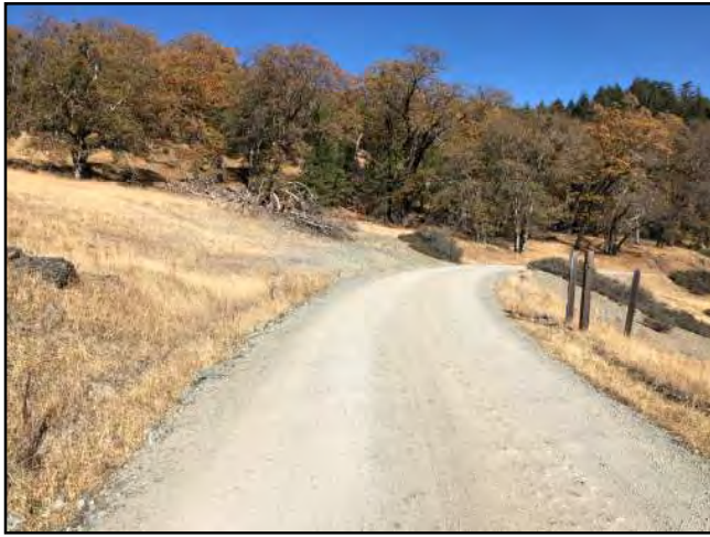
Photo #103 Unnamed Main Rd @ Pullout Looking NE @ Curve
