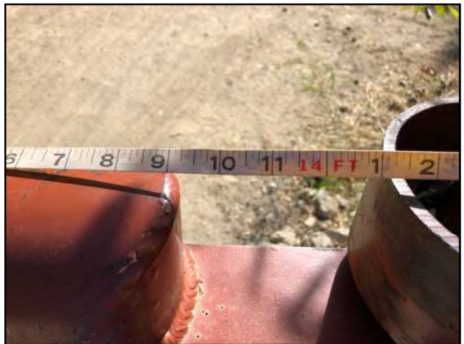
Photo #457 Unnamed Main Road Gate Width 14' (See Photo 461)
