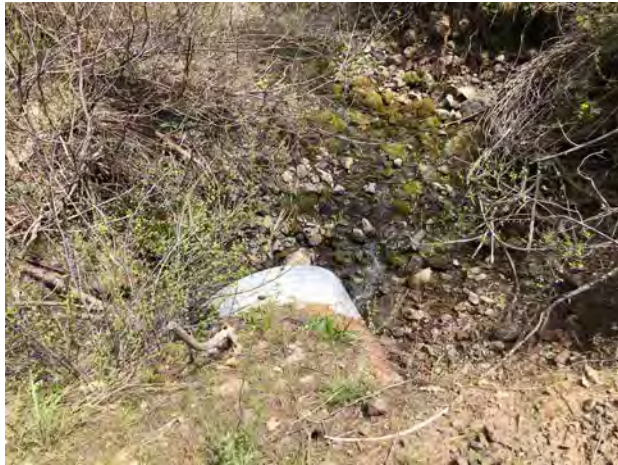
Photo #67 Access Road Looking @ Culvert In
