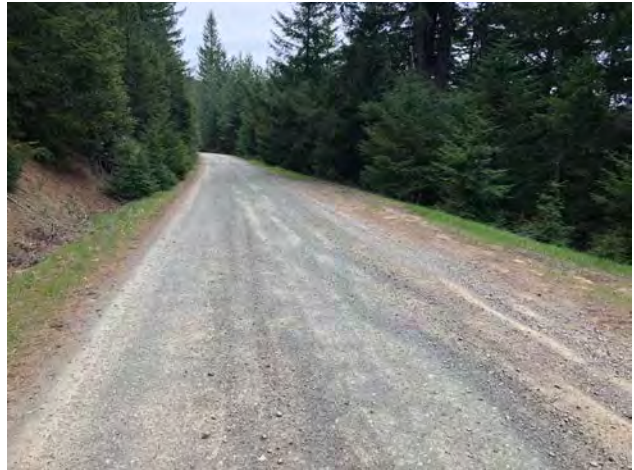
Photo #110 Access Road Looking SE w/ Pullout
