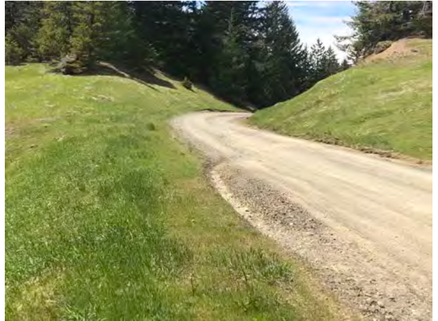
Photo #178 Access Road Looking NW @ Curve w/ Pullout
