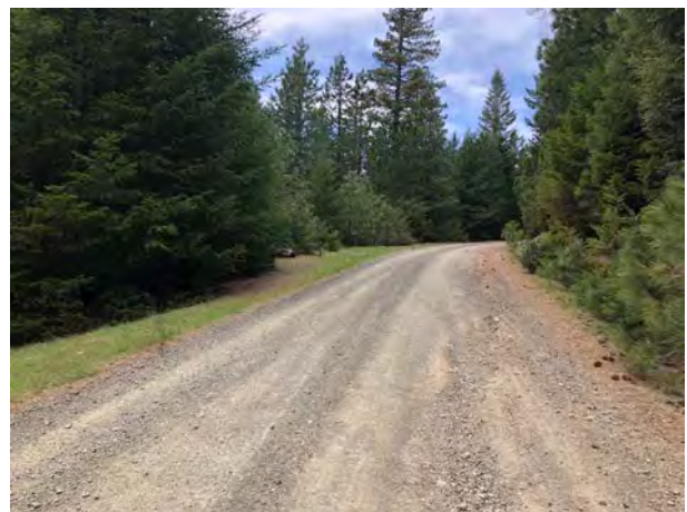
Photo #108 Access Road @ Curve Looking W
