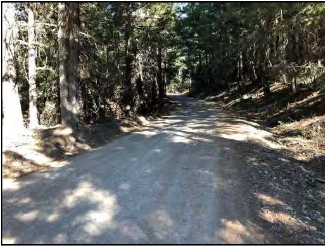
Photo #73 Unnamed Main Rd @ Pullout Looking SW @ Curve
