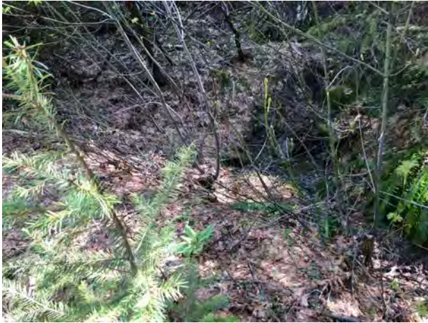
Photo #249 Access Road Looking @ Culvert In
