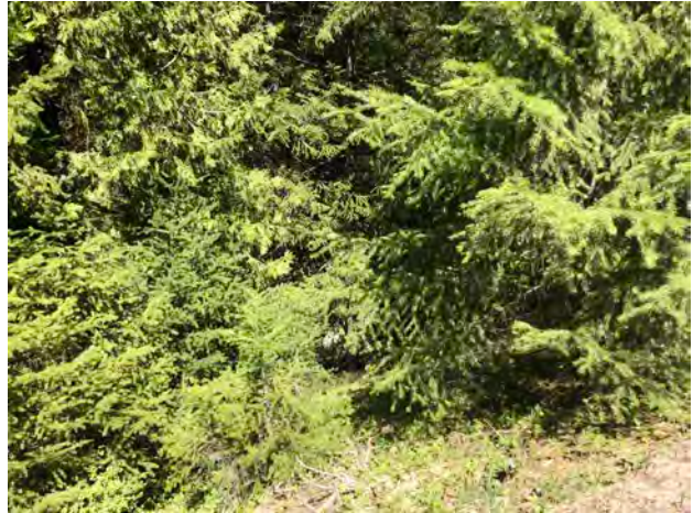
Photo #238 Access Road Looking at Culvert Out
