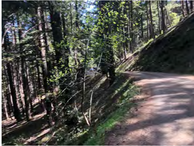
Photo #273 Access Road @ Curve Looking SW w/out Pullout
