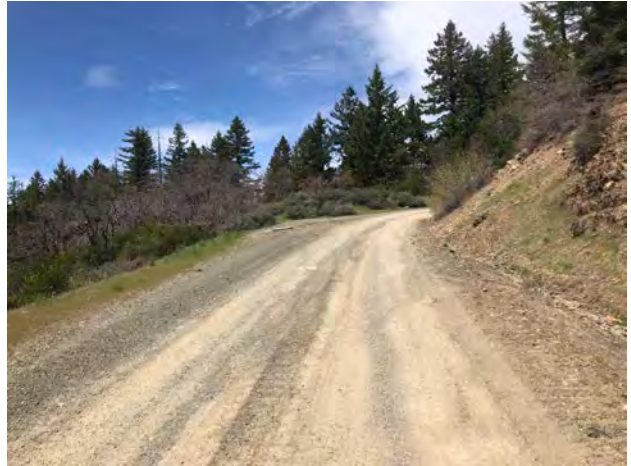
Photo #136 Access Road @ Curve Looking N
