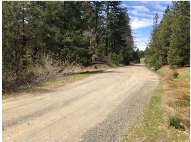
Photo #170 Access Road Looking N @ Curve
