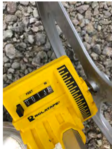
Photo #66 Access Road Width 13.6'
