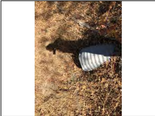
Photo #99 Unnamed Main Rd Looking @ 18" Culvert In
