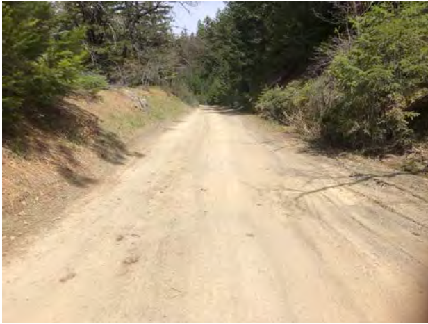
Photo #147 Access Road Looking NE @ Curve
