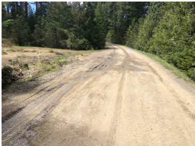
Photo #161 Access Road @ Curve Looking SW
