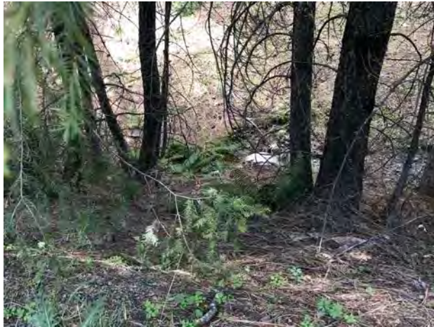
Photo #199 Access Road Looking @ Culvert In
