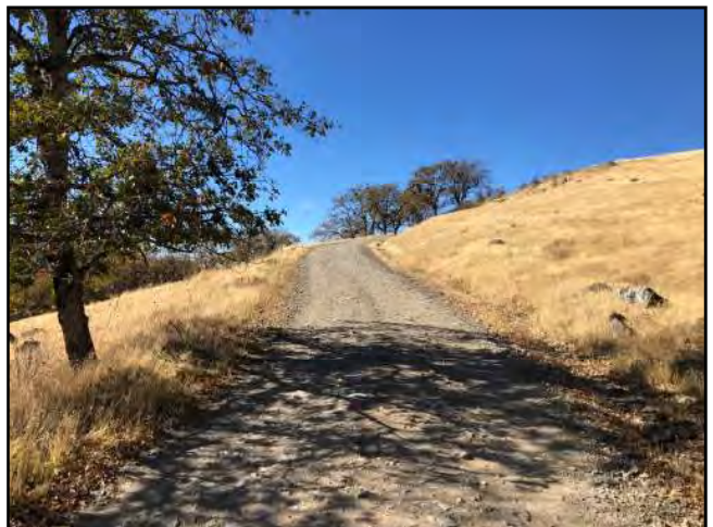
Photo #24 Unnamed Main Rd @ Curve w/ Pull-out Looking NW
