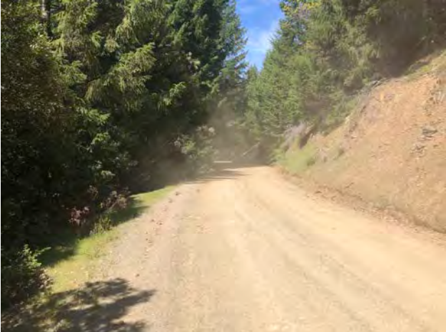
Photo #278 Access Road Looking NE @ Curve
