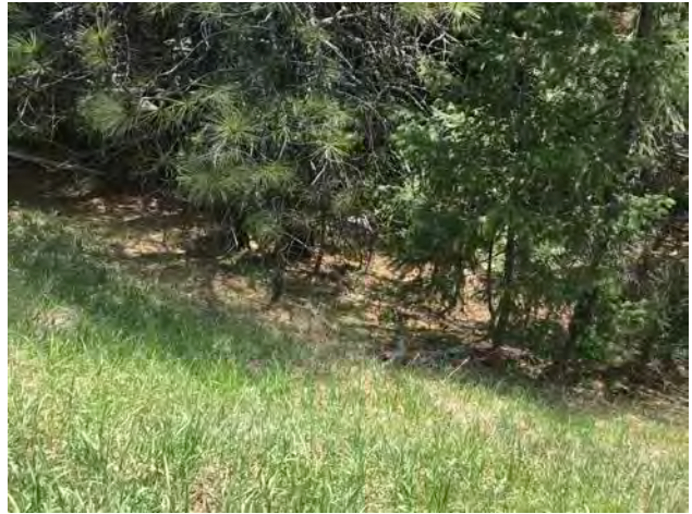
Photo #176 Access Road Looking @ Culvert Out
