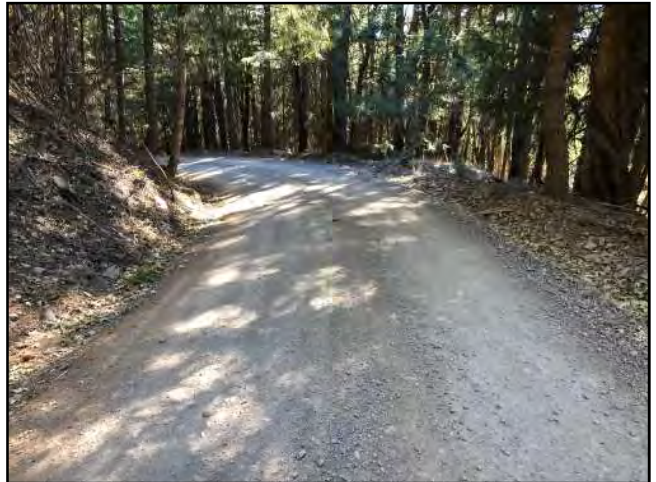
Photo #88 Unnamed Main Rd @ Pullout Looking SW @ Curve
