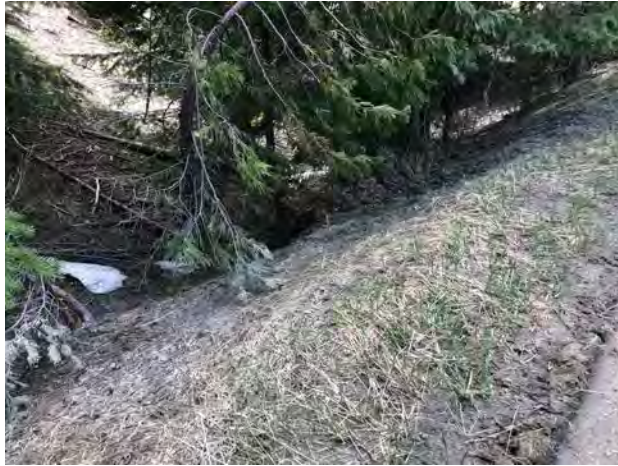
Photo #159 Access Road Looking @ Culvert In
