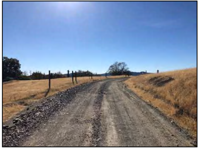
Photo #104 Unnamed Main Rd @ Pullout Looking SW @ Curve
