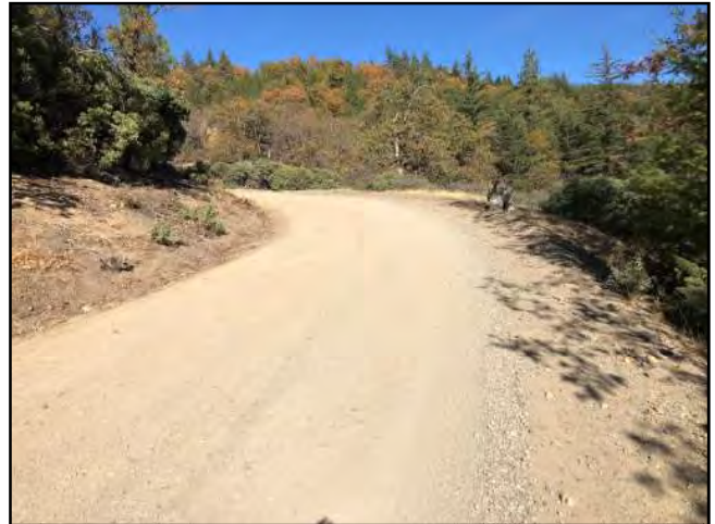
Photo #118 Unnamed Main Rd @ Pullout Looking NE @ Curve
