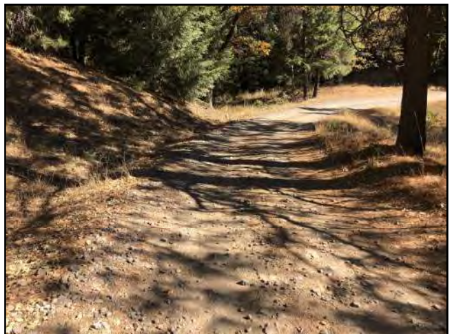
Photo #54 Unnamed Main Rd @ Pullout Looking NE @ Curve
