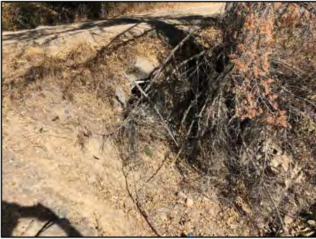
Photo #7 Unnamed Main Rd Looking @ 18" Culvert Out (Culvert In Photo 6)
