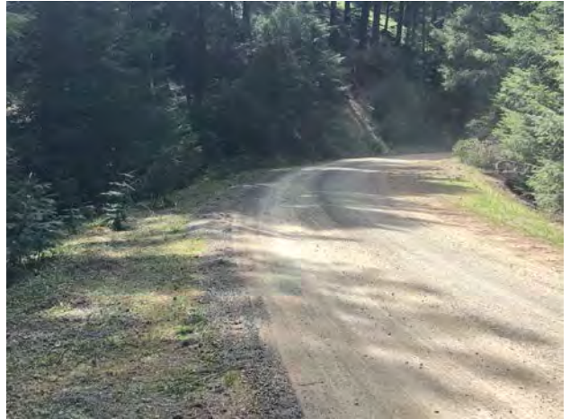
Photo #202 Access Road @ Curve Looking SW w/ Pullout
