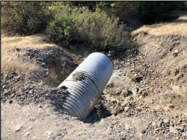
Photo #9 Unnamed Main Rd Looking @ 18" Culvert Out (Culvert In Photo 8)
