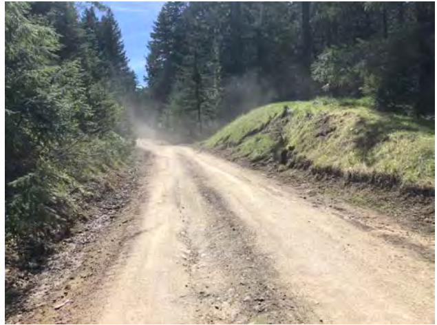
Photo #206 Access Road Looking SW
