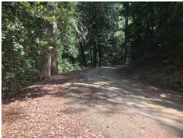
Photo #275 Access Road @ Curve Looking SE w/ Pullout
