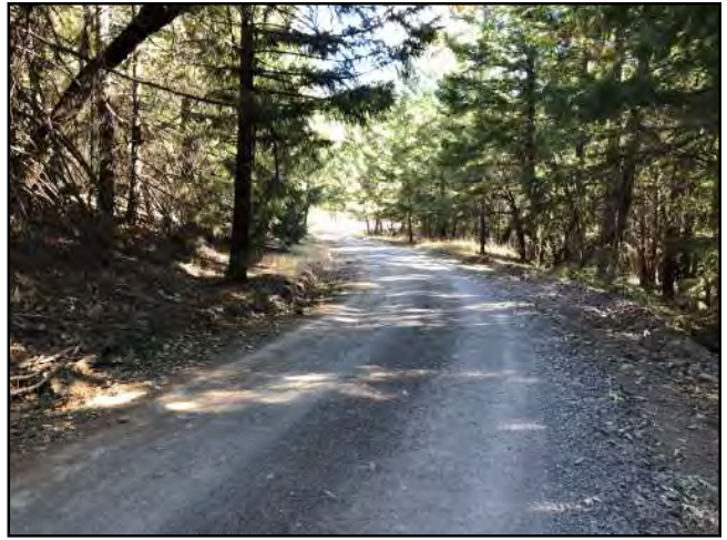
Photo #86 Unnamed Main Rd @ Pullout Looking SW @ Curve
