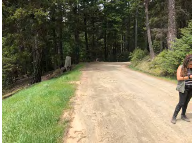
Photo #70 Access Road @ Curve Looking NW w/ Pullout
