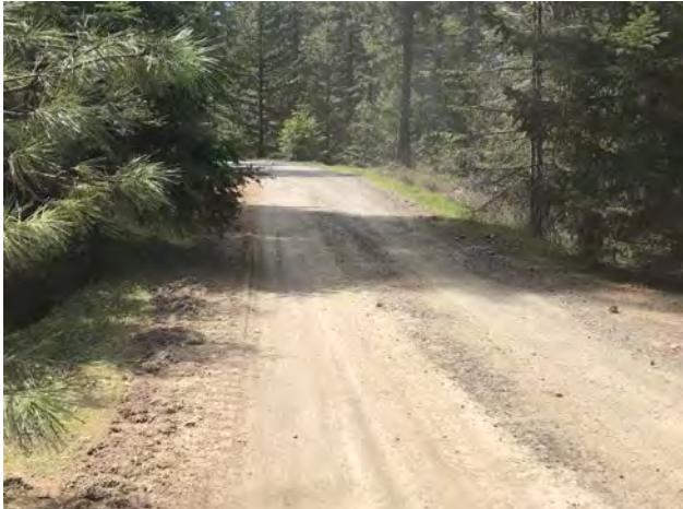
Photo #191 Access Road Looking W
