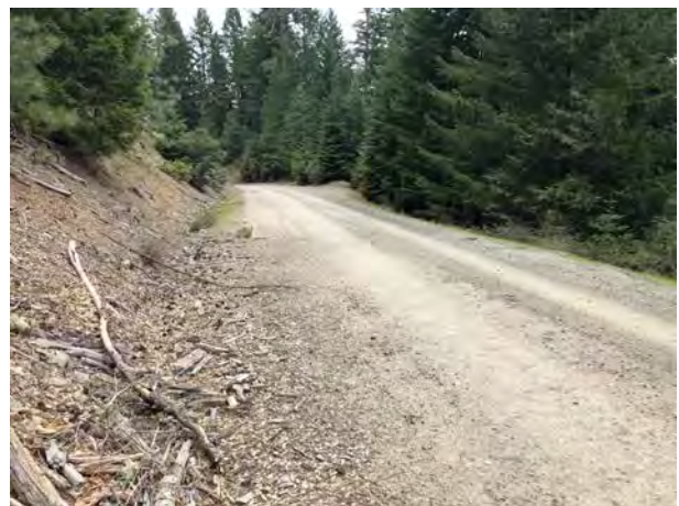
Photo #90 Access Road Looking SE w/ Pullout
