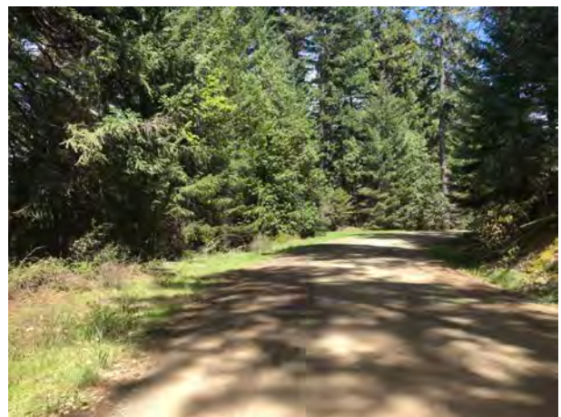
Photo #264 Access Road @ Curve Looking E
