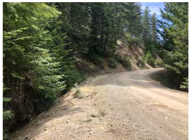
Photo #132 Access Road @ Curve w/ Culvert In
