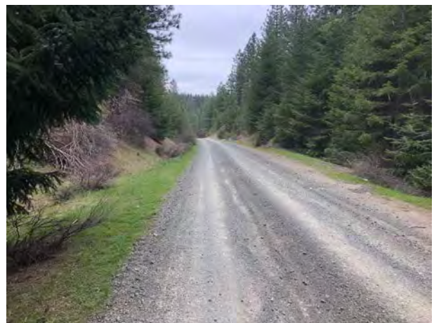
Photo #102 Access Road @ Curve Looking SE w/ Pullout
