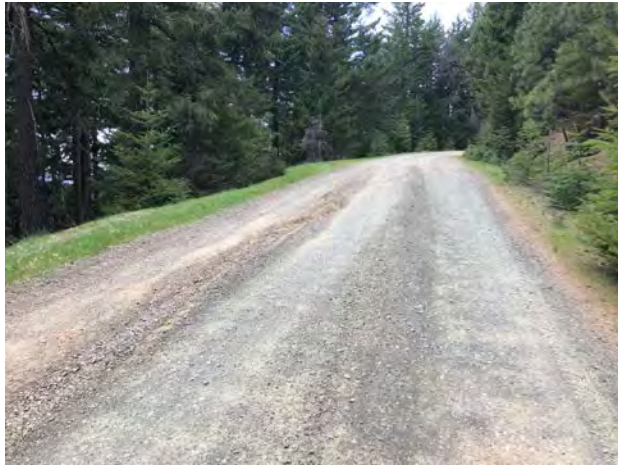
Photo #109 Access Road @ Curve Looking NW w/ Pullout
