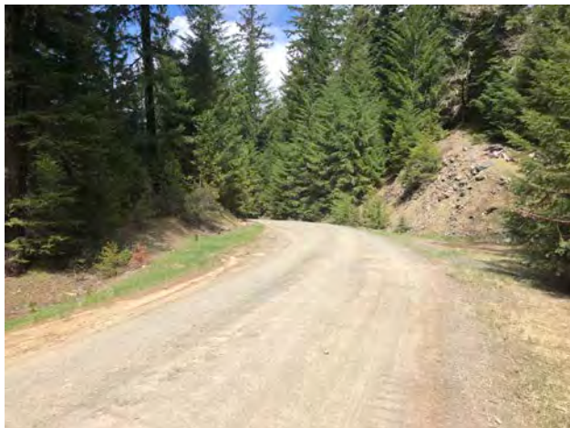
Photo #167 Access Road Looking at NE @ Curve w/ Pullout
