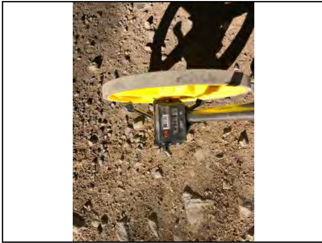
Photo #67 Unnamed Main Rd Width 13'9"
