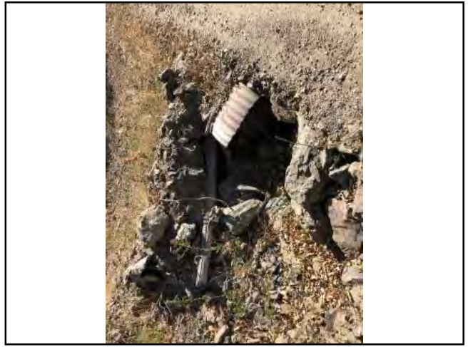
Photo #8 Unnamed Main Rd Looking @ 18" Culvert In
