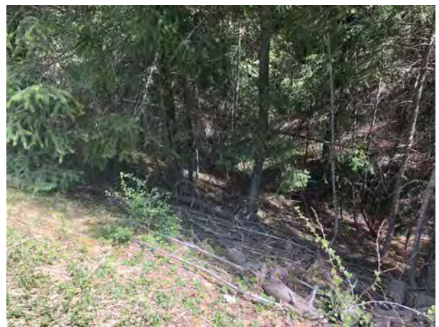
Photo #210 Access Road Looking @ Culvert In
