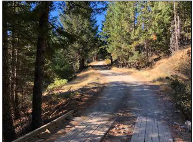
Photo #70 Unnamed Main Rd @ Railroad Car Bridge Looking NW
