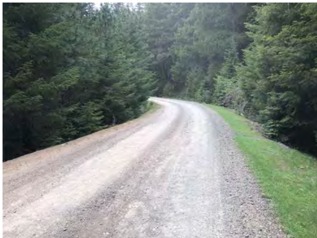
Photo #101 Access Road @ Curve Looking NW w/ Pullout
