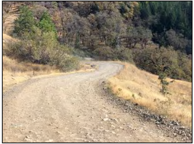
Photo #20 Unnamed Main Rd @ Pullout Looking South @ Curve
