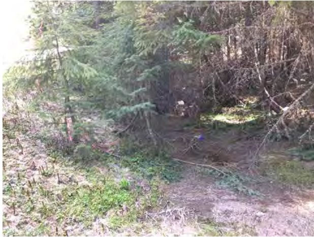
Photo #237 Access Road Looking @ Culvert In
