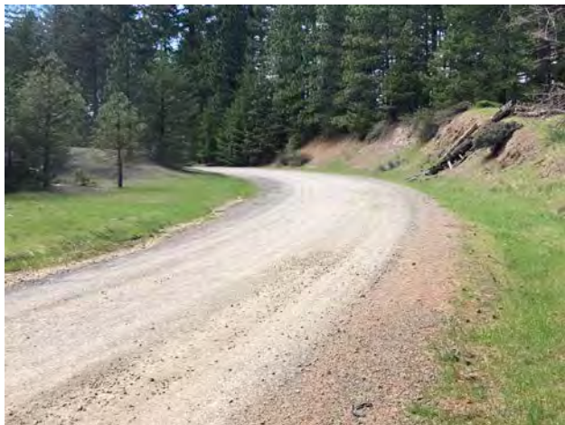
Photo #197 Access Road @ Curve Looking NW w/ Pullout
