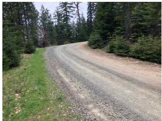
Photo #114 Access Road Looking NE @ Curve w/ Pullout
