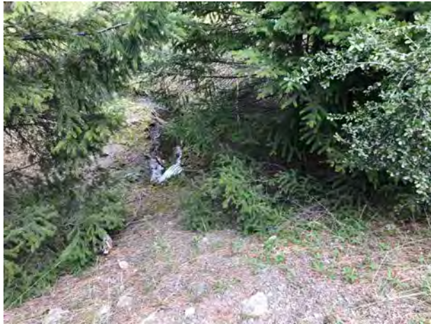
Photo #97 Access Road Looking @ Culvert Out
