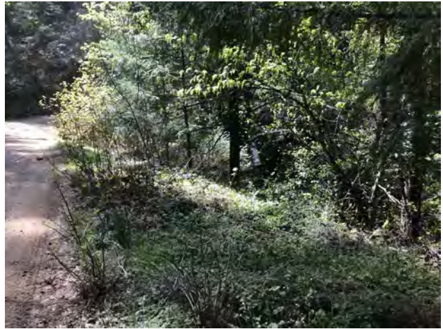
Photo #266 Access Road Looking @ Culvert Out
