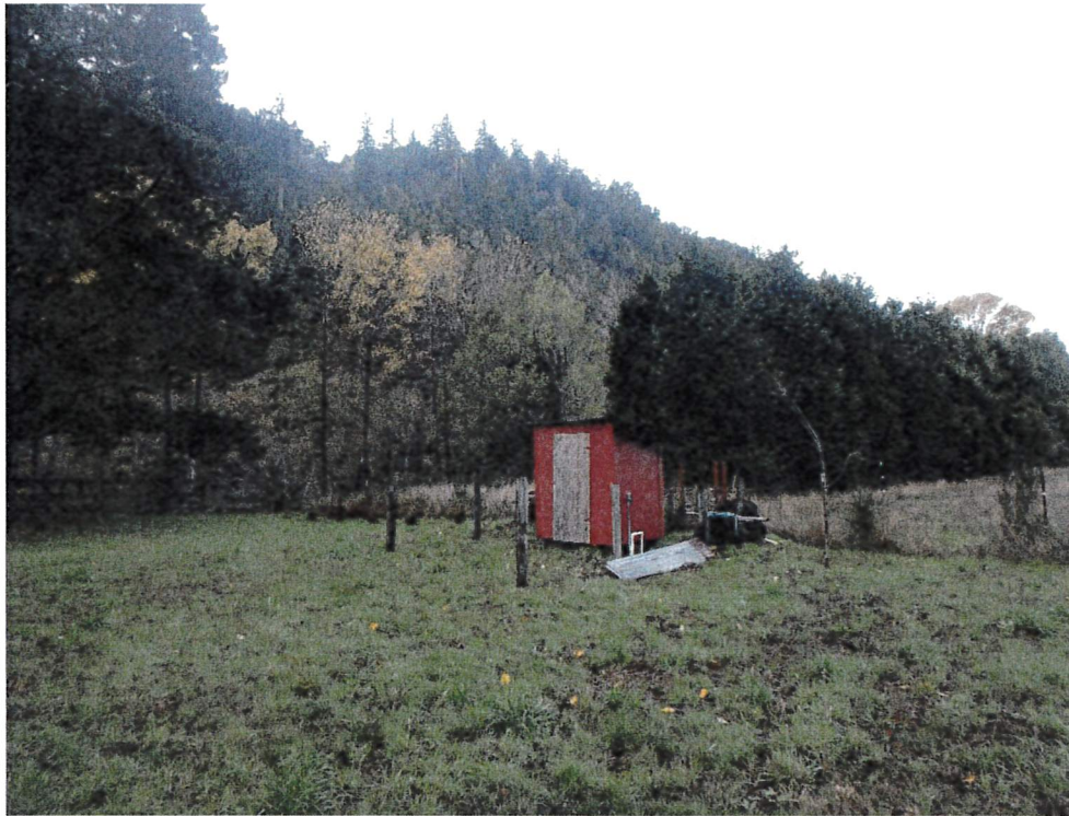
Photo 5; MP #2 – The well house on APN 105-111-017.
